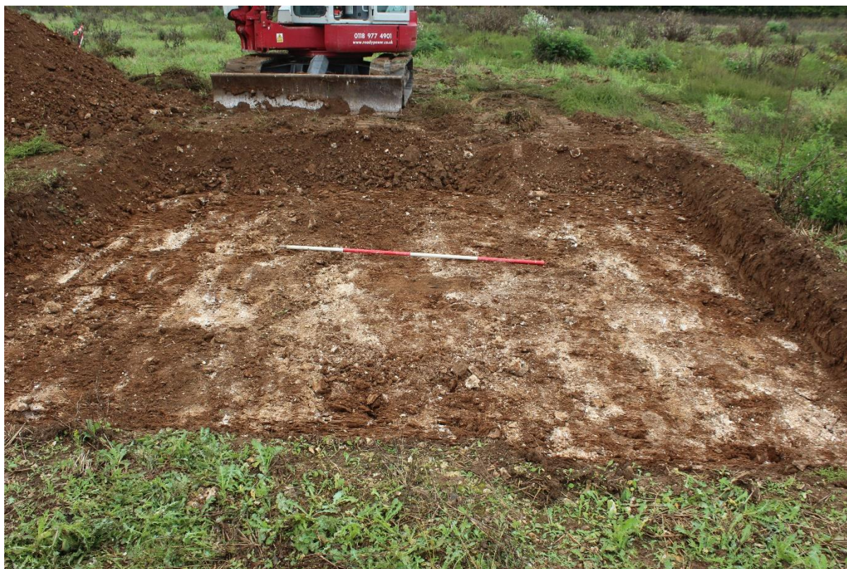
Plate 1 – Trench 41 Overview - Looking South
