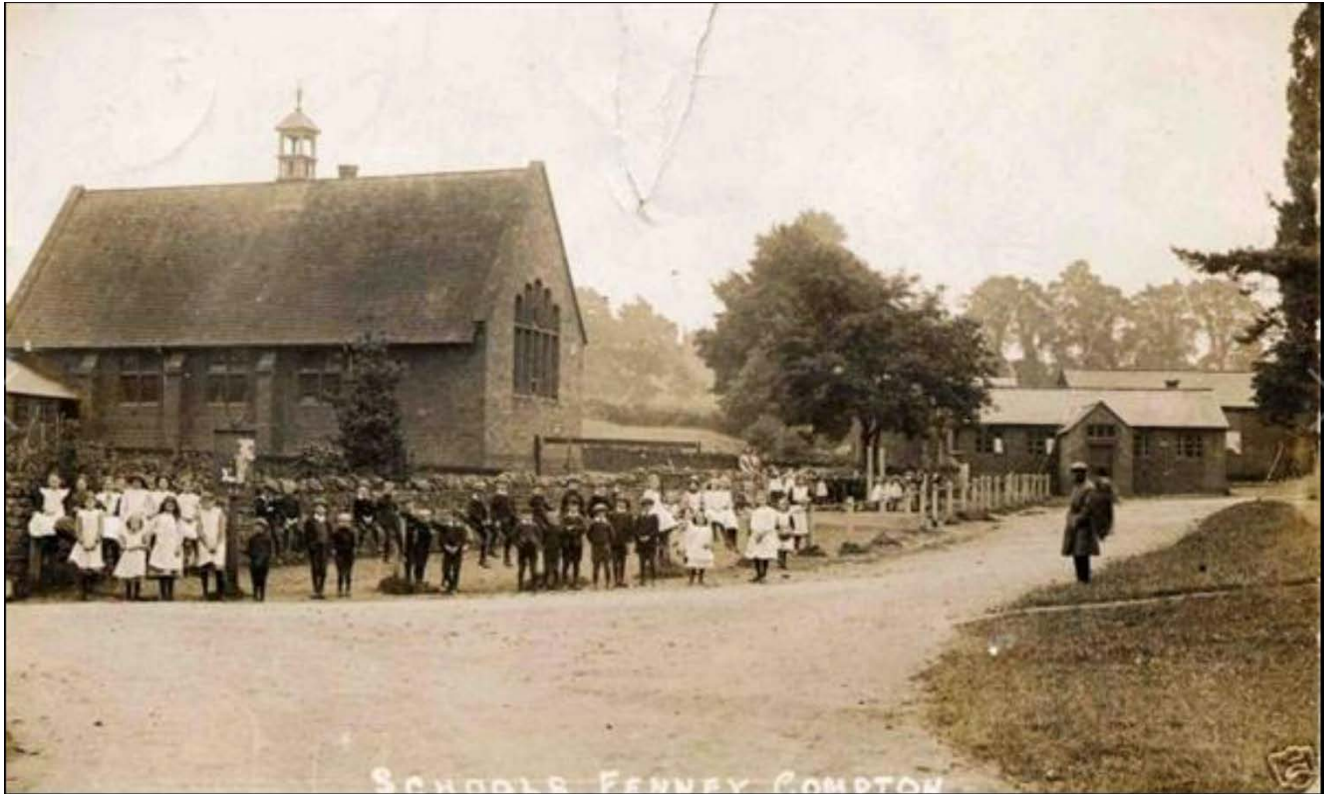
Historic Plate 1: Late 19 th /early 20 th century photograph of the 1890 Fenny Compton School (left), the former 1833 School (right) with Building B behind, looking east (viewpoint on Figure 2)
