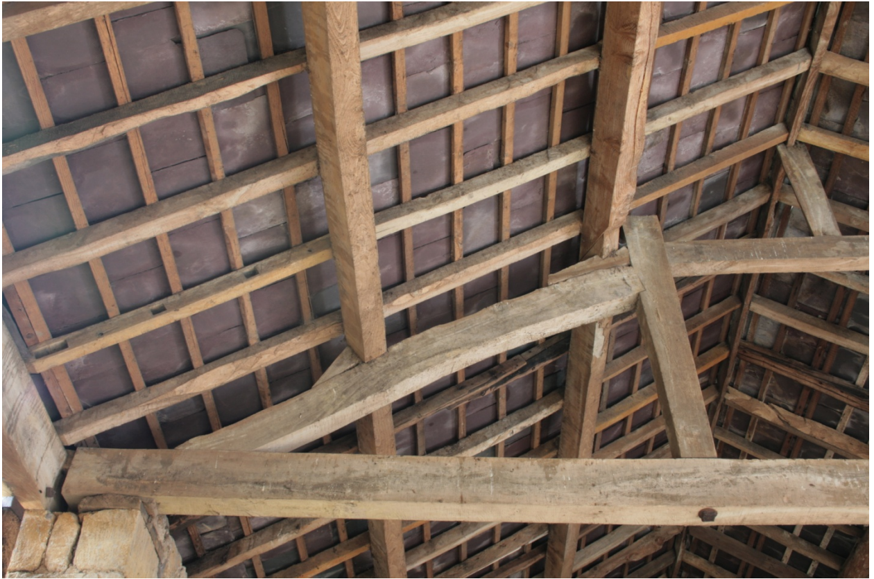
Plate 46: West end of south queen post truss main barn (Building B), looking north (CSFS17 D100 (30)) (viewpoint on Figure 11)
