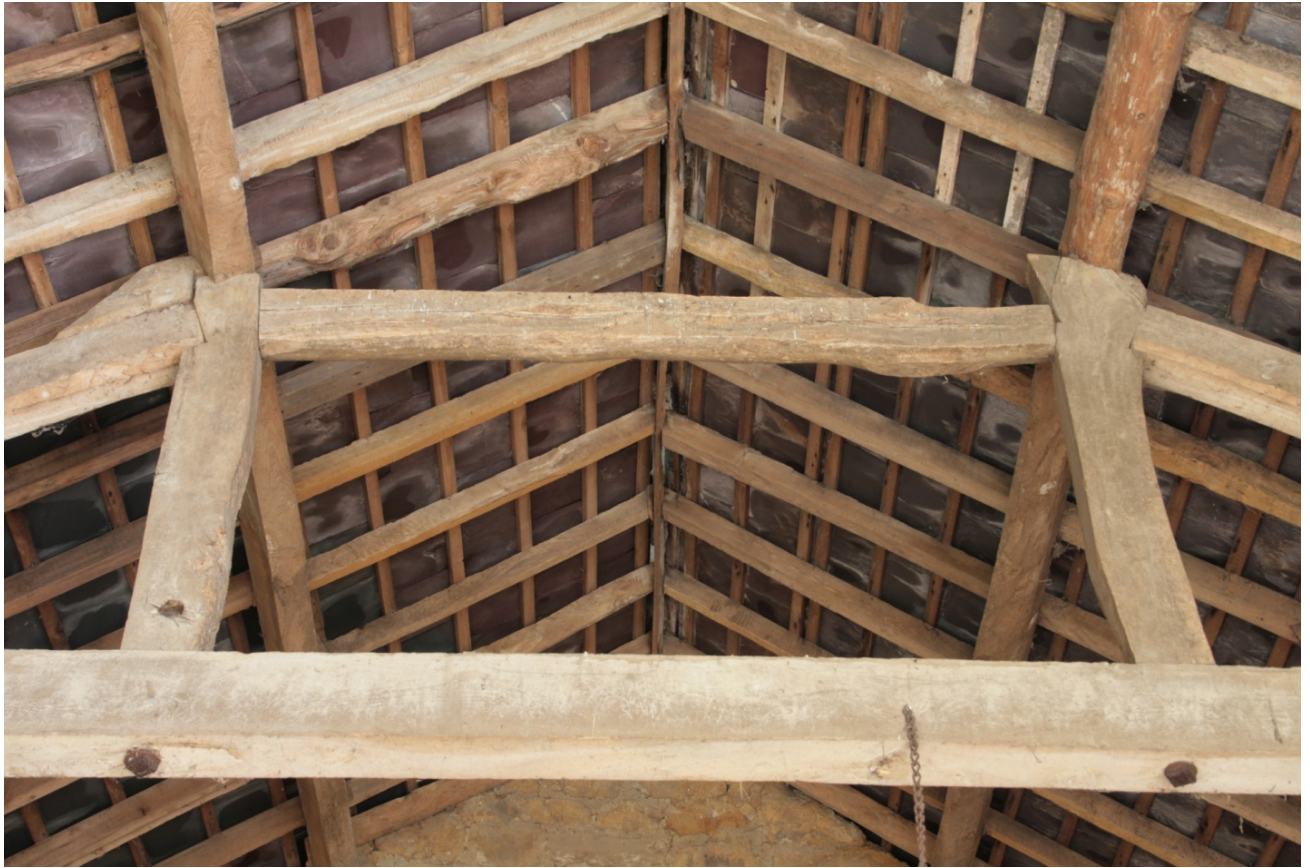
Plate 38: North queen post truss in main barn (Building B), looking north (CSFS17 D100 (4)) (viewpoint on Figure 11)
