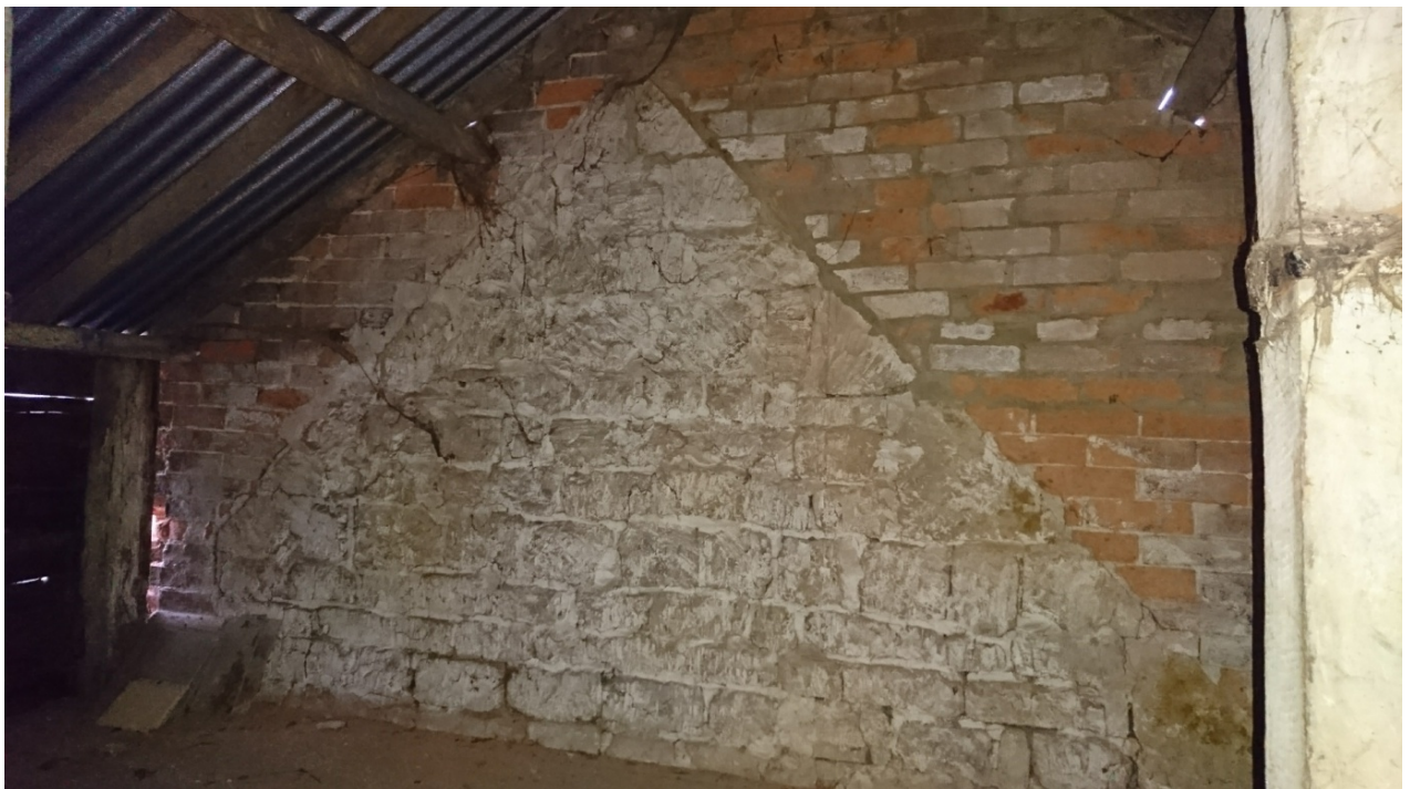
Plate 19: South gable of Building A, looking south (DSC_2340) (viewpoint on Figure 10)
