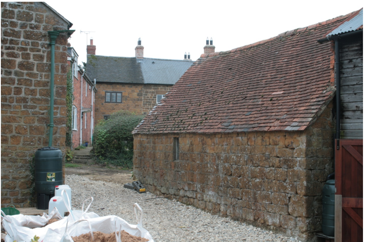
Plate 4: East elevation of barn (outside the Site) next to Building A (far right), looking south (CSFS17 D100 (77)) (viewpoint on Figure 9)
