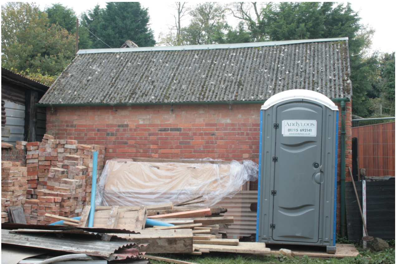
Plate 51: North elevation of Building C, looking south (CSFS17 D100 (70)) (viewpoint on Figures 9 and 12)
