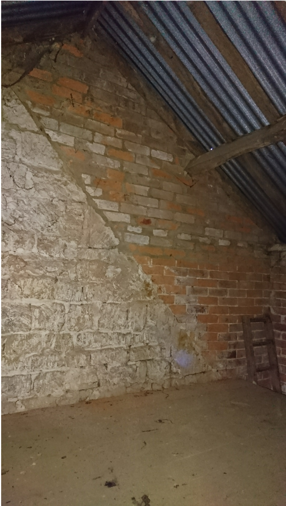
Plate 20: South gable of Building A, looking south (DSC_2339) (viewpoint on Figure 10)
