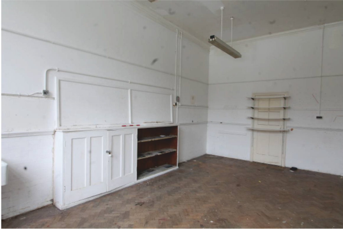
Plate 38 Classroom (27) looking south-east
