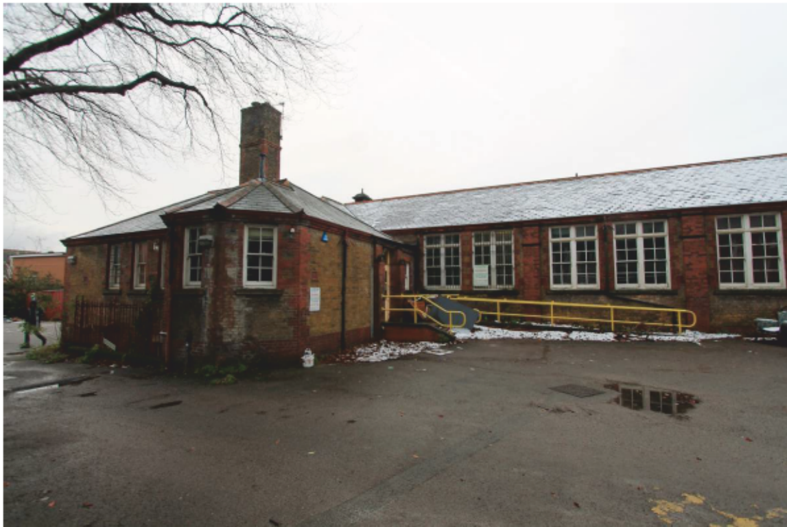
Plate 8a Eastern (Boys) classrooms, looking west
