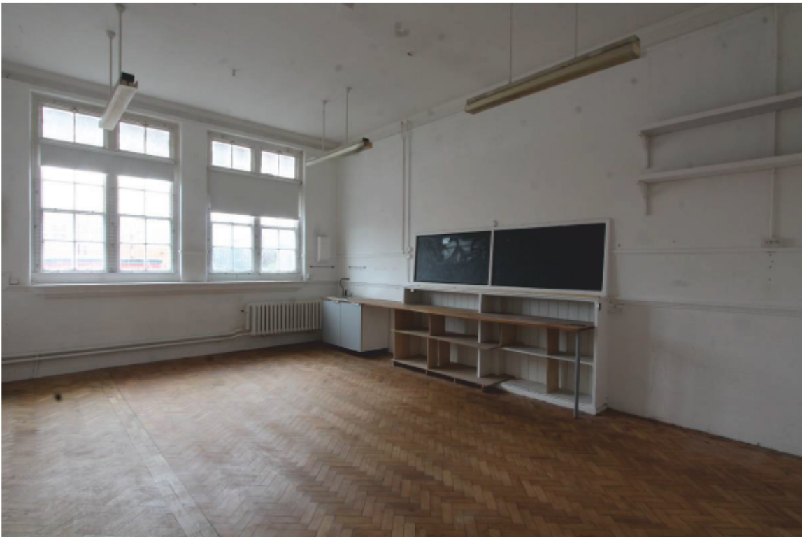
Plate 15 Classroom (10) looking south-west
