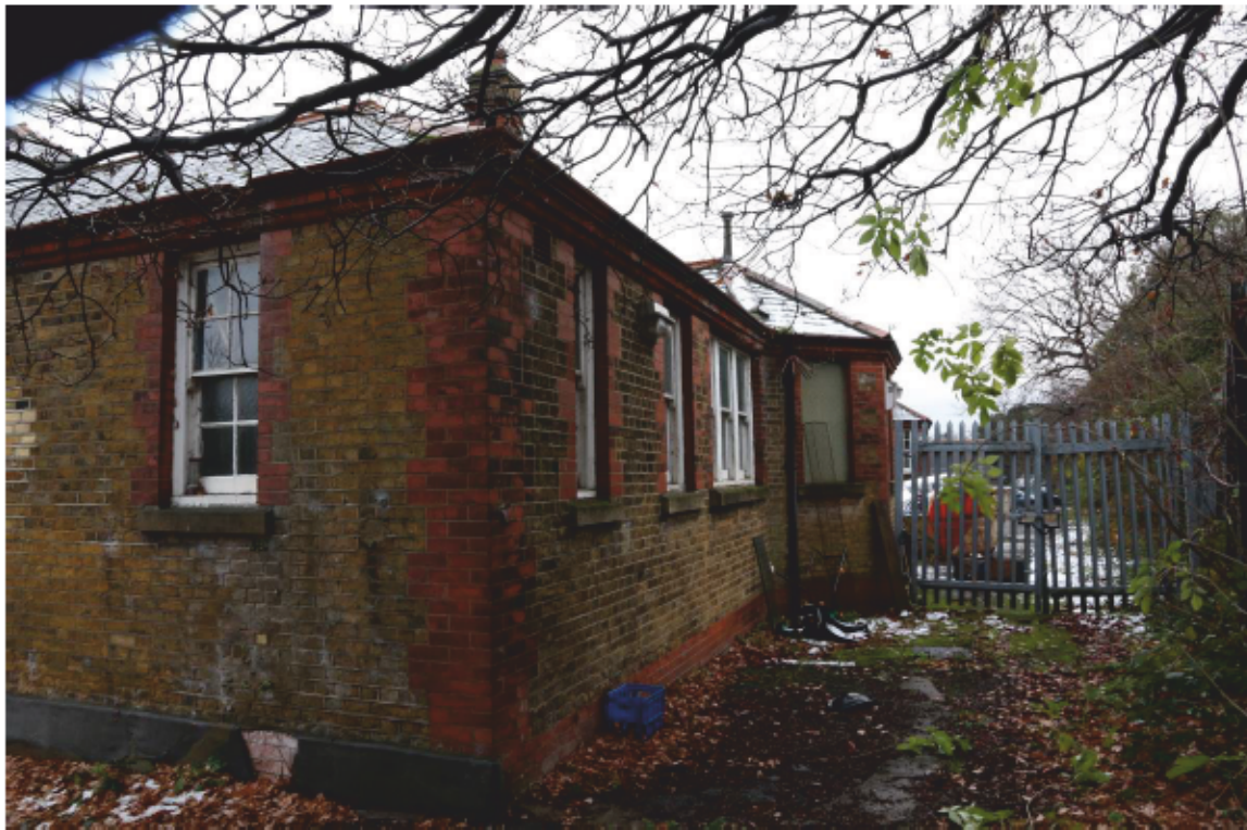
Plate 4c Western and Northern elevations facing south east
