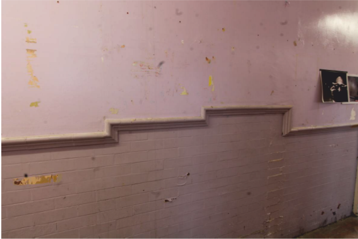
Plate 14 Stepped tile dado in corridor (9)
