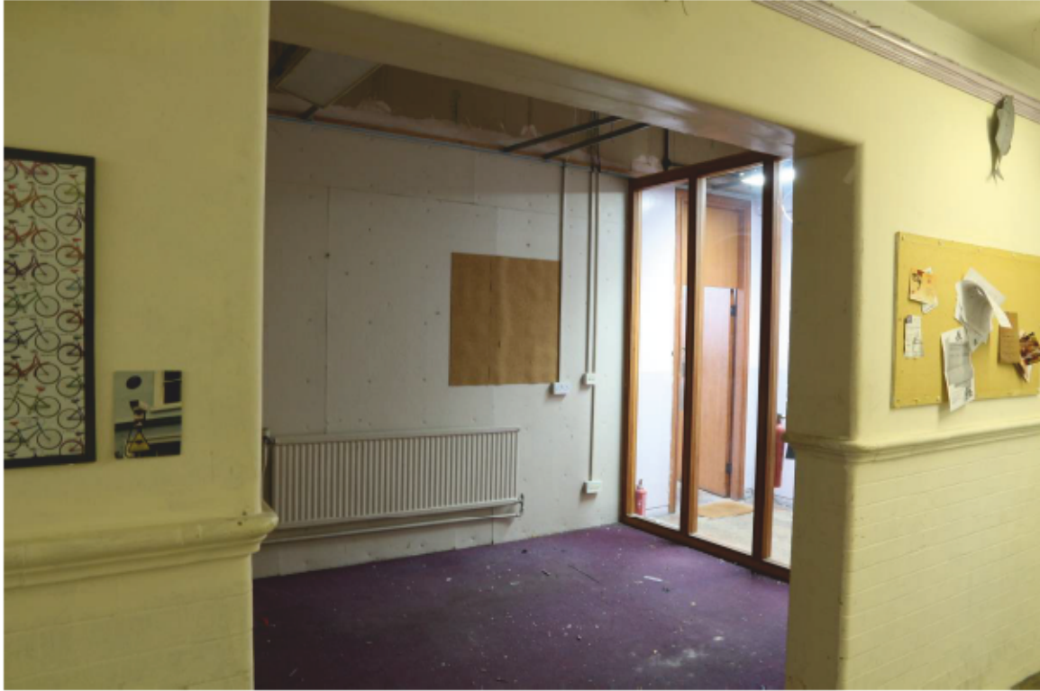
Plate 42 View into Classroom (5) from Corridor (6)
