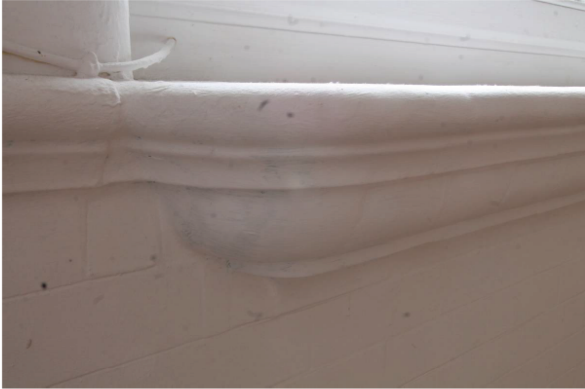
Plate 18 Detail of window sill and moulded apron (10)
