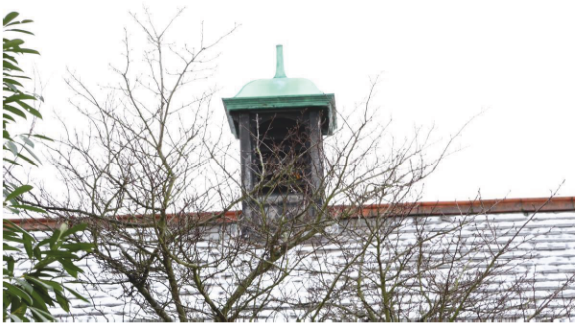
Plate 5 Detail of ventilation cupola with verdigris cap
