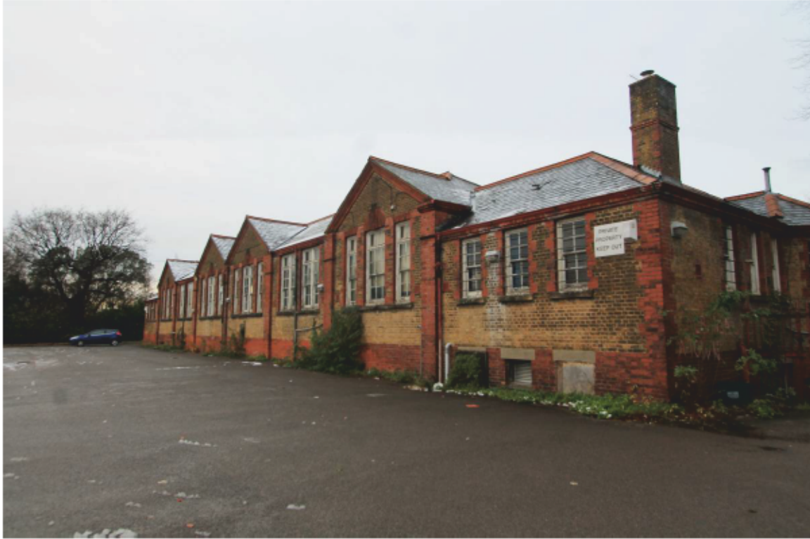
Plate 1 Southern Elevation, looking north-west
