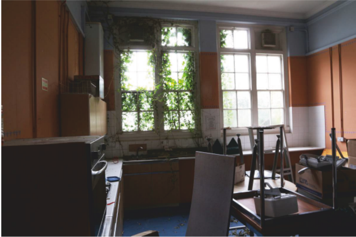
Plate 46 Classroom (29) looking north
