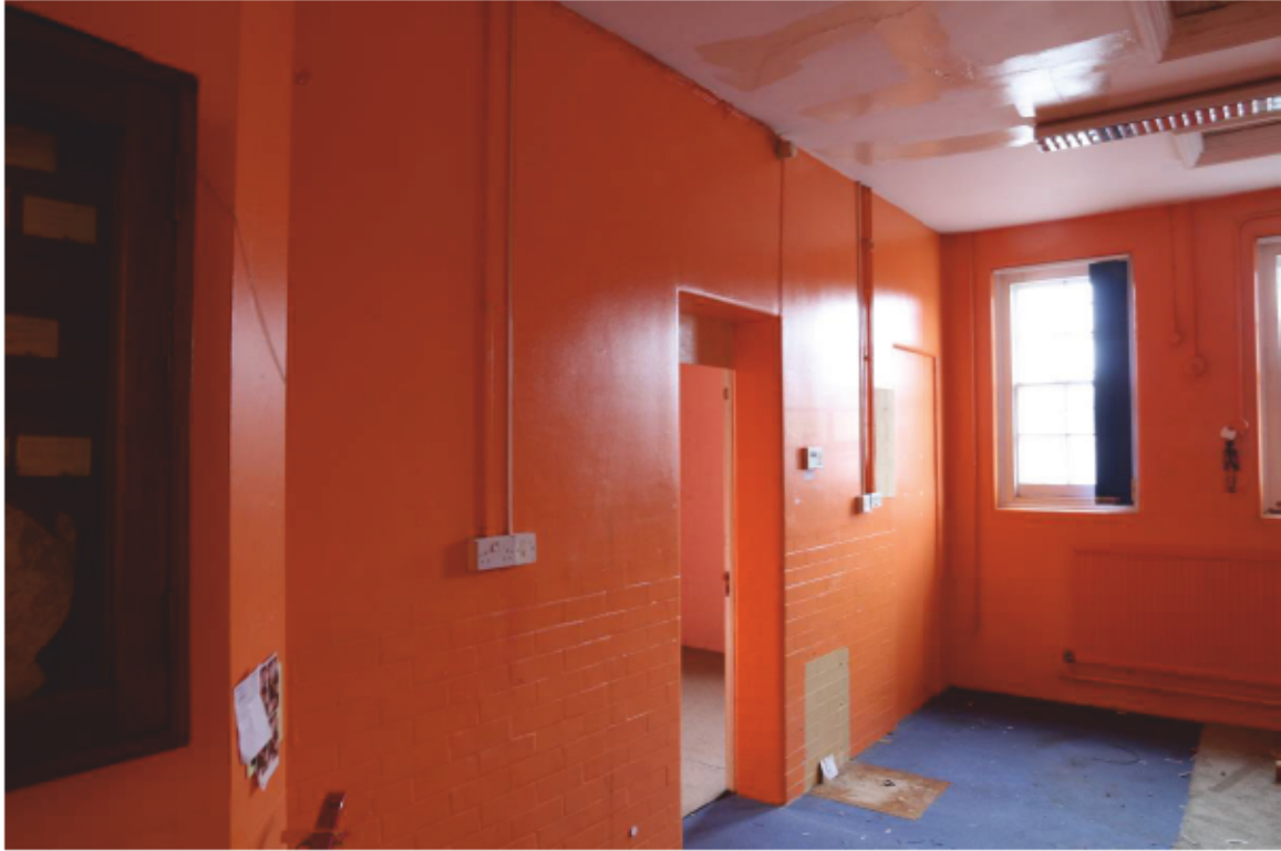
Plate 40 Former Boys Cloak Room (2), looking south-east
