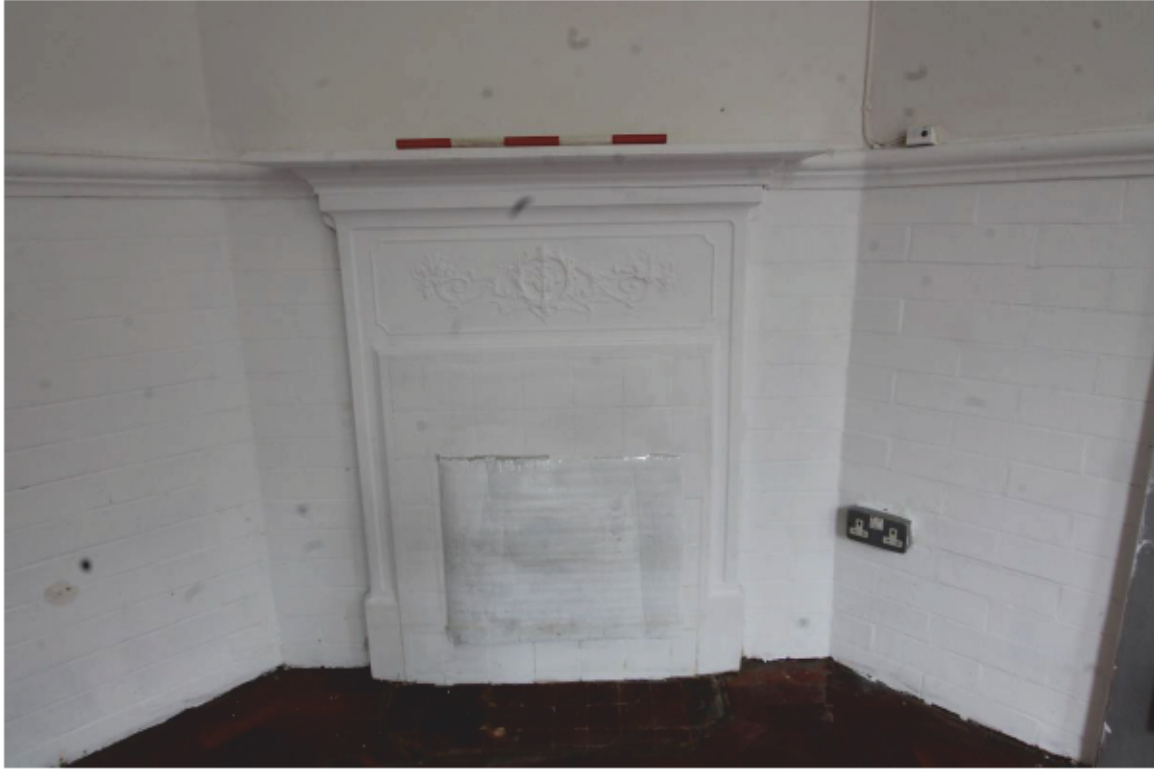
Plate 22 Cast-iron fire surround (13)
