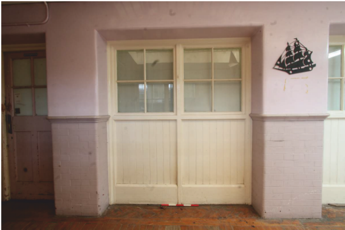
Plate 27 Part glazed timber partition in (16)
