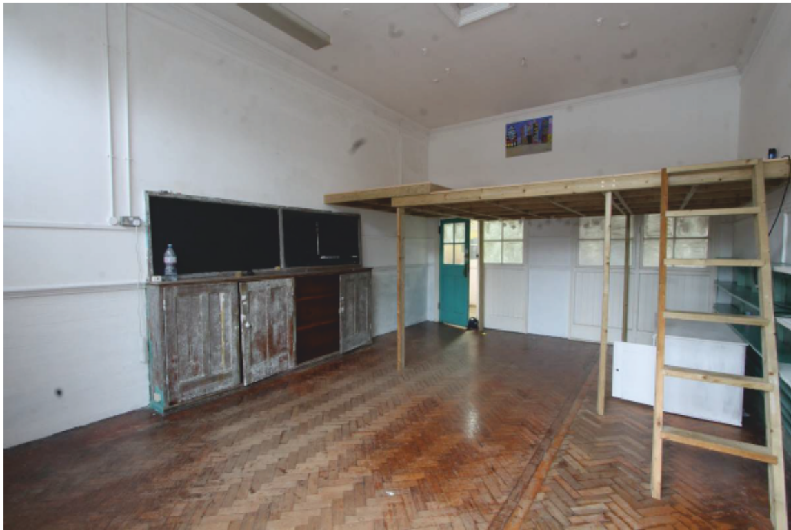
Plate 31 Classroom (19) with inserted mezzanine floor
