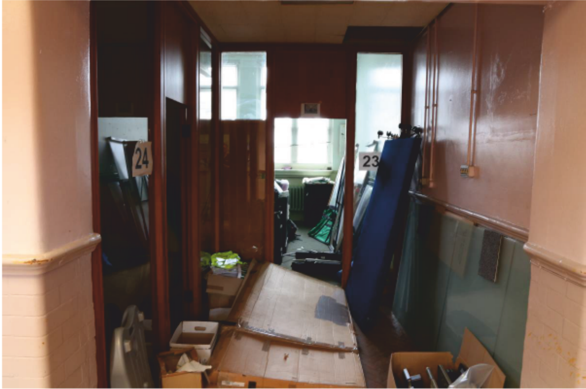
Plate 50 View to classroom (34) looking east
