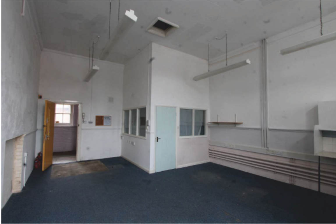
Plate 20 Classroom (11) looking north-east
