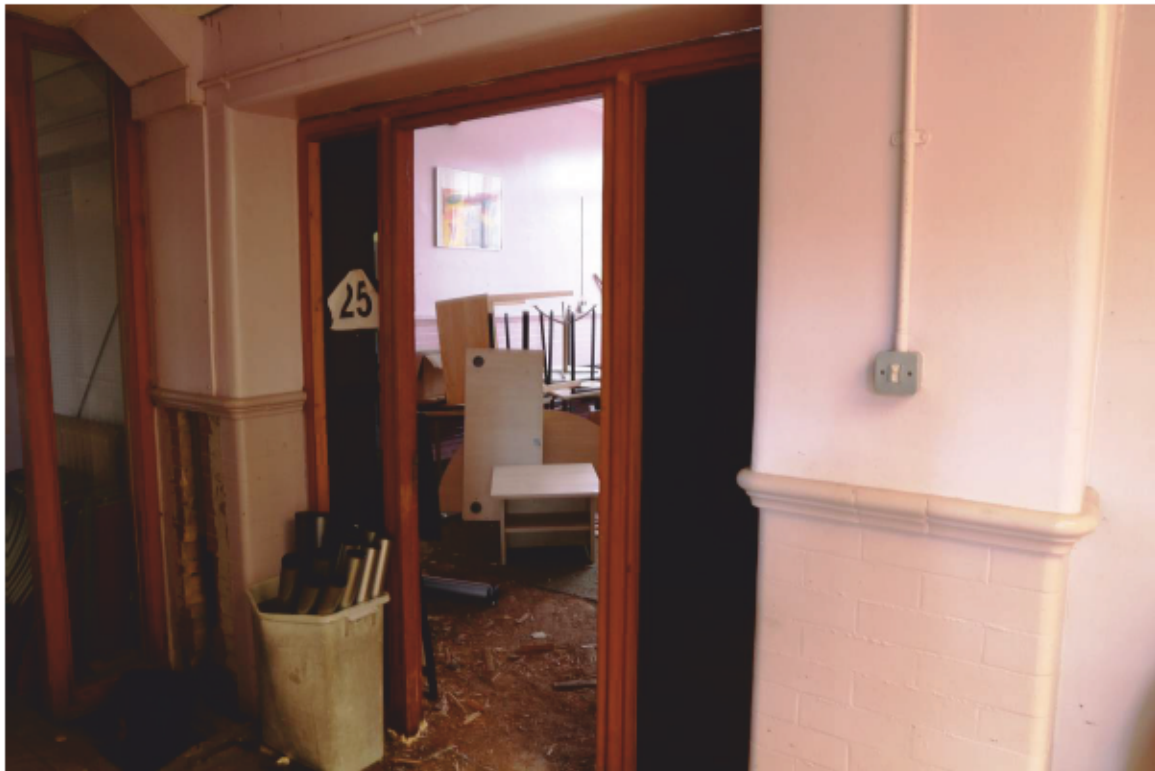
Plate 49 View to classroom (33) from corridor (37)
