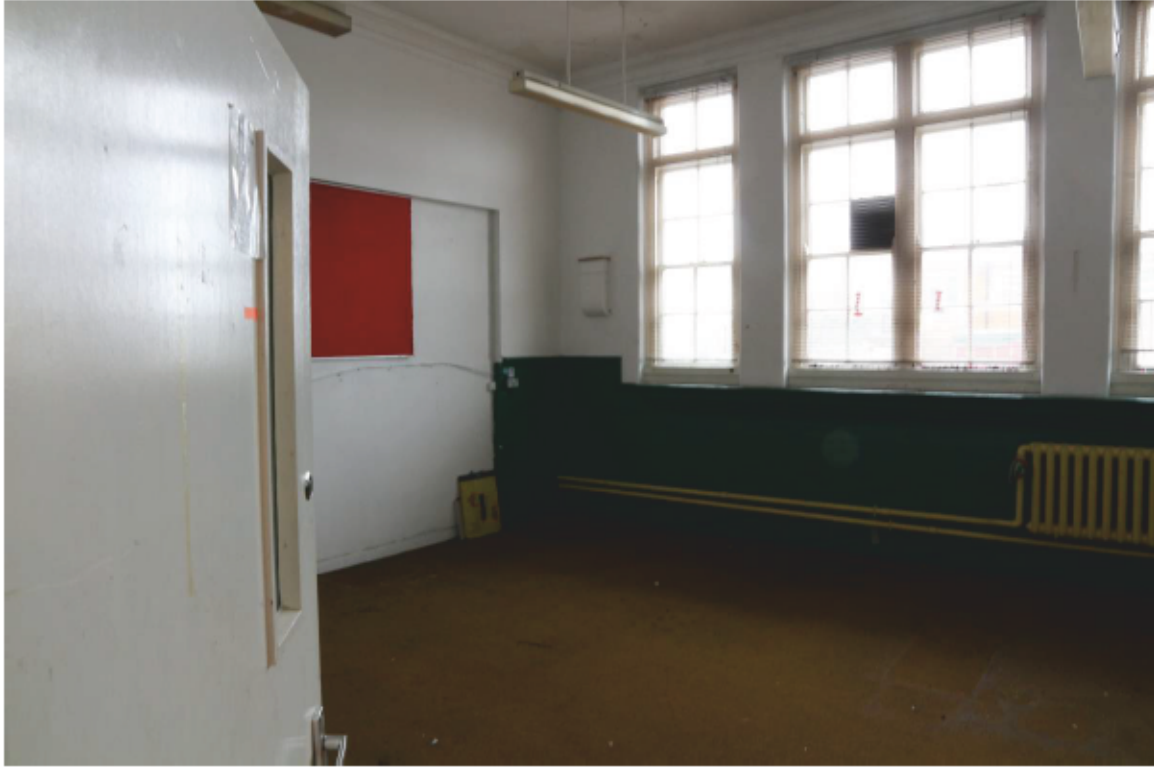
Plate 44 Classroom (7) looking south-east
