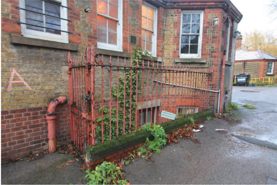
Plate 7 Railings around external access to basement, looking north-west
