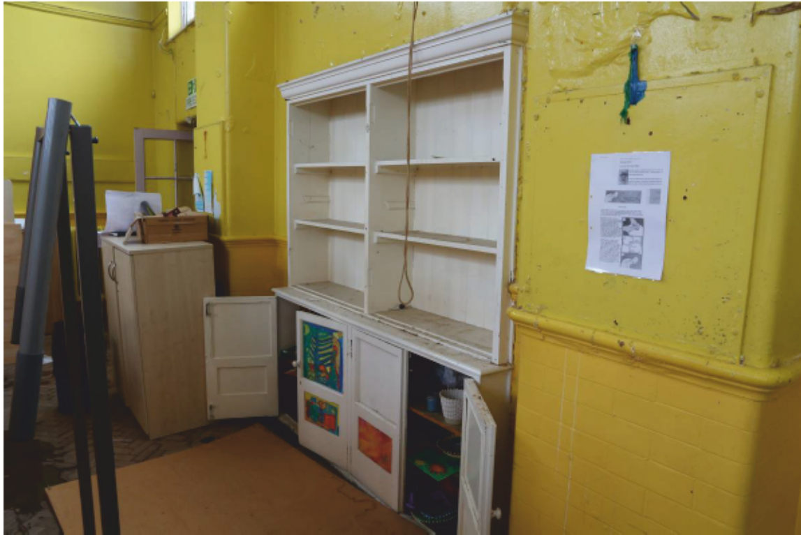
Plate 52 Built-in cupboard/shelving unit in Assembly Hall (36) looking south-west
