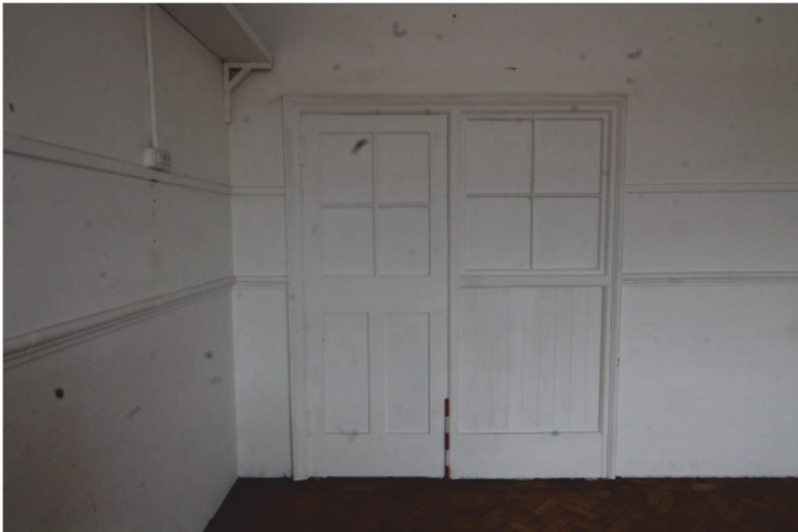
Plate 17 Detail of 'blocked' part-glazed door and side panel (10)
