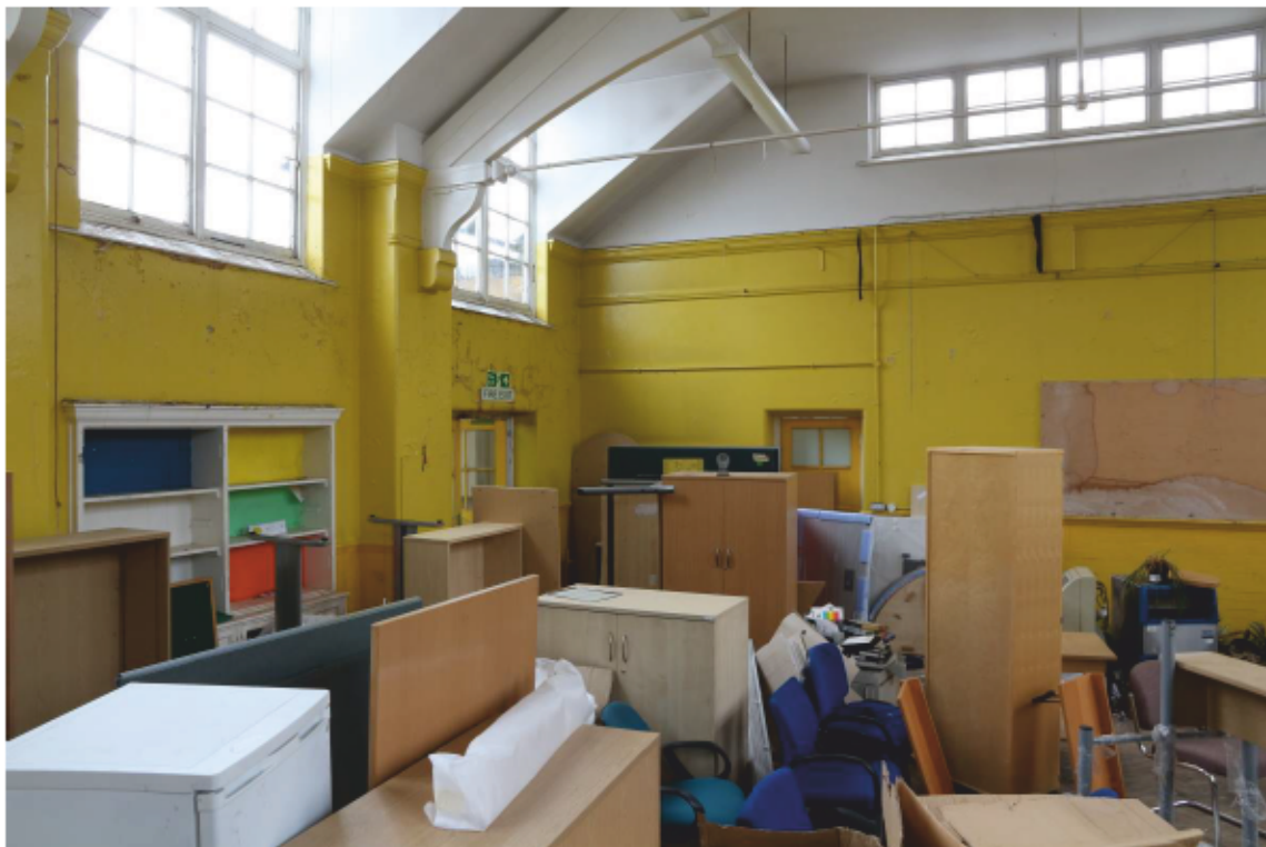
Plate 53: Built-in cupboard/shelving unit in Assembly Hall (36) looking north-west
