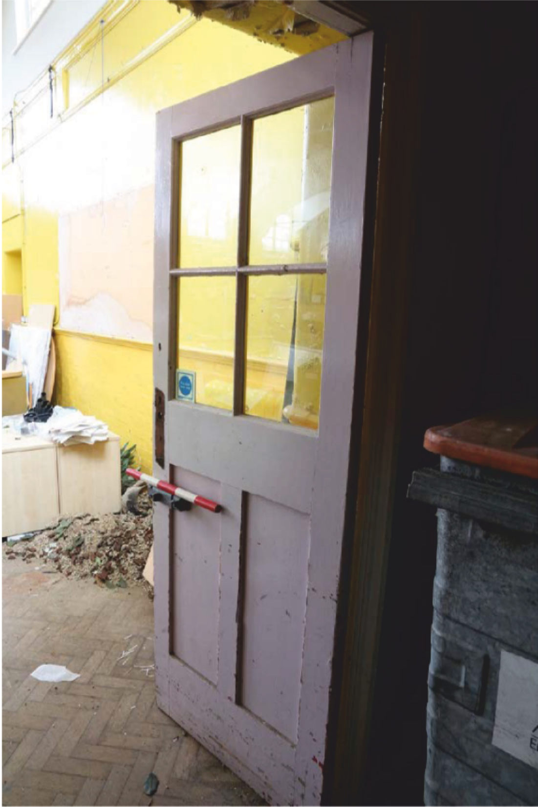
Plate 54: Floor in Assembly Hall (36) showing scar of stage/platform, looking north-west
