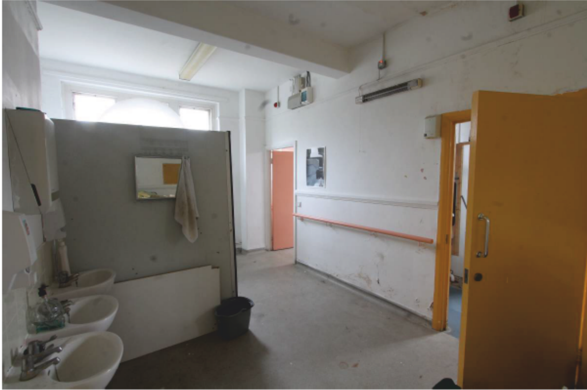
Plate 34 Former Cloak Room (22) now WCs
