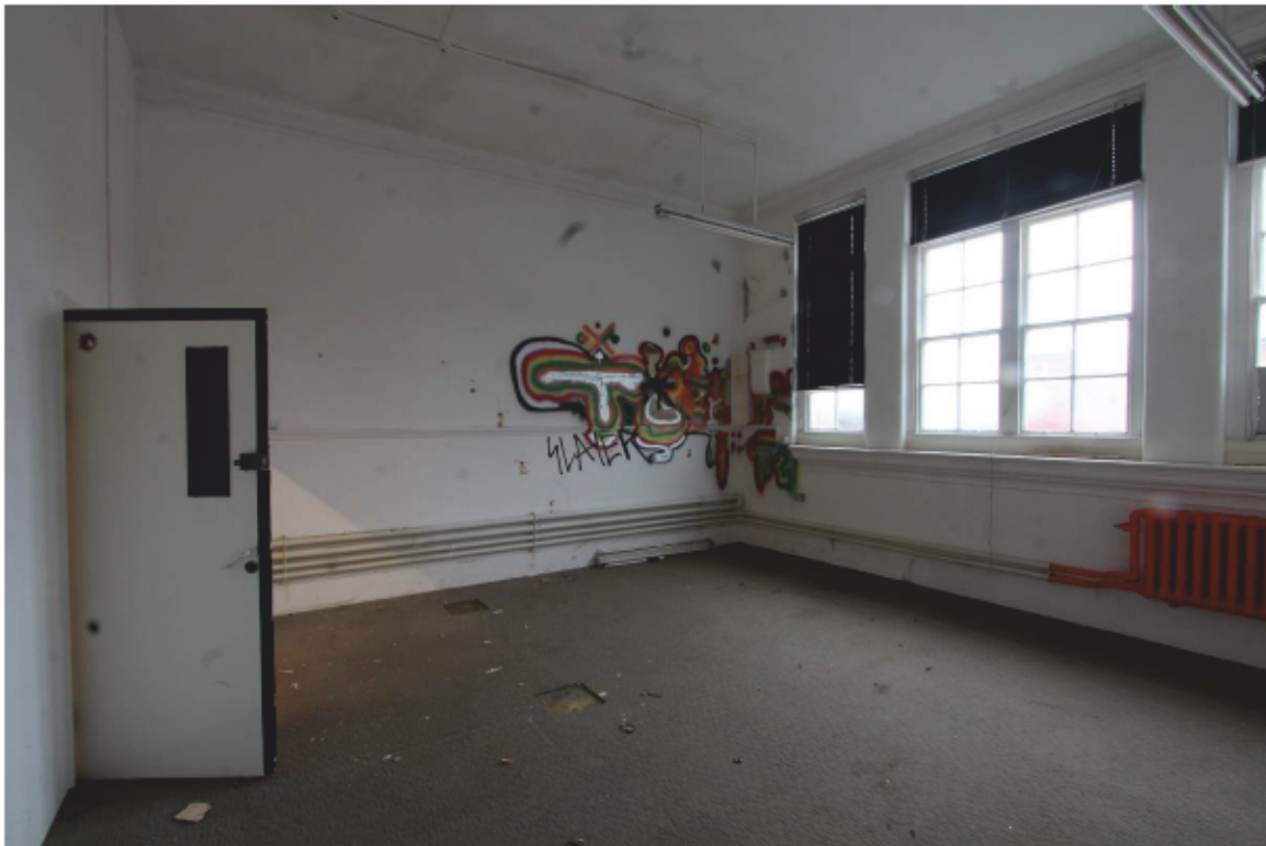
Plate 13 Classroom (8) looking south-east
