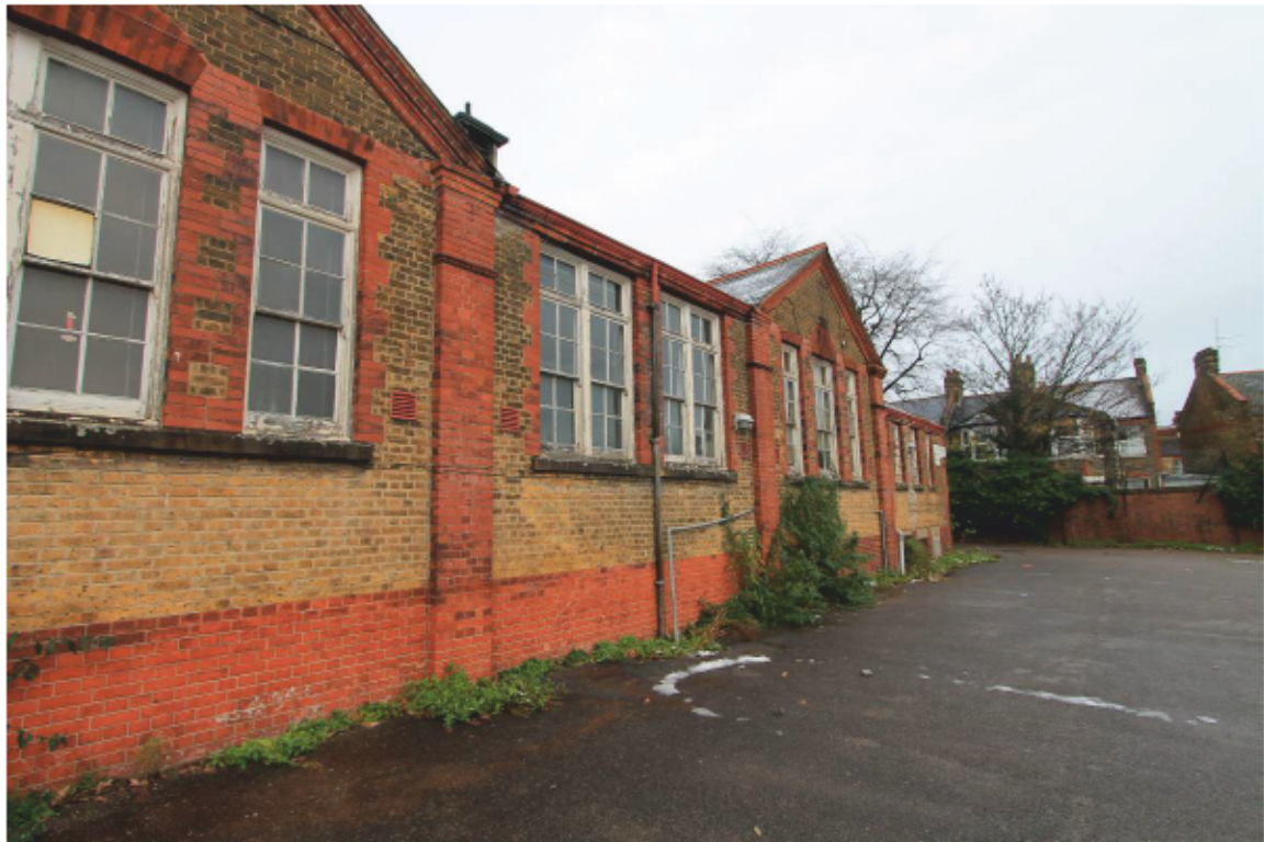
Plate 2 Southern Elevation, looking north-east
