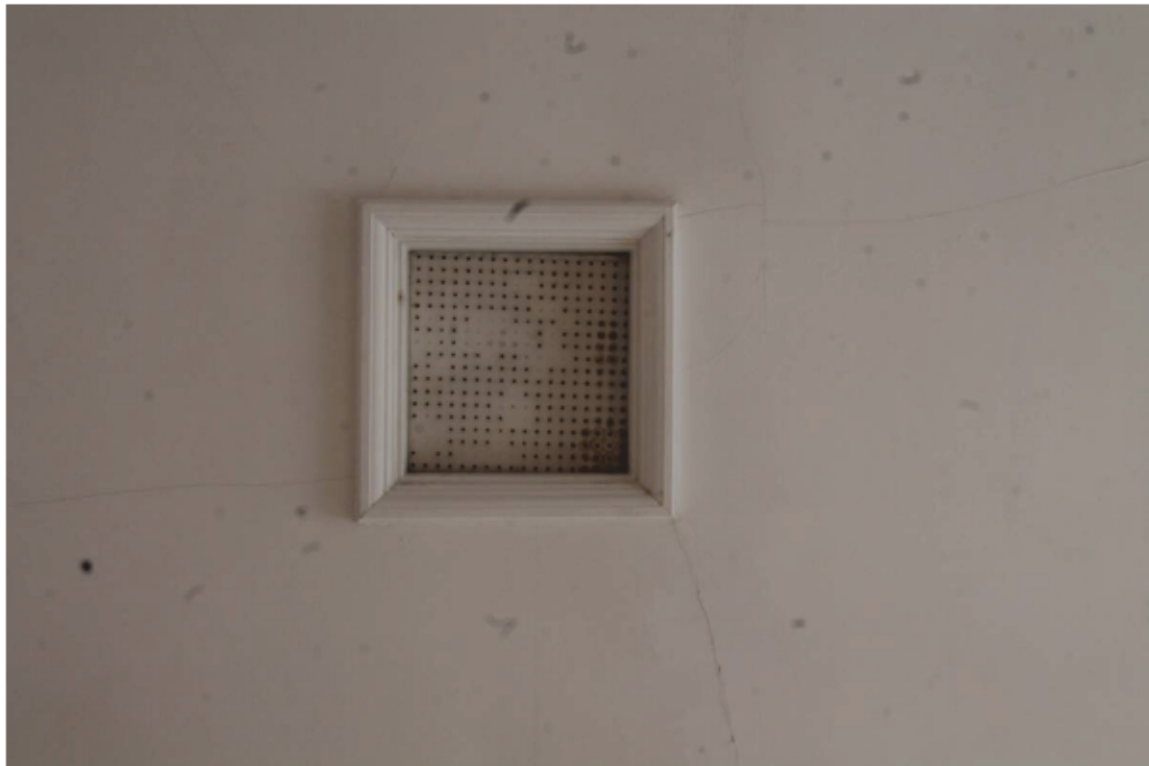
Plate 19 Ventilated ceiling hatch (10)
