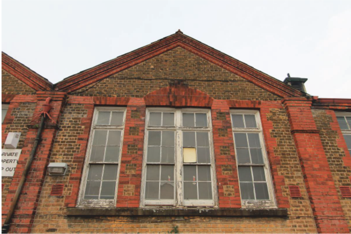
Plate 3 Detail of decorative brickwork, gaugework and fenestration
