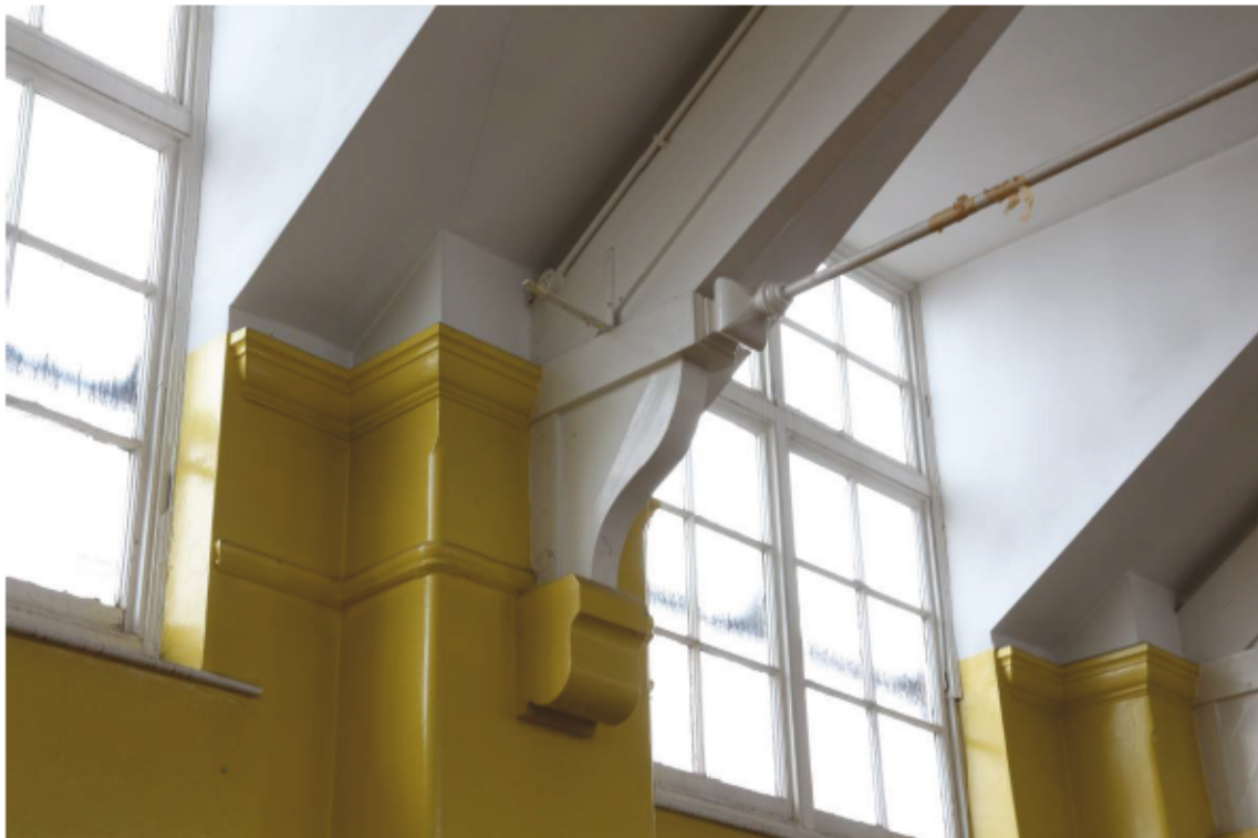
Plate 56: Dormer windows in Assembly Hall (36), looking south-east
