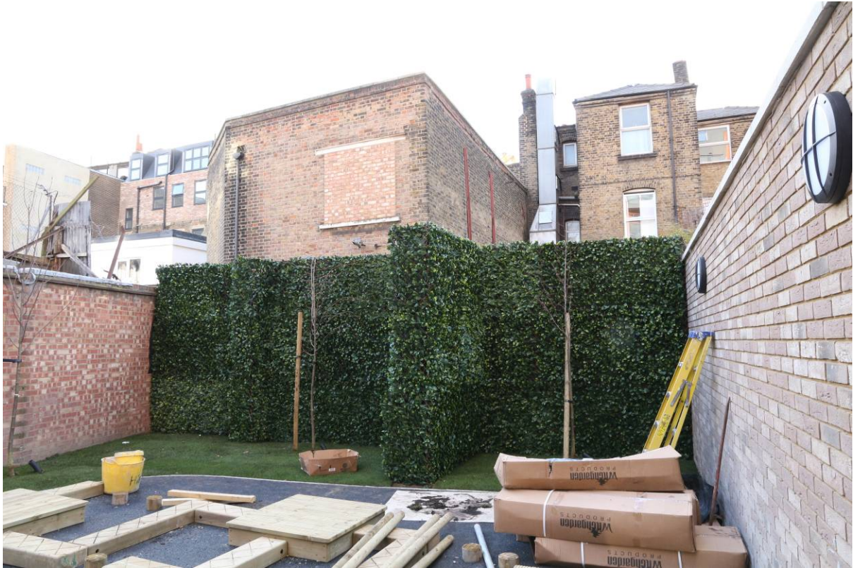
Plate 54 Photograph of the south end of the site taken in December 2017 (PCA) showing rear (east) elevations of buildings along Walworth Road, looking west (viewpoint on Figure 19)
