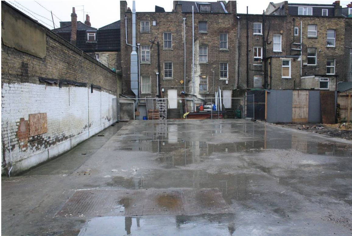
Plate 5 Photograph taken in March 2014 (CgMs part of RPS) showing north wall of Building 4 and concrete slab of Building 5 and rear (east) elevations of buildings along Walworth Road, looking west (viewpoint on Figure 17)
