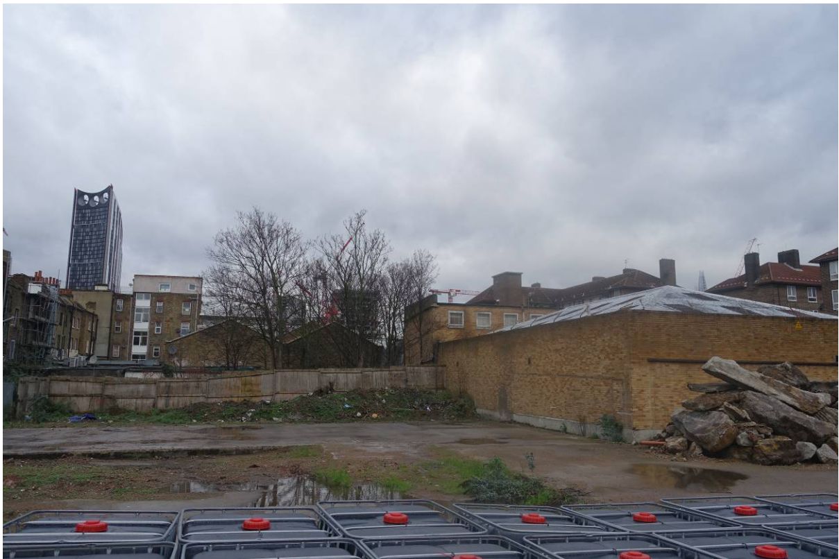
Plate 27 Photograph taken in early 2017 (CField Construction) showing York House (right), looking north (viewpoint on Figure 18)
