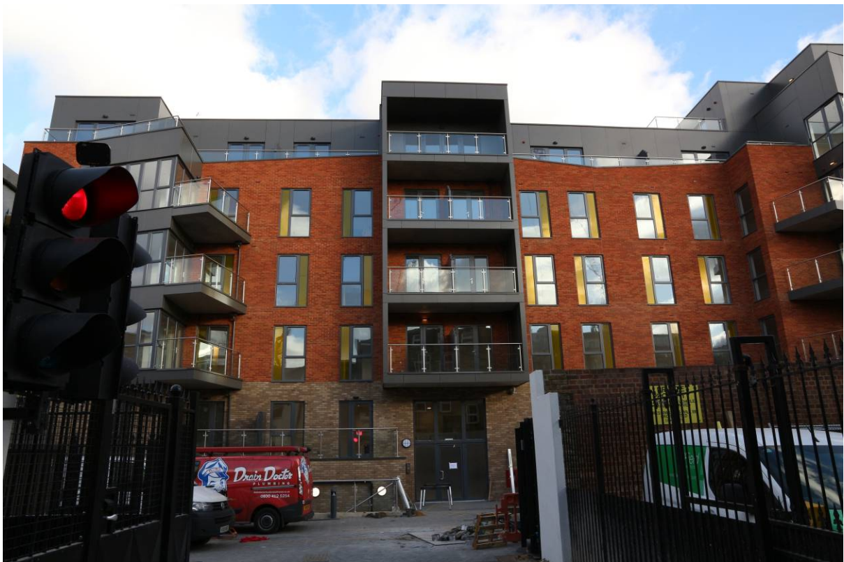
Plate 49 Photograph taken in December 2017 (PCA) from site entrance of the newly constructed east building, looking east (viewpoint on Figure 19)
