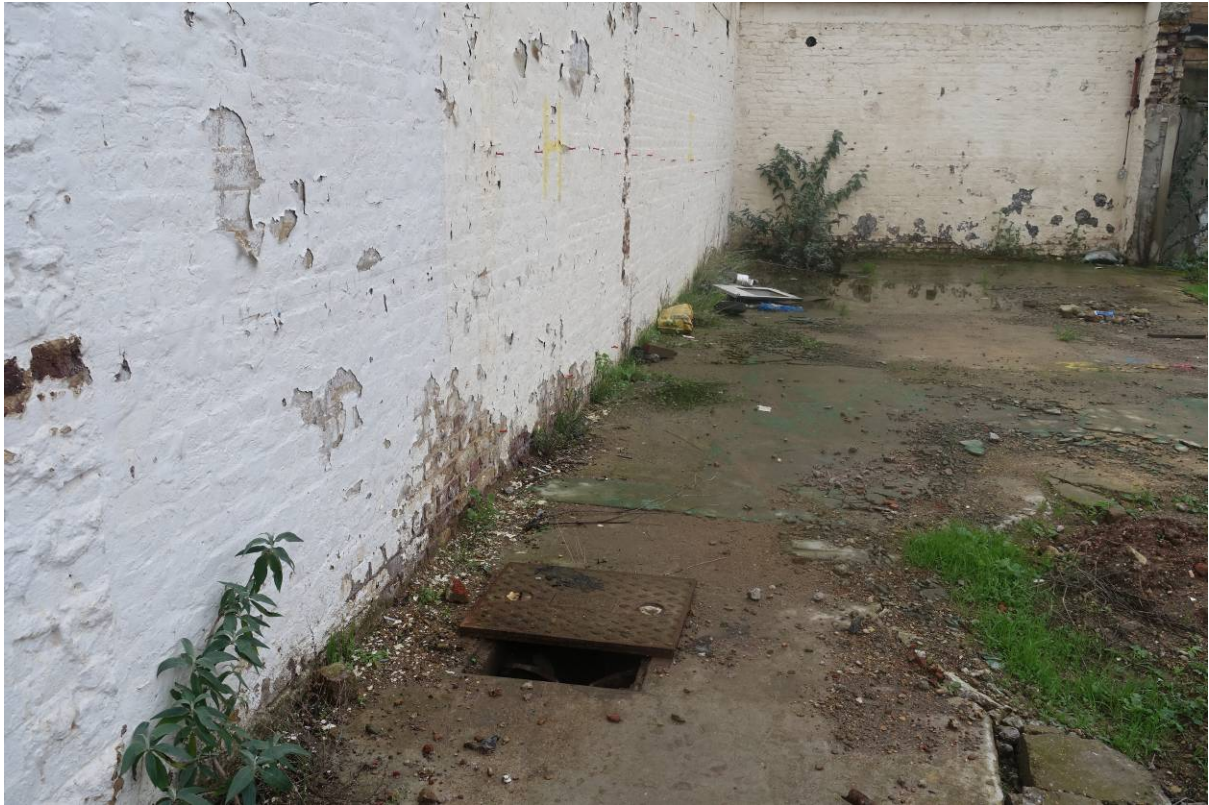
Plate 40 Photograph taken in early 2017 (CField Construction) of the boundary wall, looking south-east (viewpoint on Figure 18)
