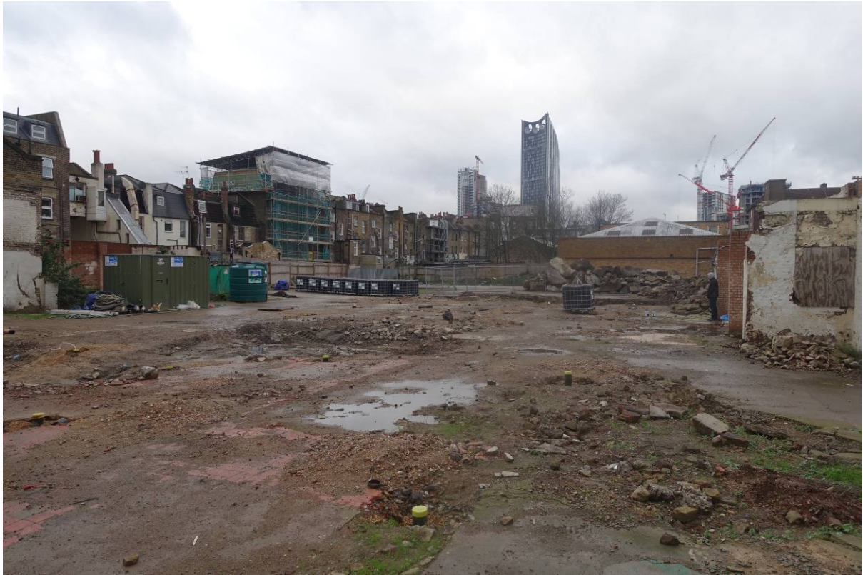
Plate 26 Photograph of site taken in early 2017 (CField Construction) showing rear (east) elevations of buildings along Walworth Road, looking north-west (viewpoint on Figure 18)
