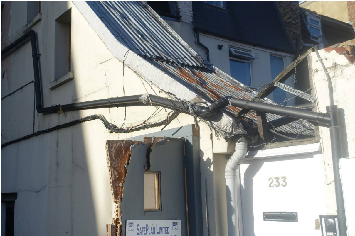
Plate 24 Photograph taken in early 2017 (CField Construction) showing north side of site entrance, looking north-west (viewpoint on Figure 18)
