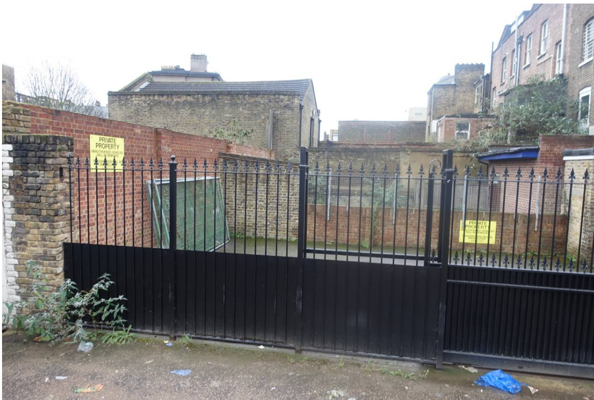
Plate 43 Photograph taken in early 2017 (CField Construction) showing the north elevation of building to the rear (east) of no. 243 Walworth Road and rear (east) elevations of buildings along Walworth Road (right), looking south (viewpoint on Figure 18)
