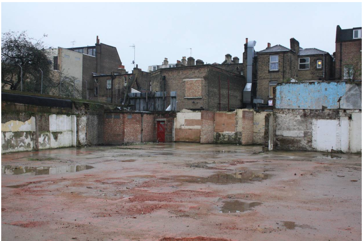
Plate 14 Photograph taken in March 2014 (CgMs part of RPS) of site boundary wall and rear (east) elevations of buildings along Walworth Road, looking south-west (viewpoint on Figure 17)
