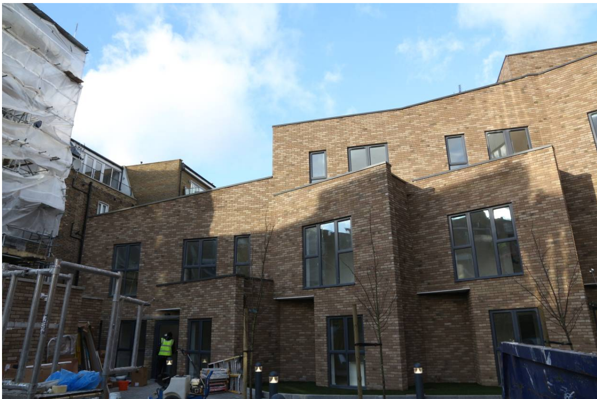
Plate 47 Photograph taken in December 2017 (PCA) of the newly constructed north building and the rear (east) elevations of buildings along Walworth Road (left), looking north-west (viewpoint on Figure 19)
