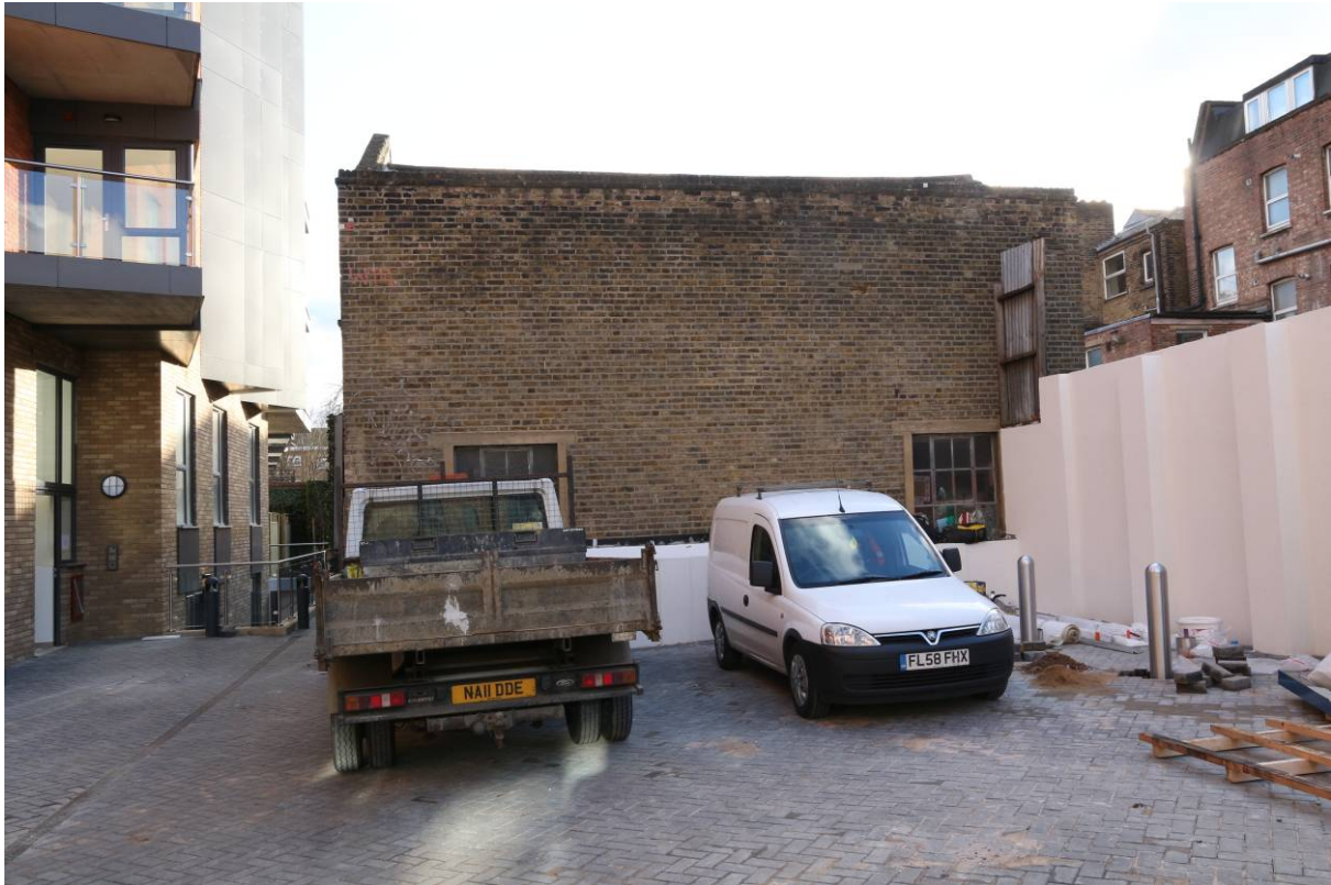
Plate 50 Photograph taken in December 2017 (PCA) of north elevation of building to the rear (east) of no. 243 Walworth Road, looking south (viewpoint on Figure 19)
