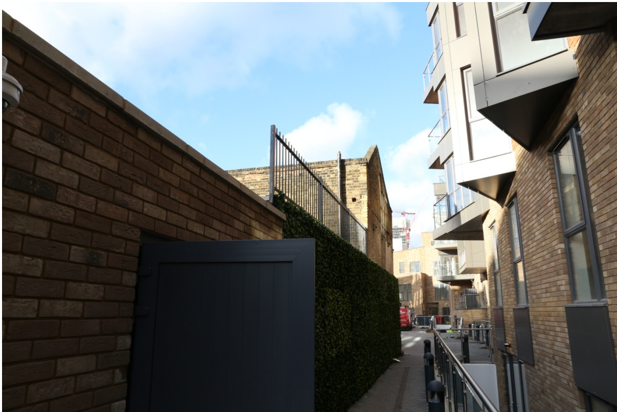
Plate 53 Photograph taken in December 2017 (PCA) of east elevation of building to the rear (east) of no. 243 Walworth Road (left) and newly constructed building (right), looking north (viewpoint on Figure 19)
