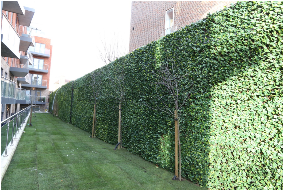
Plate 60 Photograph taken in December 2017 (PCA) of the boundary wall with the newly constructed building (left), and Southey House (right) beyond, looking north (viewpoint on Figure 18)
