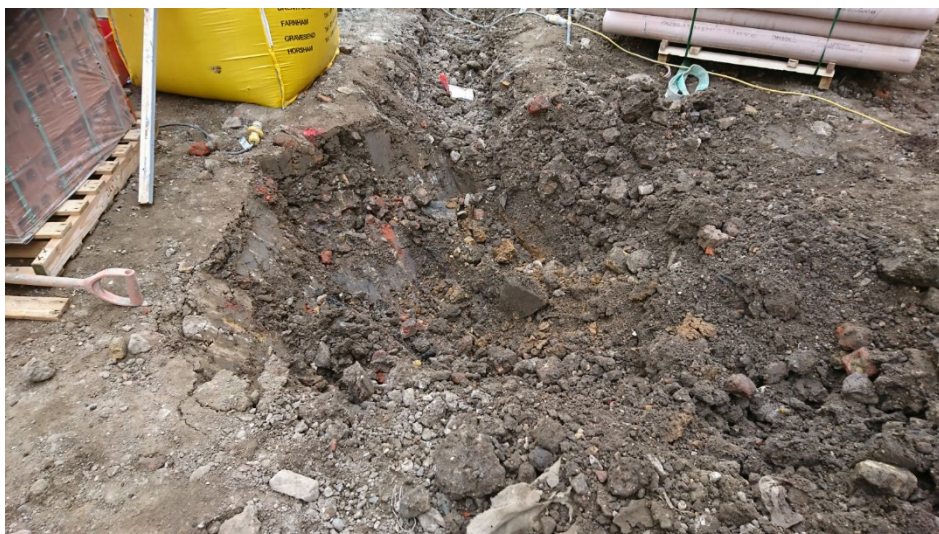
Plate 2: View of SWMH01, showing ground conditions at depths up to 0.5m bgl
