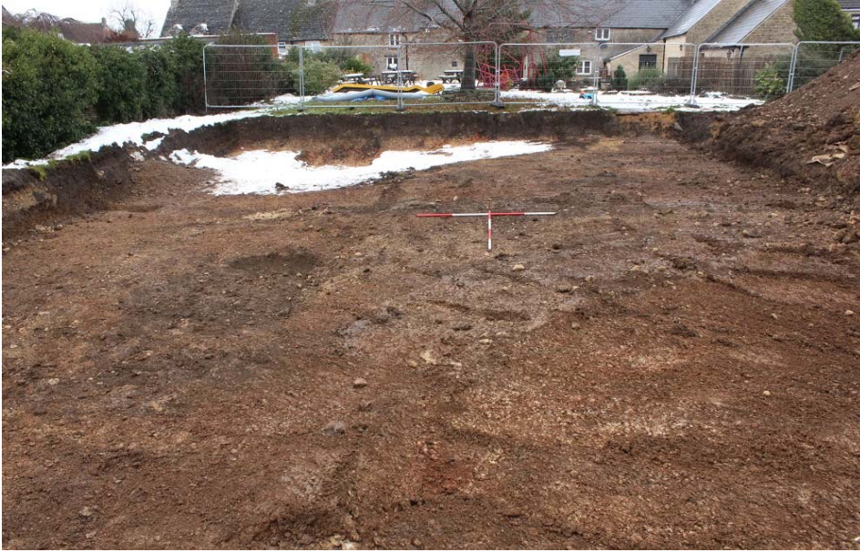
Plate 1. General view, western side of the Site, view to north.
