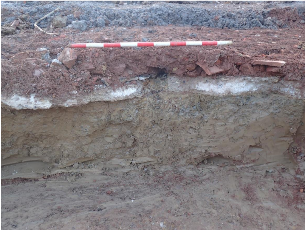
Plate 5: Trench 5 section looking east. 1 m scale.
