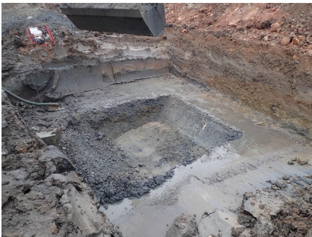
Plate 4: Trench 1 facing south west
