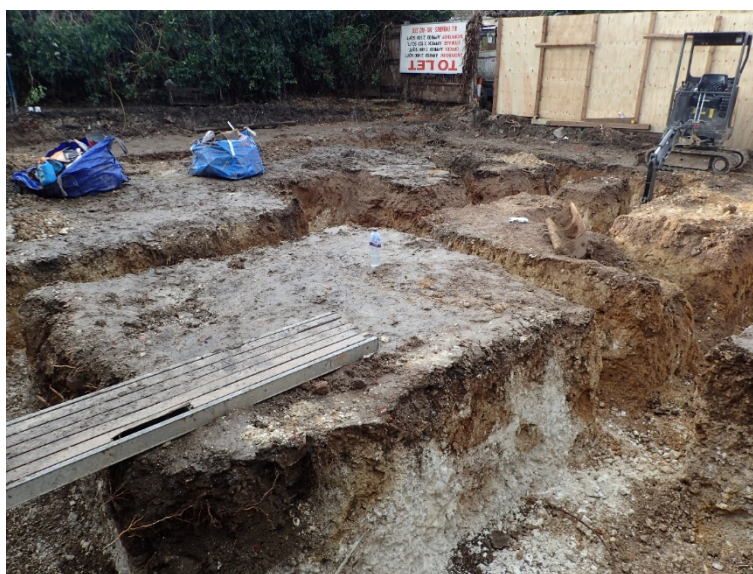
Plate 1: Site Overview, Facing West
