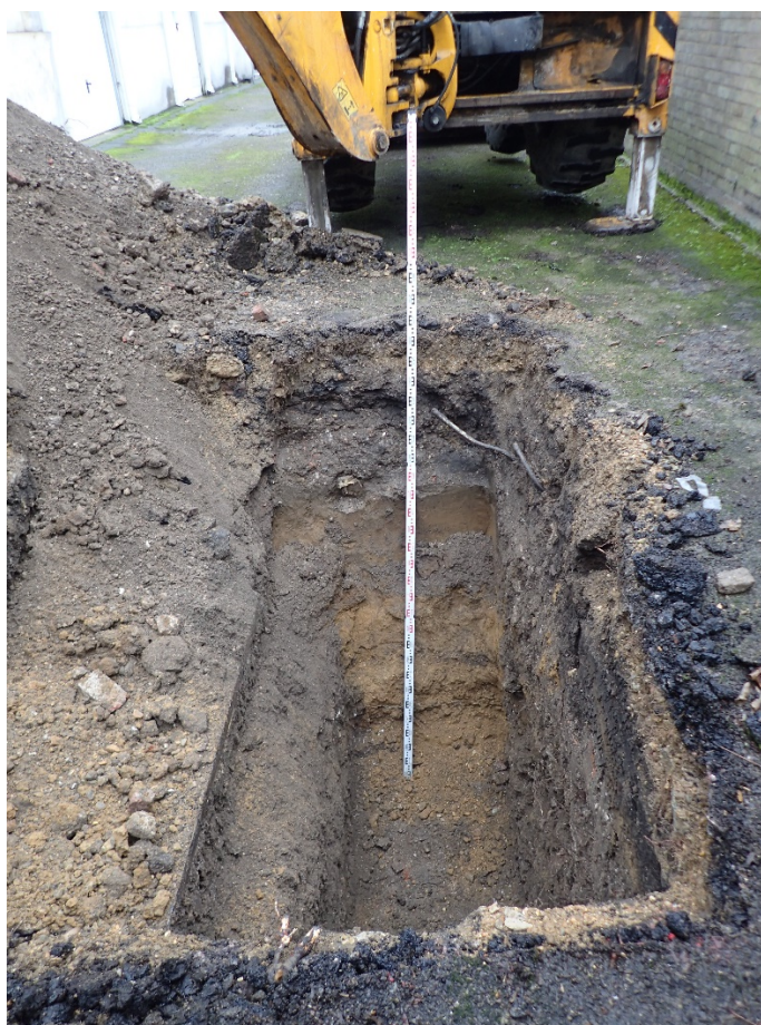
Plate 6: Section 3 including sondage, Trench 3, West facing
