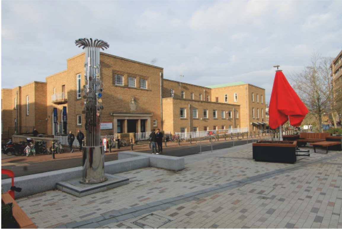
Plate 3 Percy Gee Building, East Wing, looking north-west
