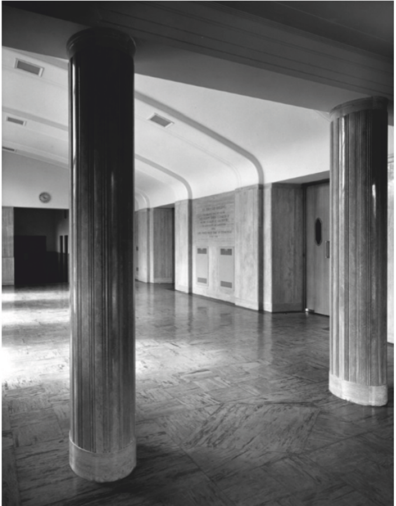
Historic Plate 5: Columns in Foyer (G2). ©University of Leicester
