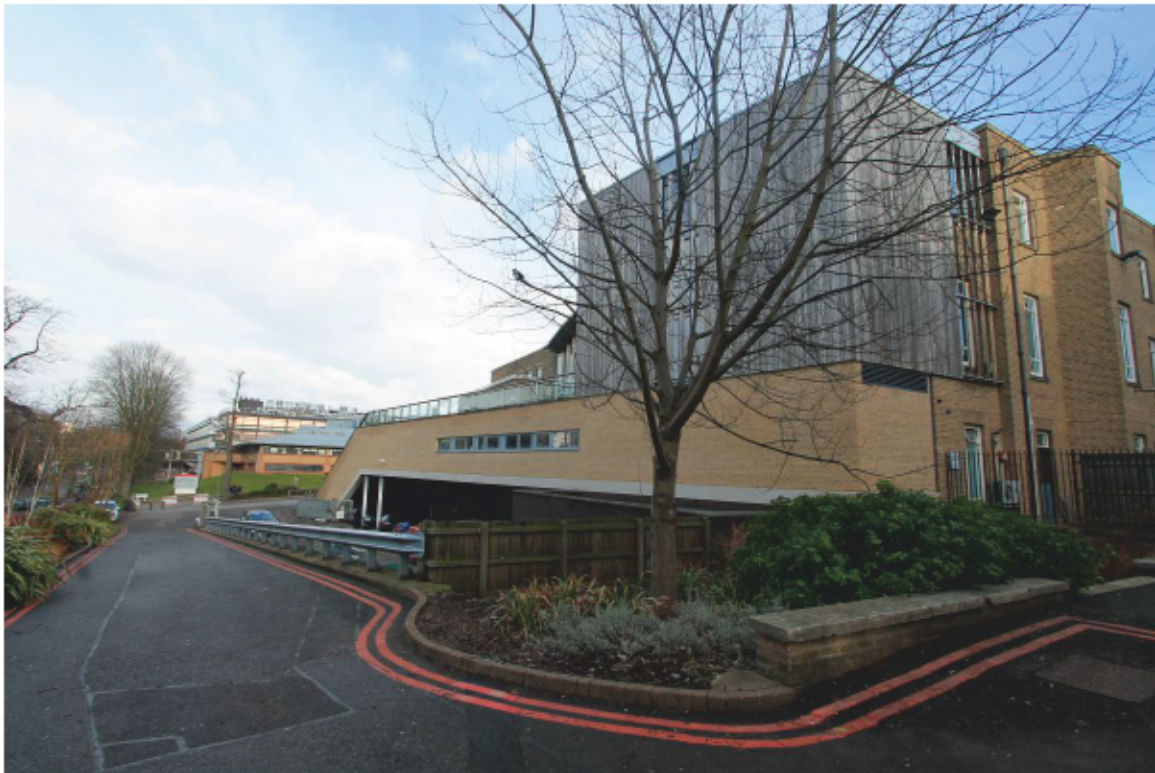
Plate 10 Percy Gee Building, west elevation, looking north-east
