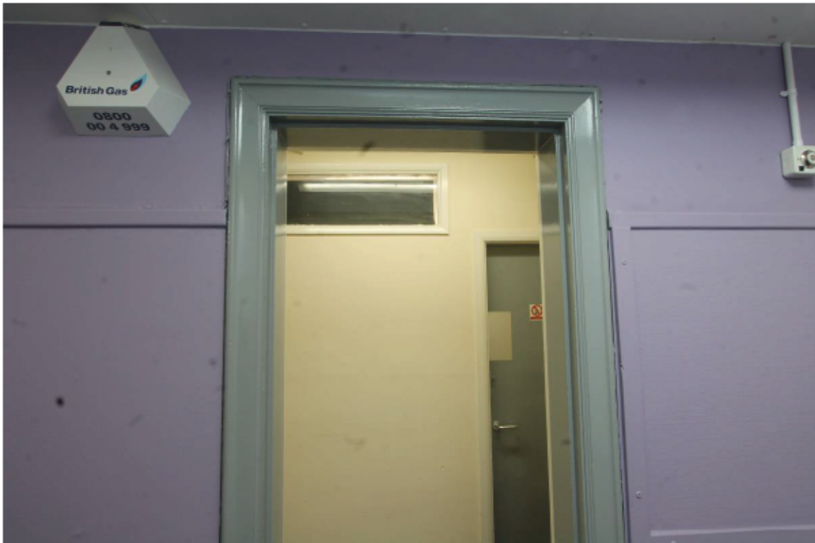
Plate 32 Unusual survival of door architrave (M9)
