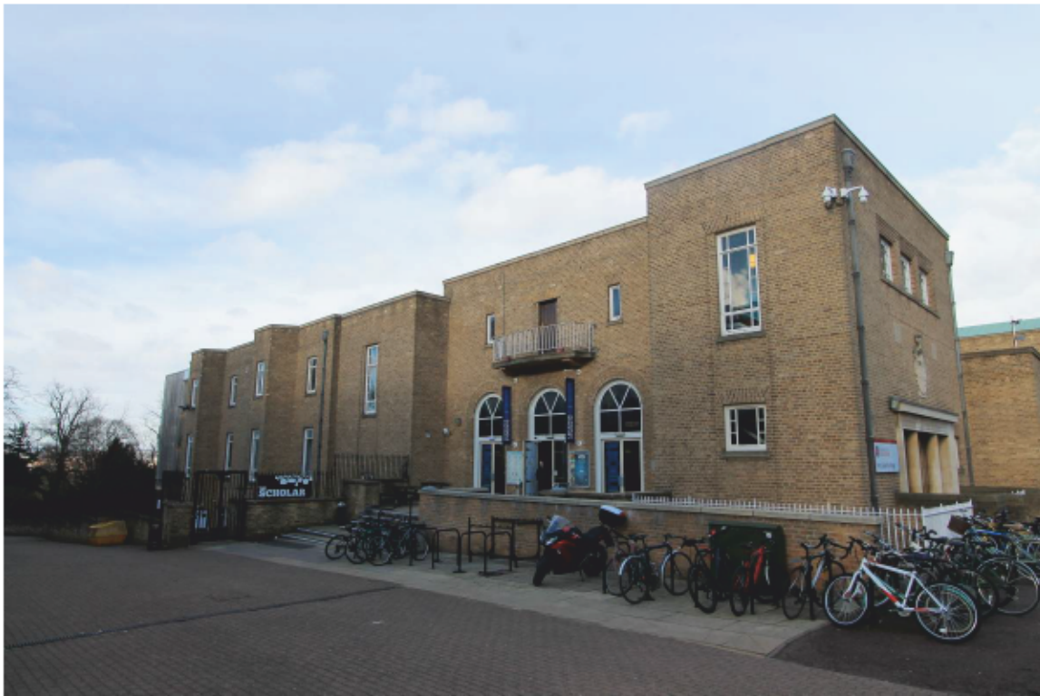
Plate 8 Percy Gee Building, Southern Elevation, looking north
