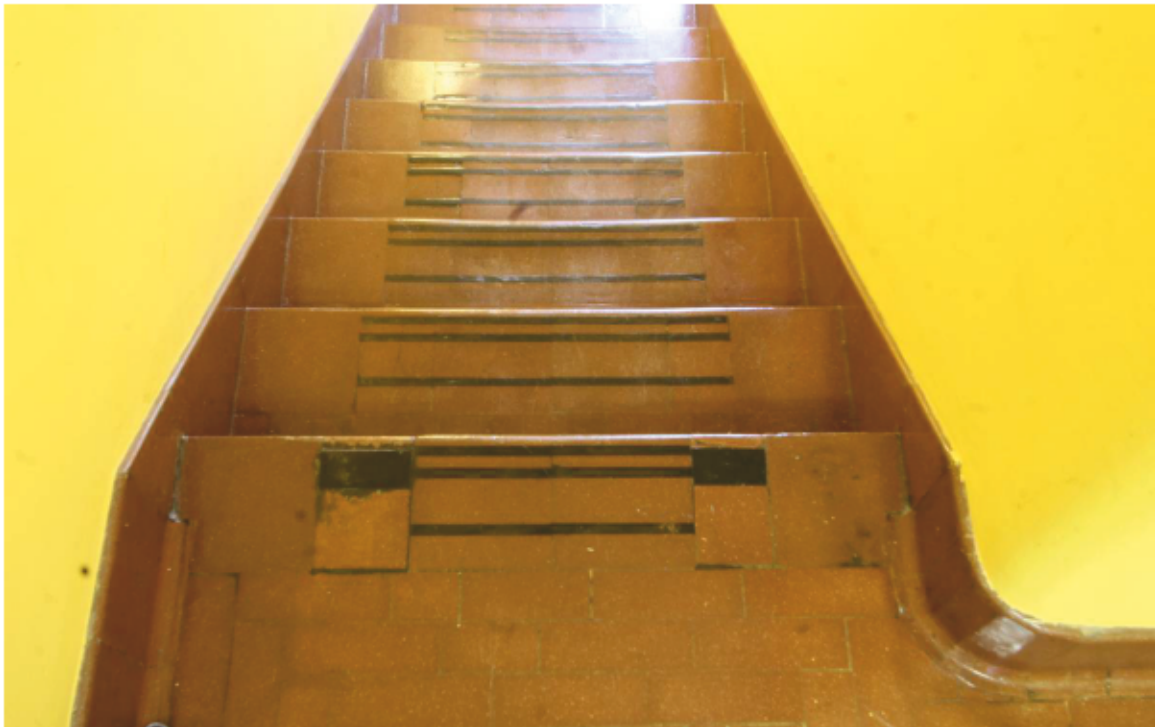
Plate 22 Detail of tiling to stair treads and landing
