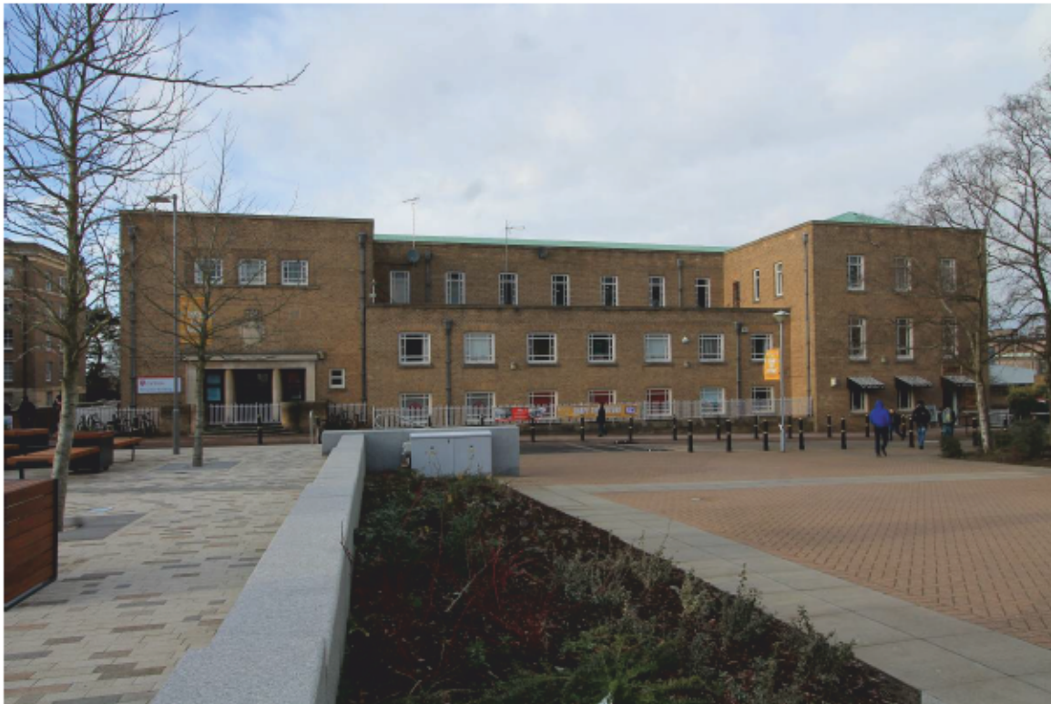
Plate 2 Percy Gee Building, East Wing viewed from the public realm to the east, looking north-west
