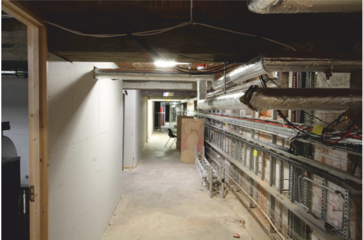
Plate 52 Basement corridor (LB3)
