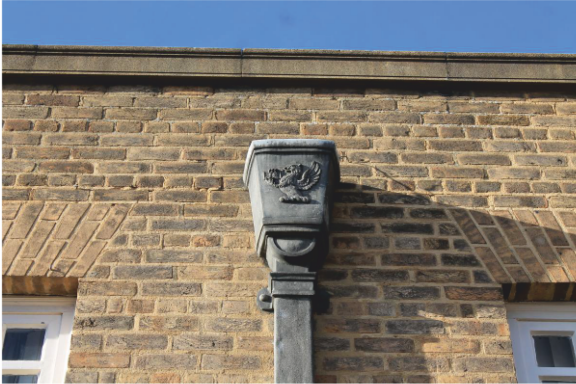
Plate 7 Percy Gee Building, Detail of rainwater hopper
