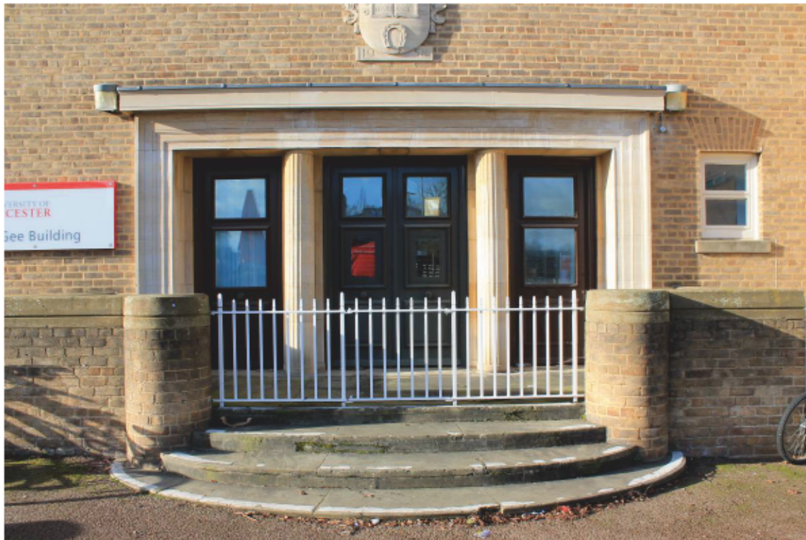
Plate 5 Percy Gee Building, East Wing, Former principal entrance
