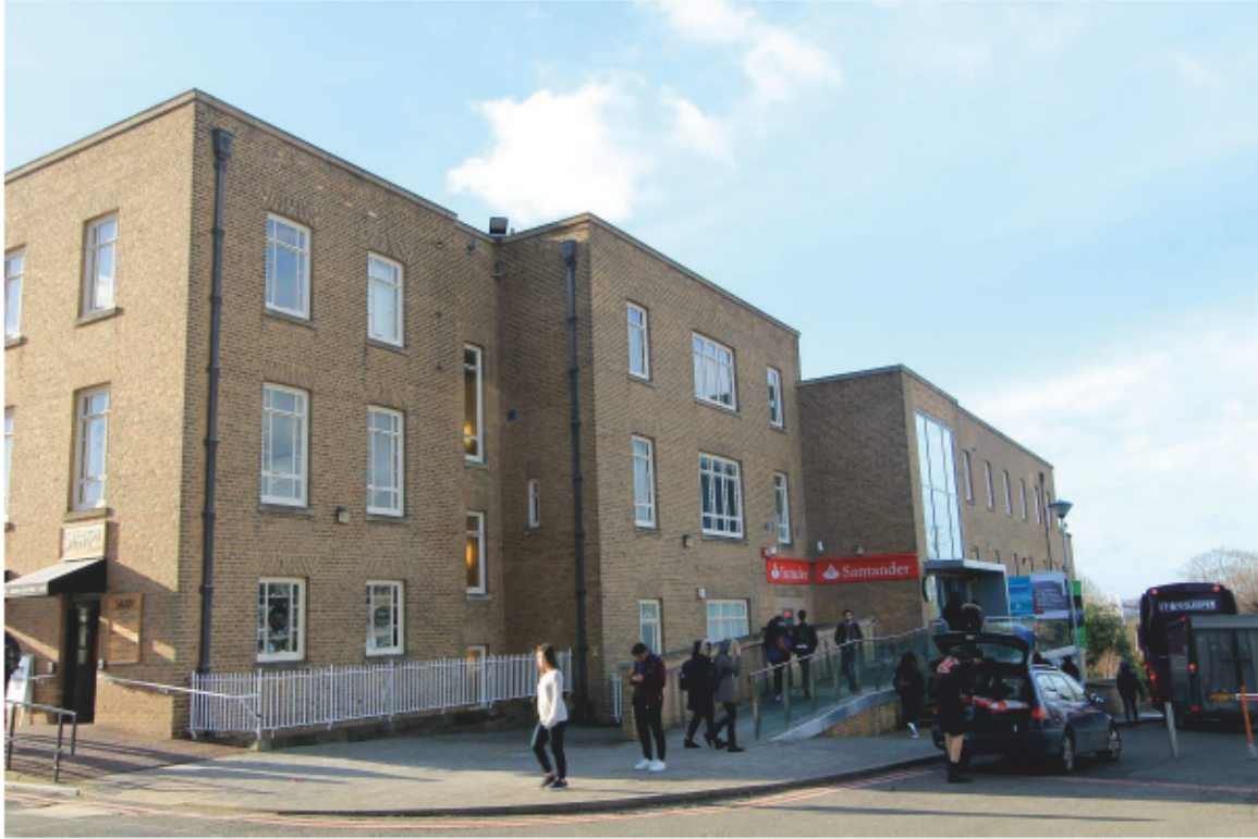
Plate 11 Percy Gee Building, east (left) and north elevations, looking south-west
