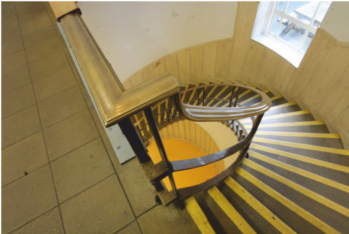
Plate 20 Stair (G3) down to upper basement
