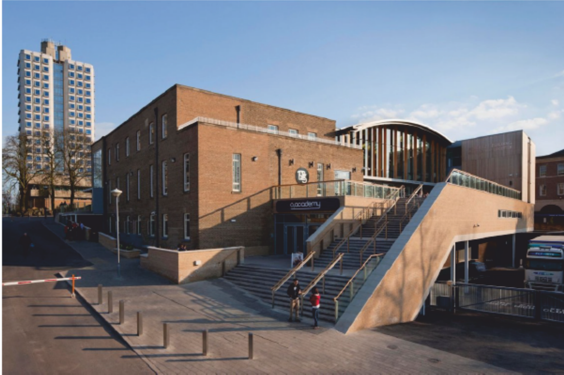
Plate 1 Percy Gee Building looking towards the north and remodelled west elevation (Shepherd Epstein Hunter)
