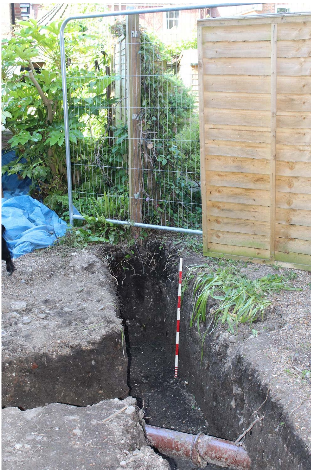
Plate 2: D3, View to South of foundation trench. Scale 1m.
