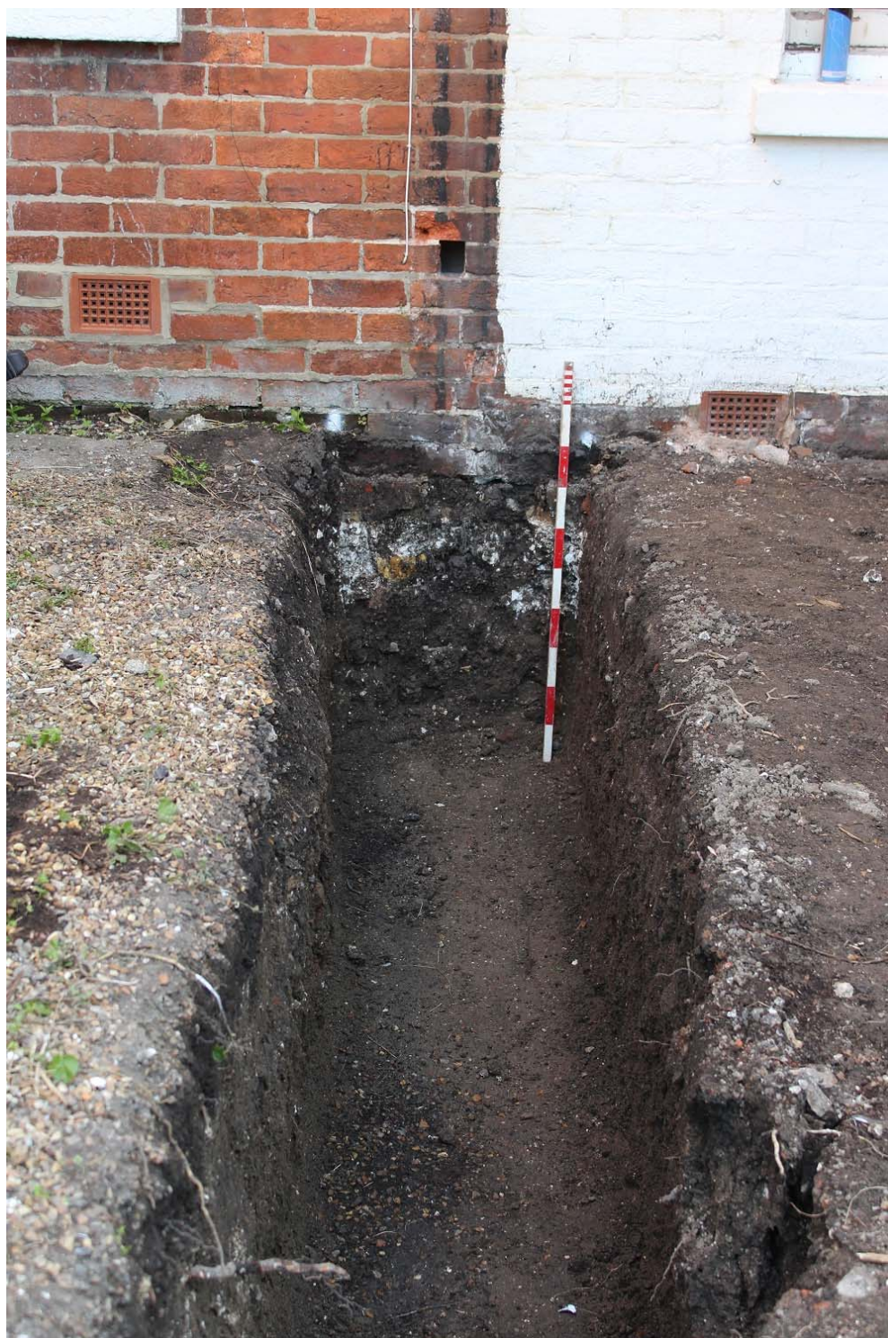
Plate 1: D1, View to North of new foundation trench. Scale 1m.
