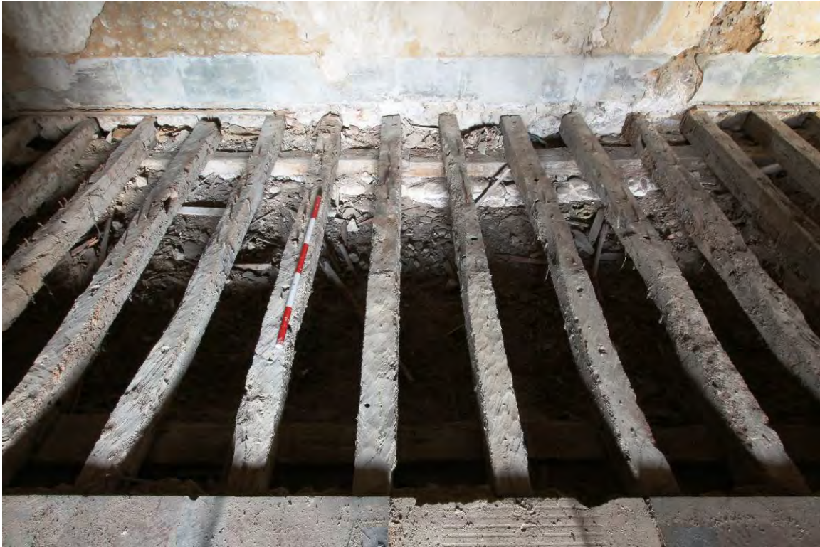
Plate 18 Floor section 1, central, joists 1:5-1:10
