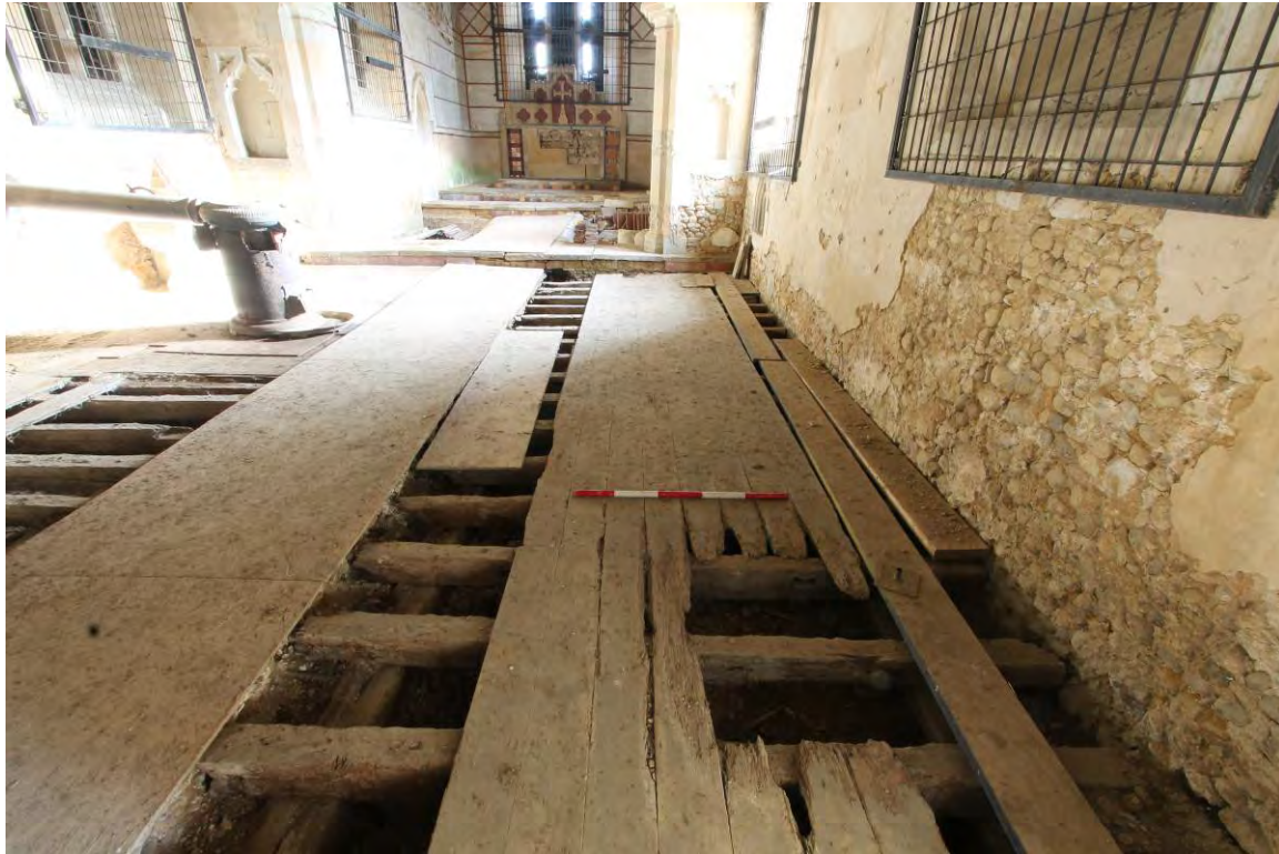
Plate 8 Extant floorboards to floor section (3), looking east (Pre-commencement)
