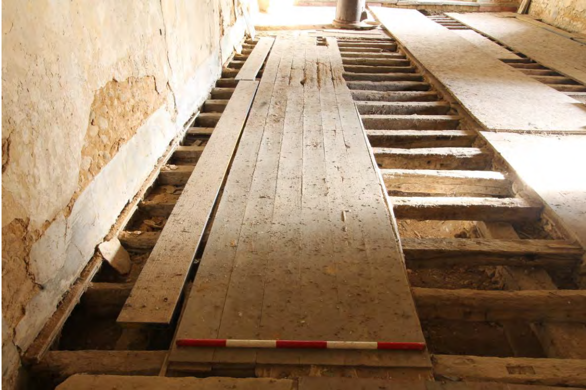
Plate 6 Extant floorboards to floor section (1), looking east (Pre-commencement)
