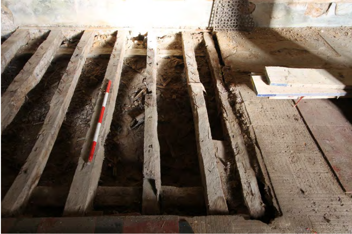
Plate 15 Floor section 1, east end, joists 1:14-1:18
