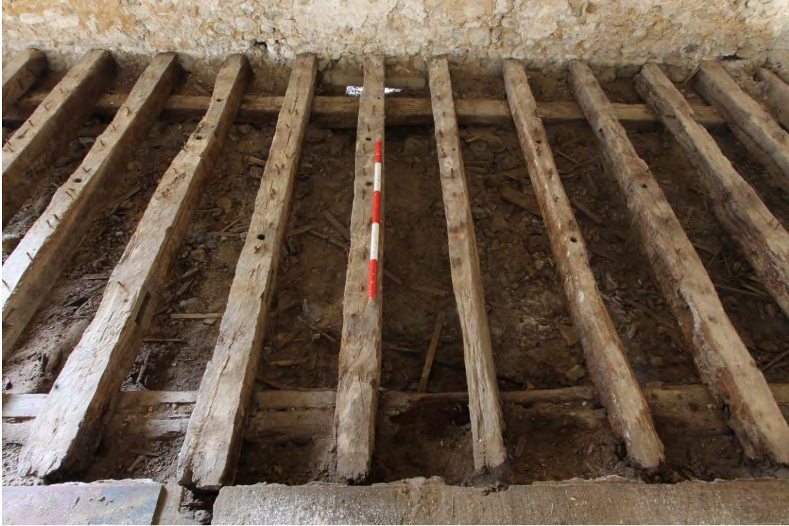
Plate 31 Floor section 3, joists 3:9-3:14
