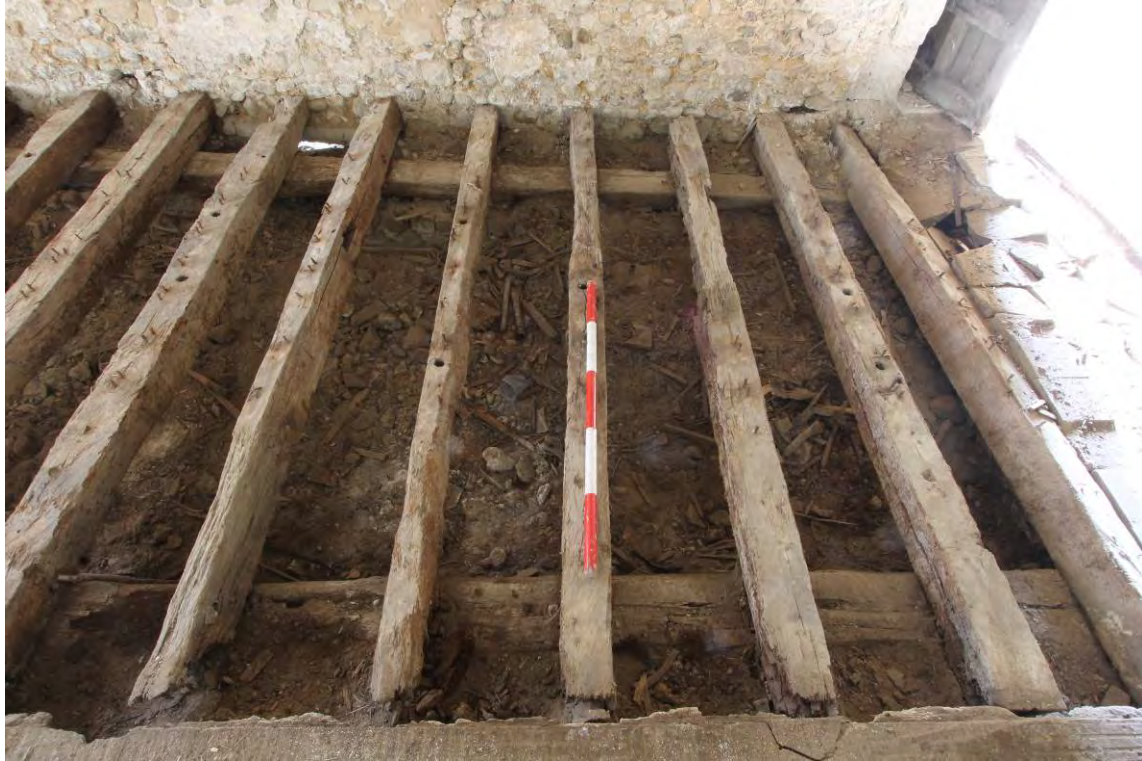
Plate 32 Floor section 3, joists 3:12-3:17
