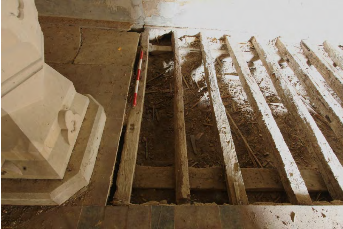
Plate 19 Floor section 1, west end, joists 1:1- 1:5
