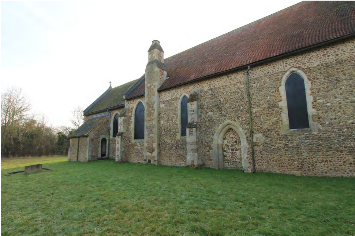
Plate 2 Northern elevations looking south-east
