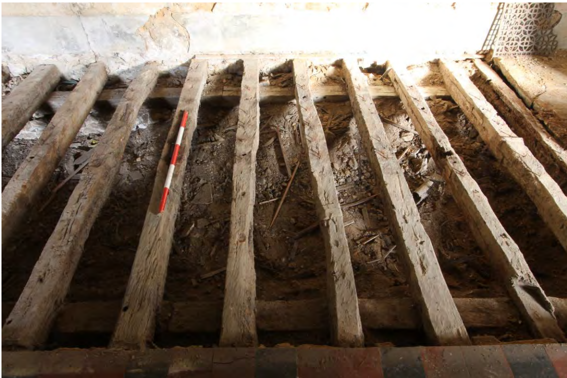
Plate 16 Floor section 1, east end, joists 1:15-1:11
