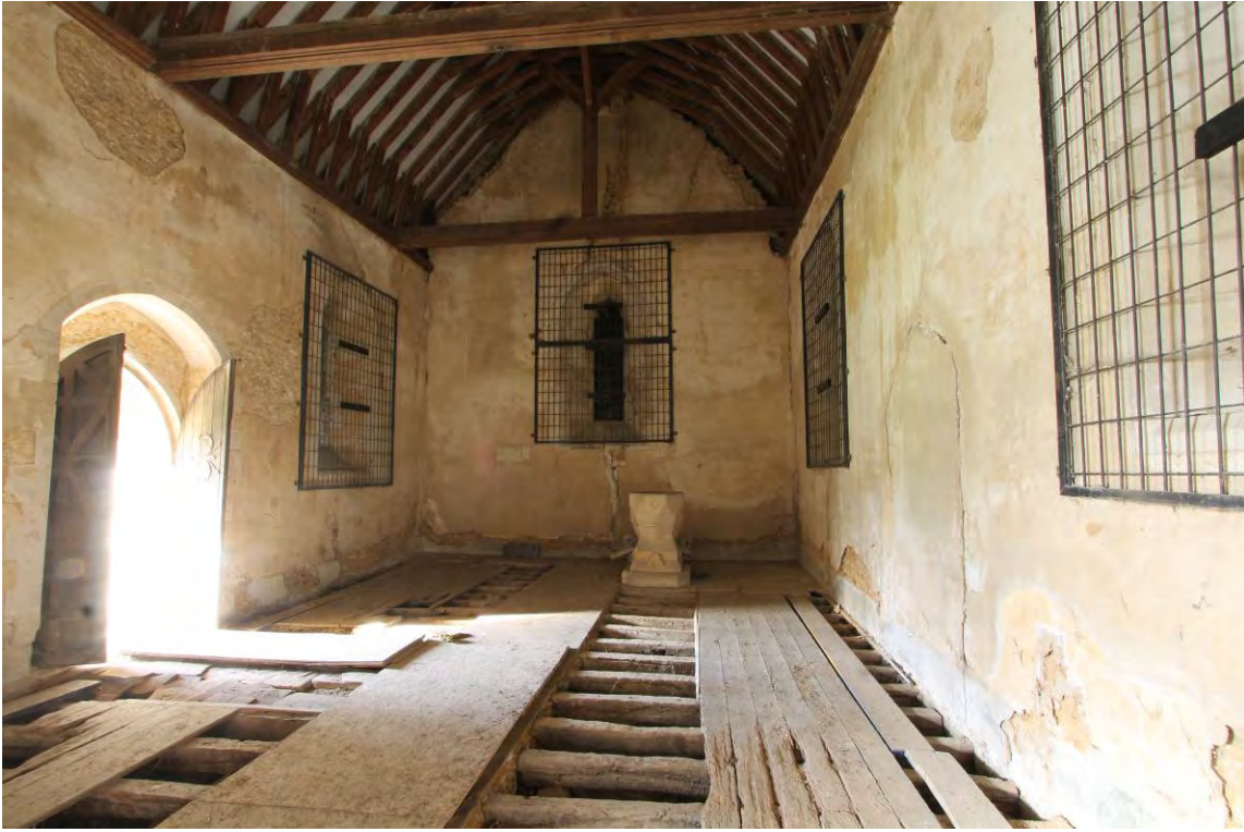
Plate 4 The nave looking west
