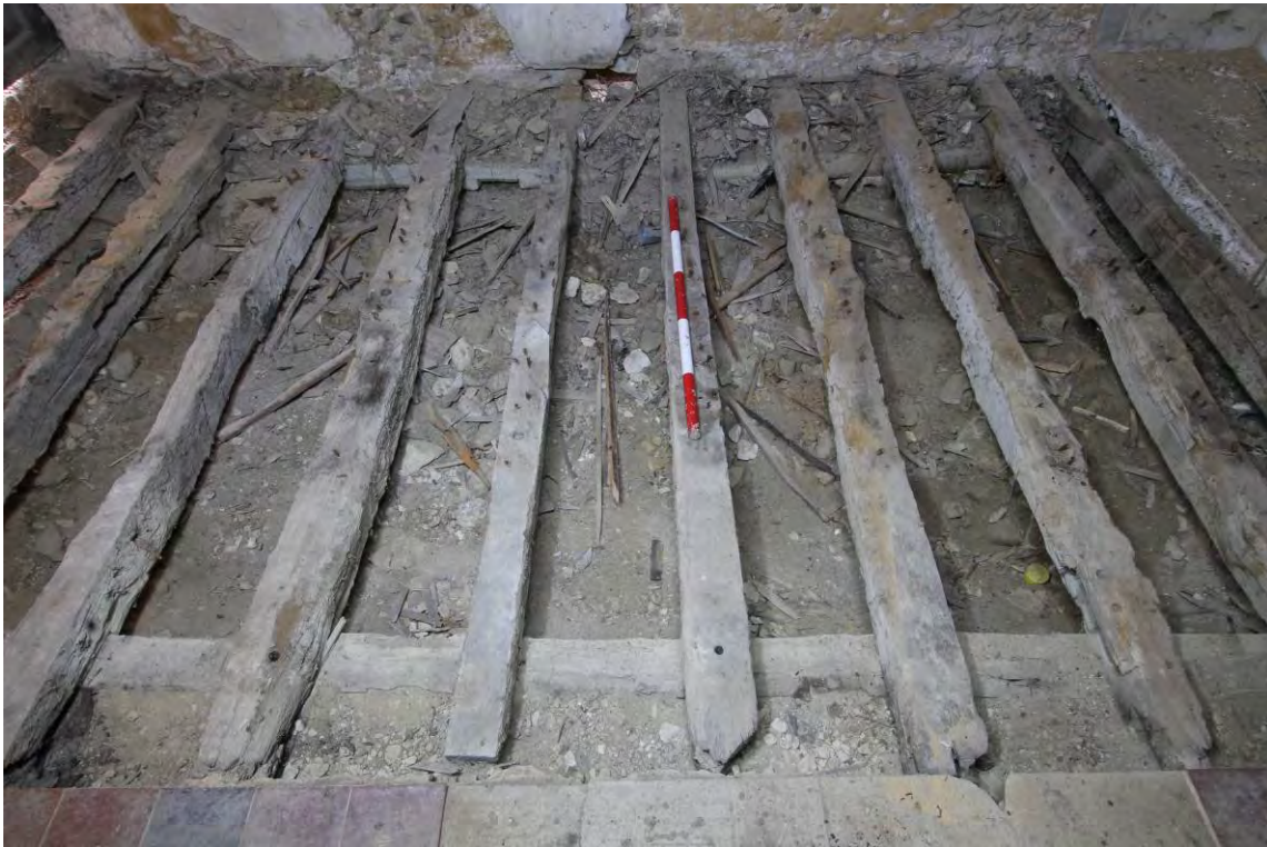
Plate 24 Floor section 2, joists 2:3-2:8
