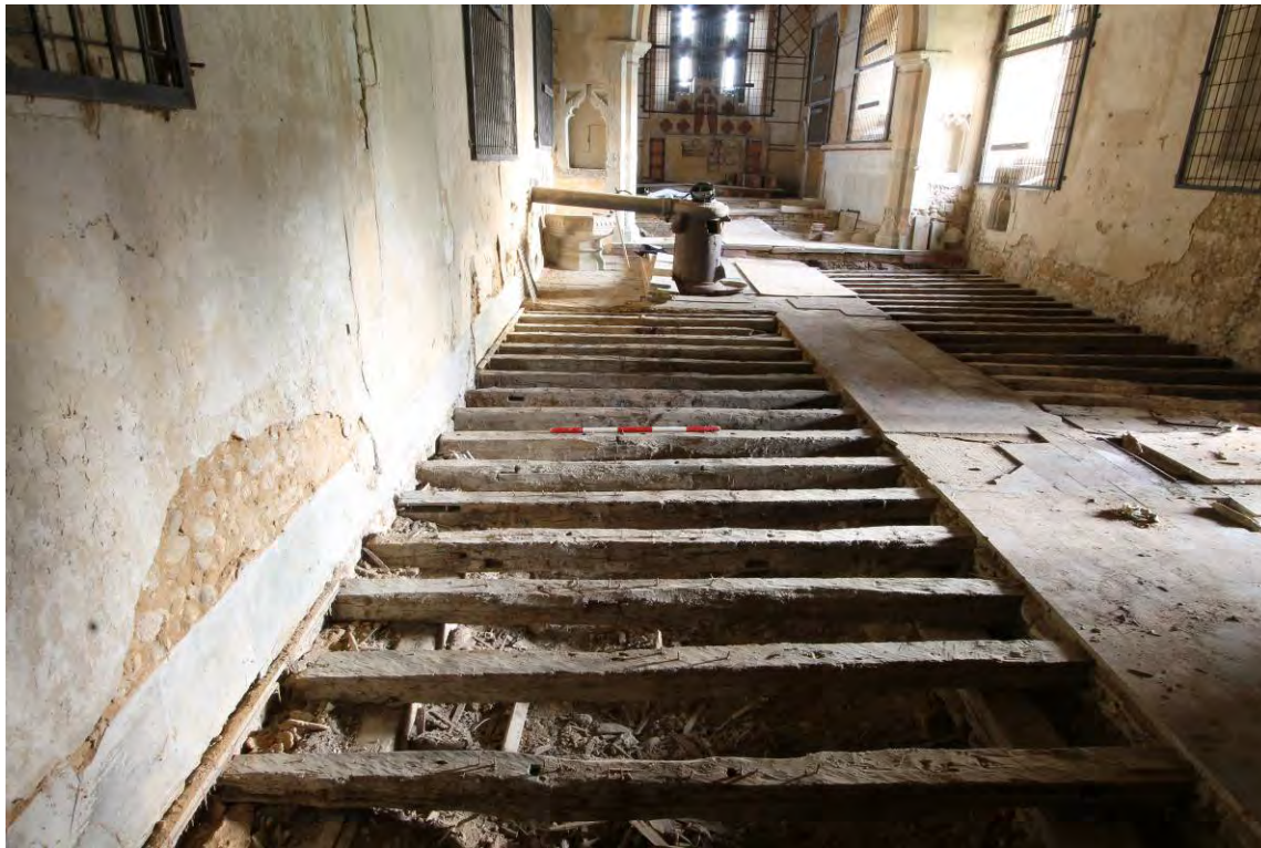
Plate 13 Nave, floor section (1) after the removal of boards, looking east
