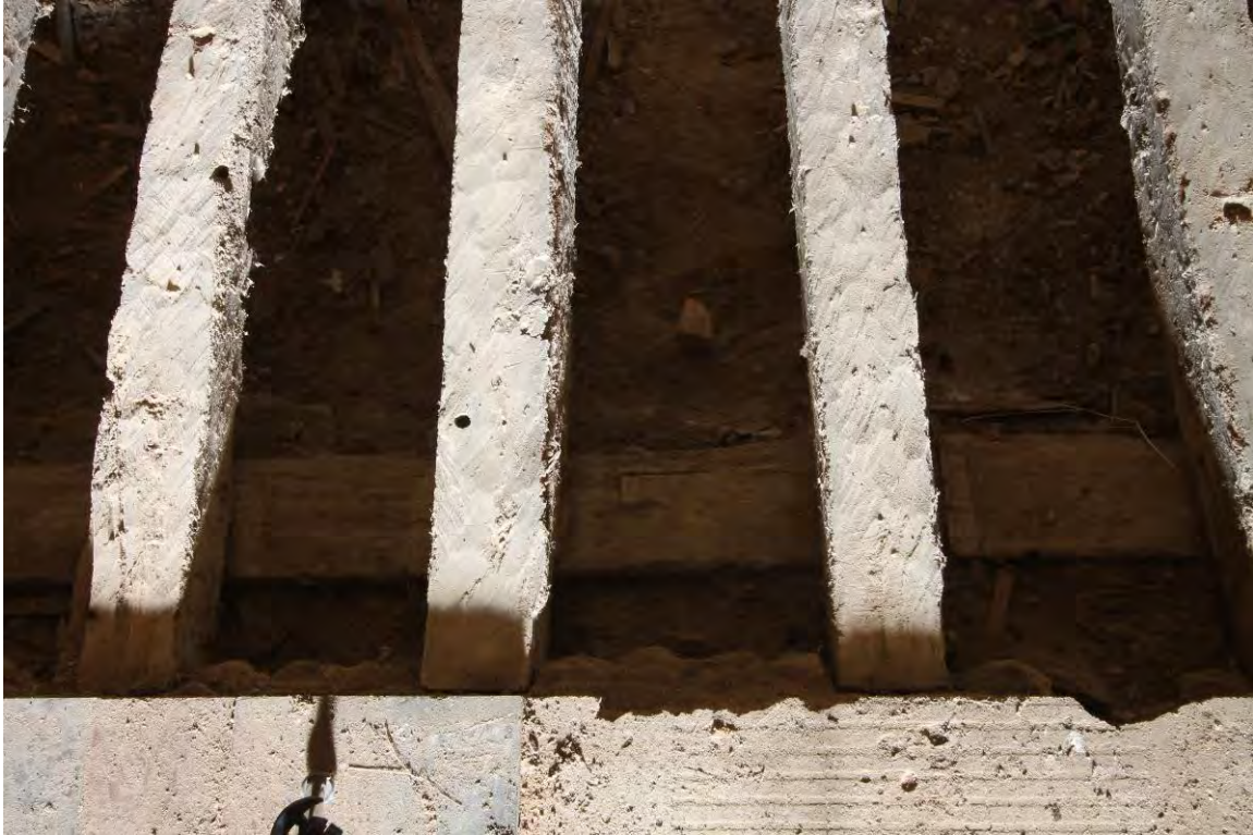
Plate 20 Floor section 1, detail of adze marks
