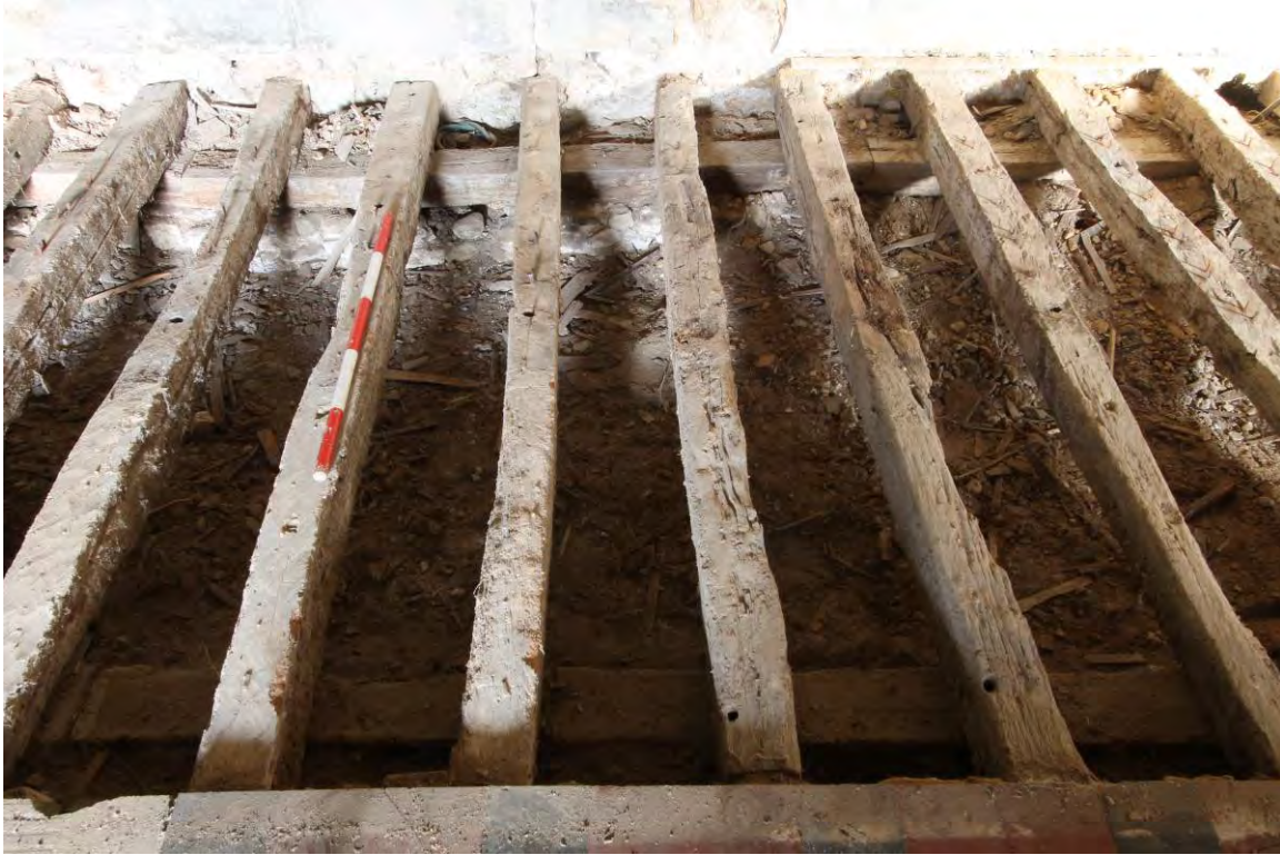
Plate 17 Floor section 1, central, joists 1:9-1:12
