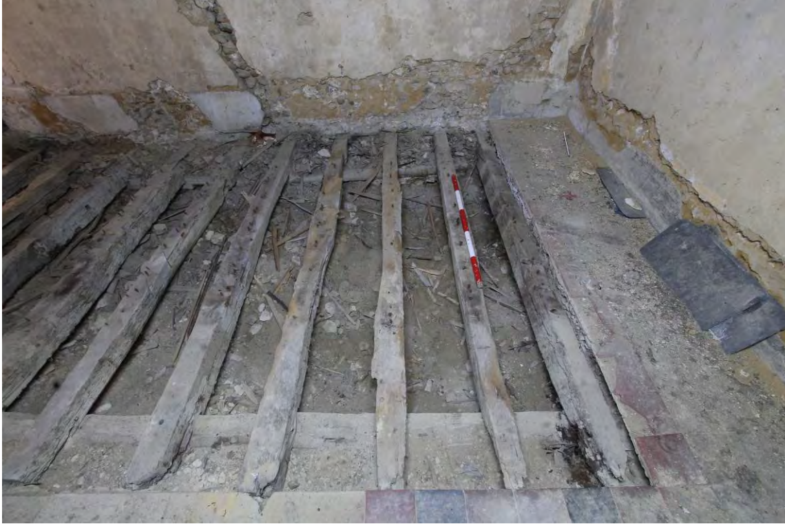
Plate 23 Floor section 2, west end, joists 2:1-2:6
