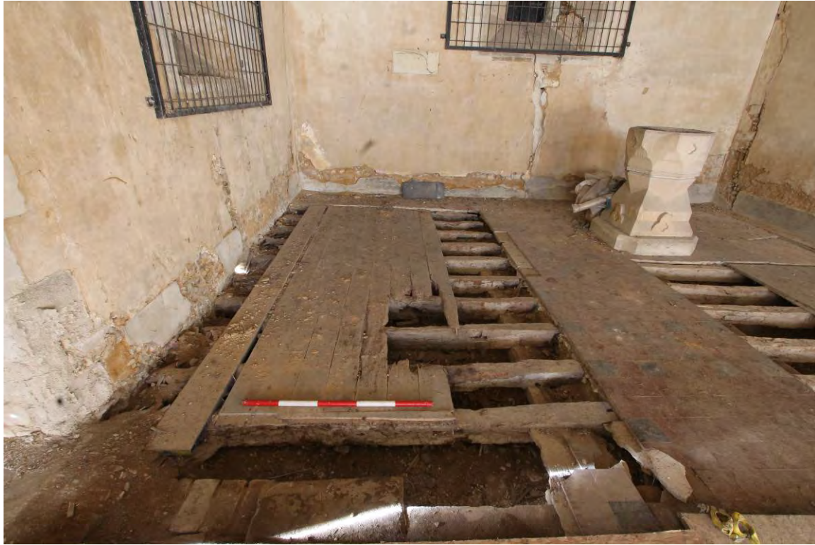
Plate 7 Extant floorboards to floor section (2), looking west (Pre-commencement)
