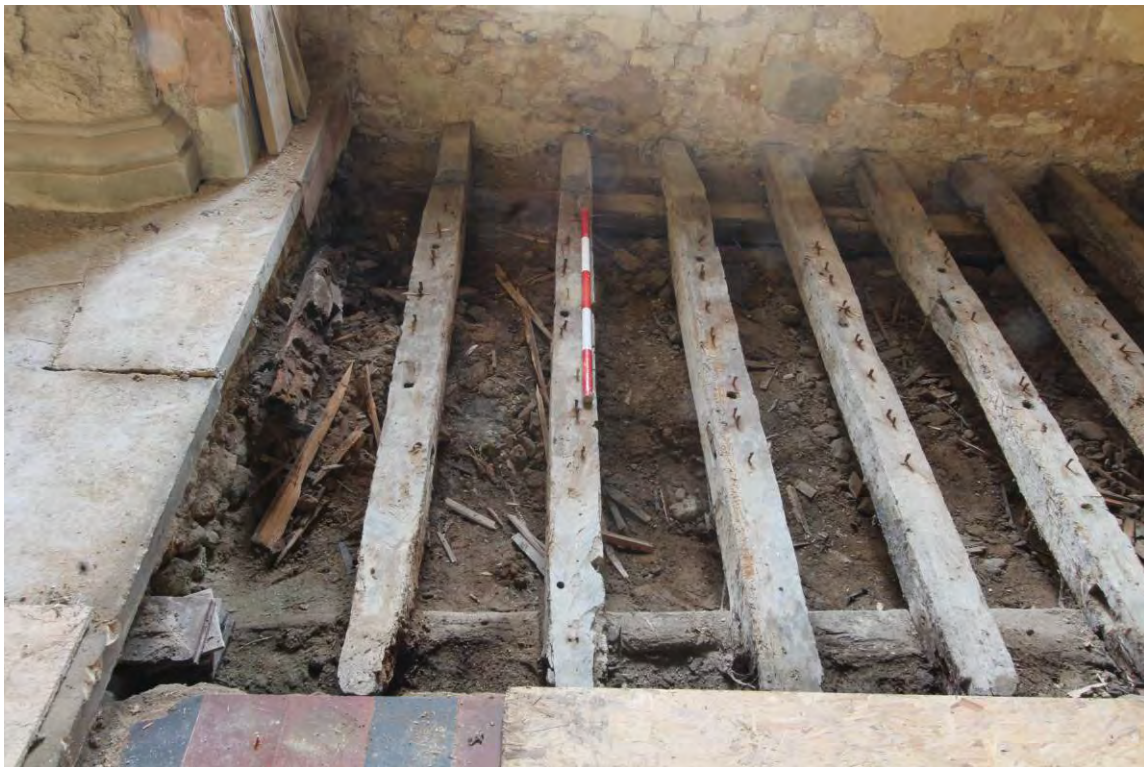
Plate 28 Floor section 3, east end, joists 3:1-3:4
