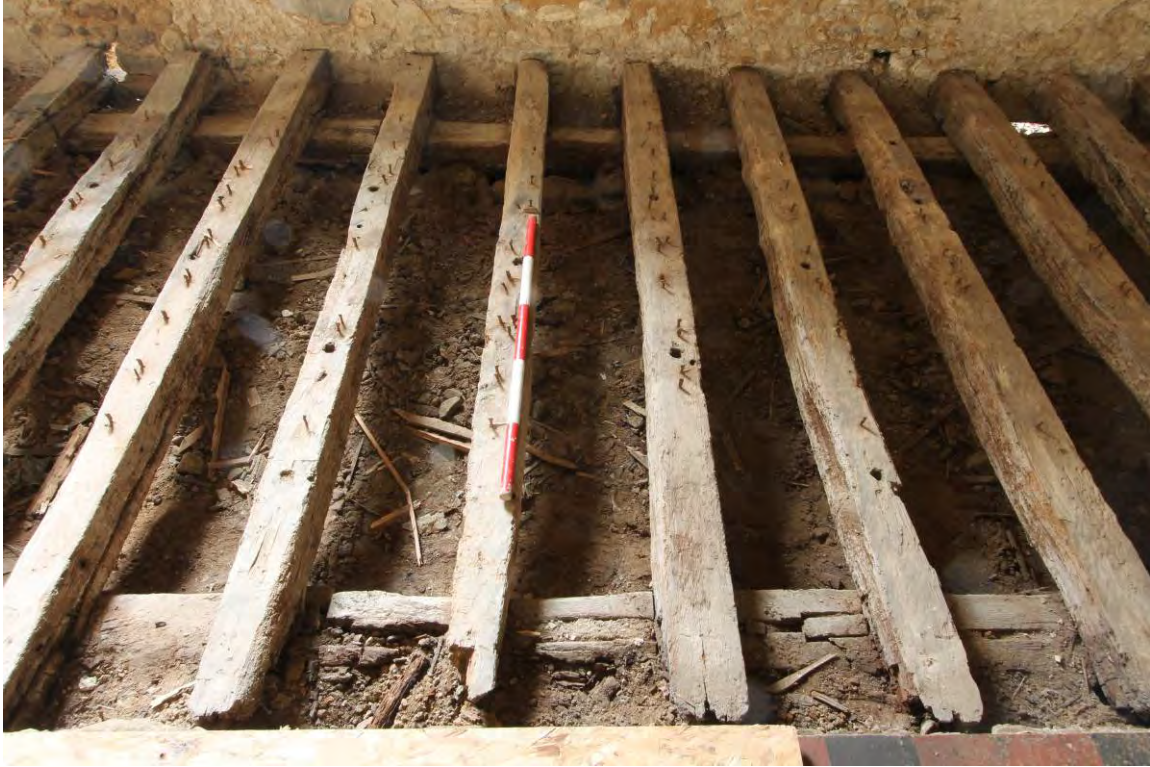
Plate 29 Floor section 3, joists 3:5-3:8
