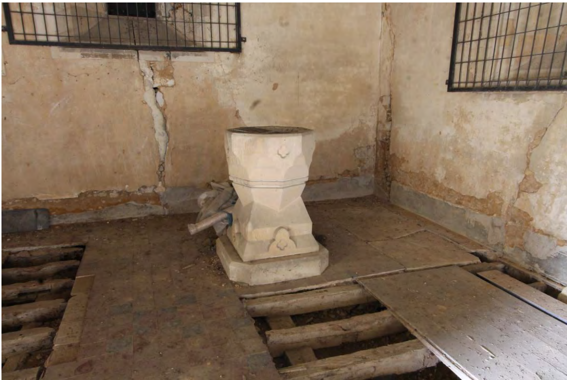
Plate 10 Quarry tile floor to central aisle and around font
