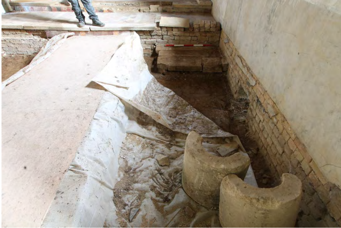
Plate 37 Floor void, chancel, south side
