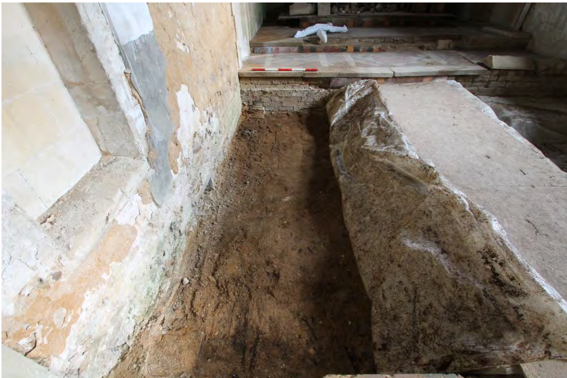
Plate 36 Floor void, chancel, north side
