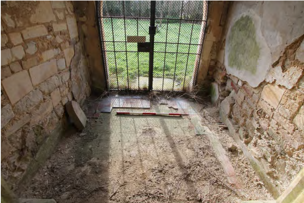
Plate 34 Remains of quarry tiles in south porch
