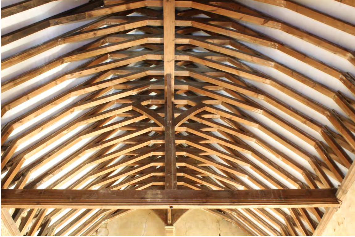
Plate 5 Detail of later 19 th century crown post roof over nave
