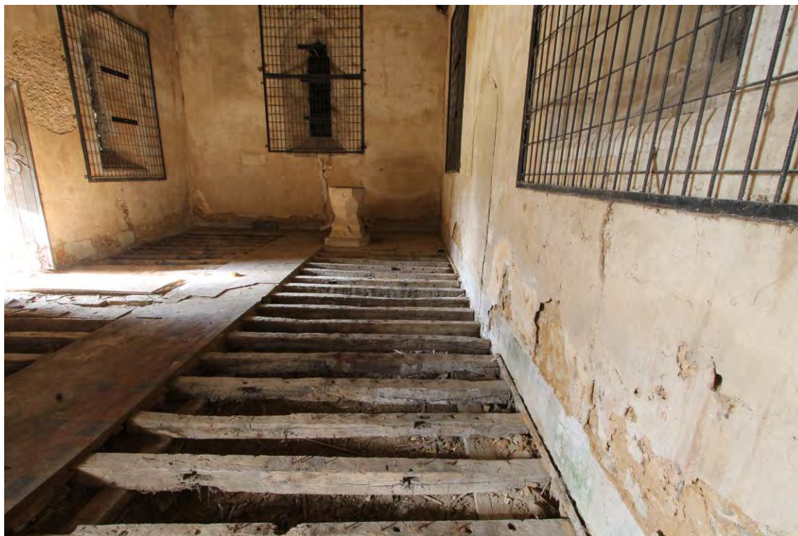
Plate 14 Nave, floor section (1) after the removal of boards, looking west
