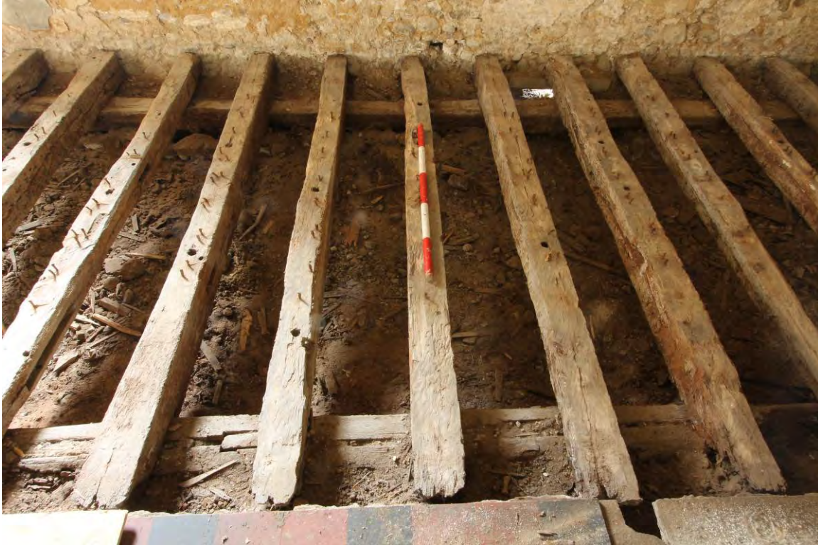
Plate 30 Floor section 3, joists 3:7-3:11
