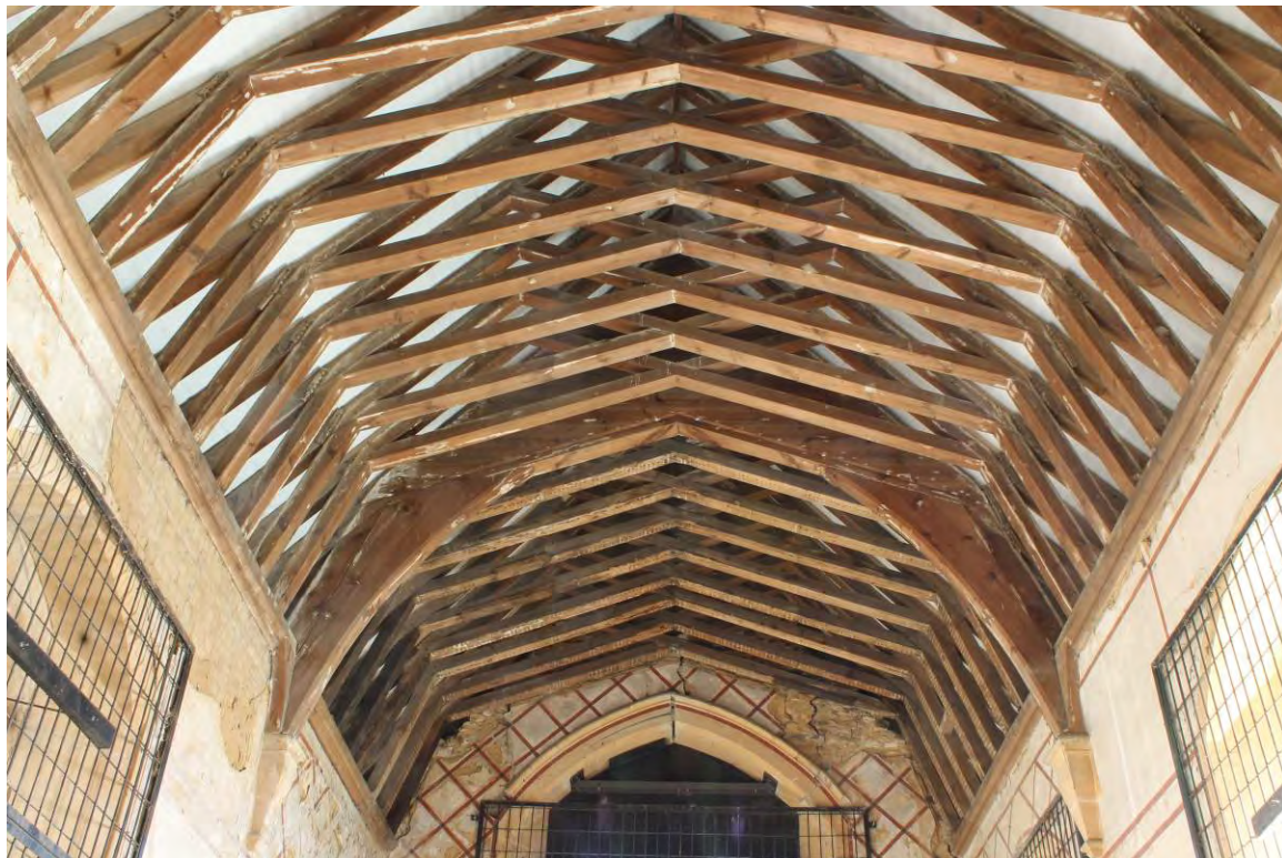
Plate 38 Replacement 19th century chancel roof
