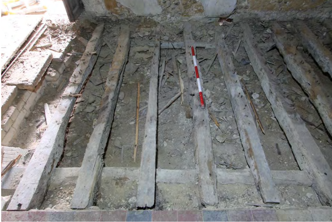
Plate 25 Floor section 2, joists 2:6-2:10
