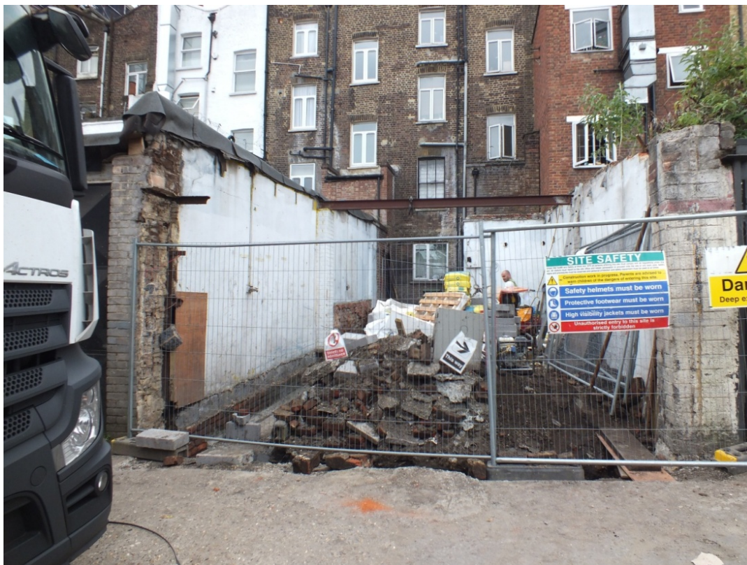
Plate 3: Site, looking south (NCS17 D1 (2))
