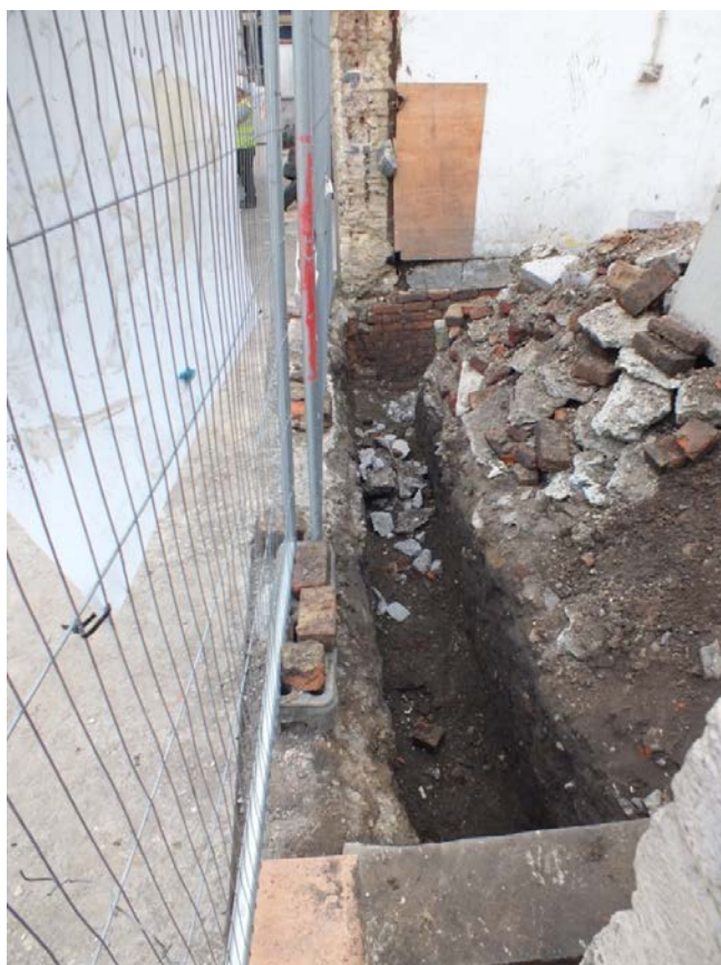
Plate 4: Northernmost foundation trench, looking east (NCS17 D1 (3))
