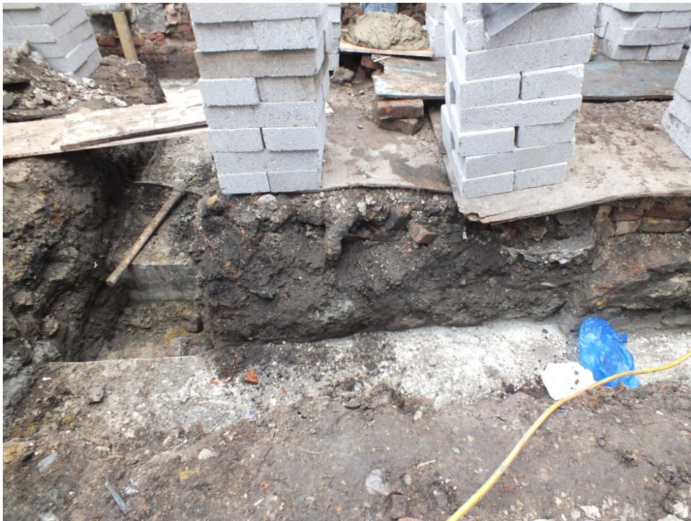
Plate 9: West end of the southernmost foundation trench, looking north (NCS17 D1 (9))
