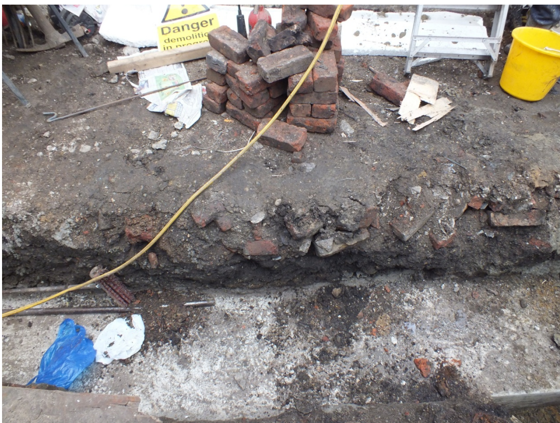
Plate 10: Southernmost foundation trench, looking south (NCS17 D1 (11))
