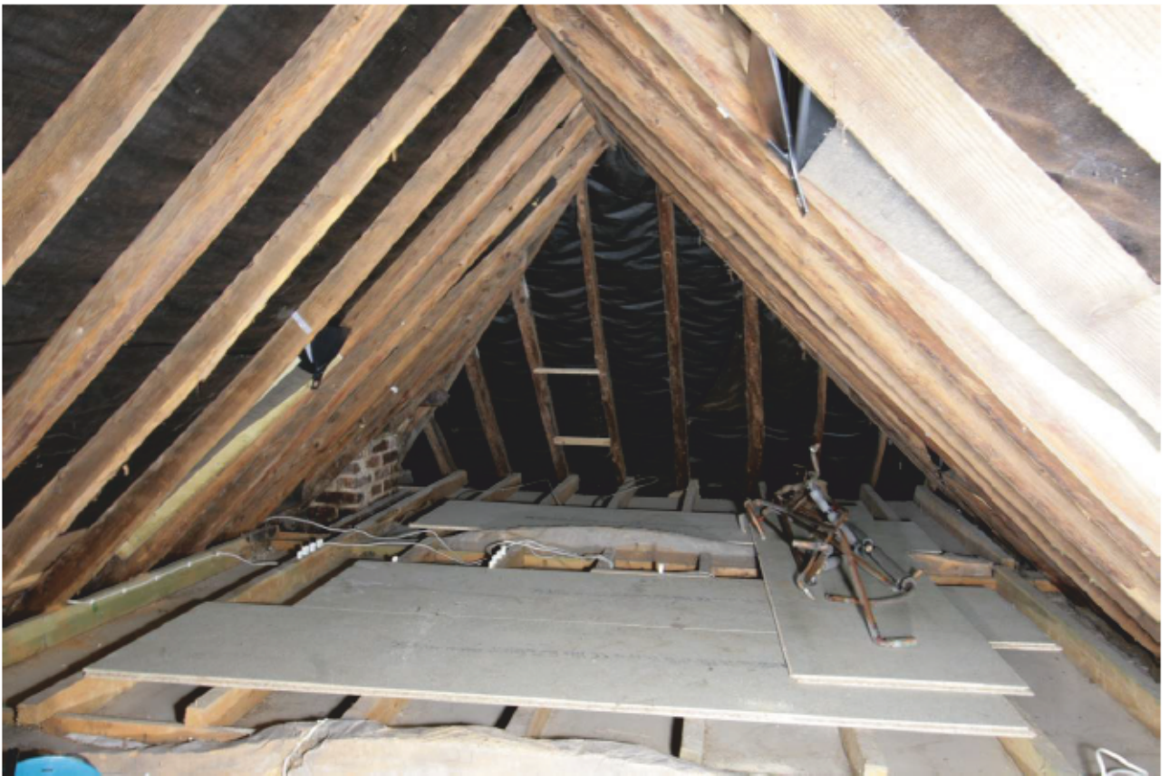
Plate 62: Roof space over Bedroom 2, looking west (D3 027)
