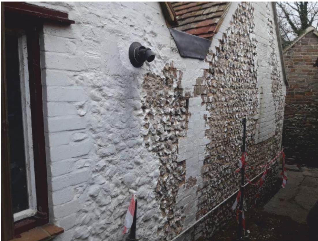
Plate 6: Side (west) elevations of the Old Bakery, looking south-east (photograph provided by George Roberts)
