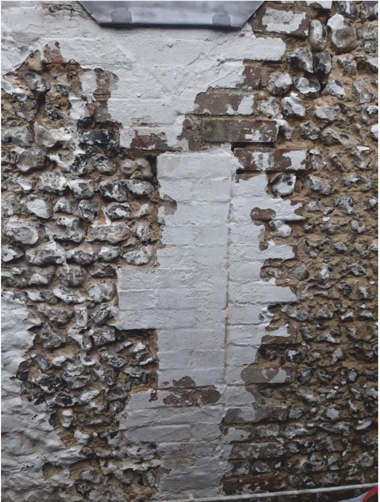
Plate 7: West elevation showing straight joint between Utility Room and Kitchen, looking east (photograph provided by George Roberts)
