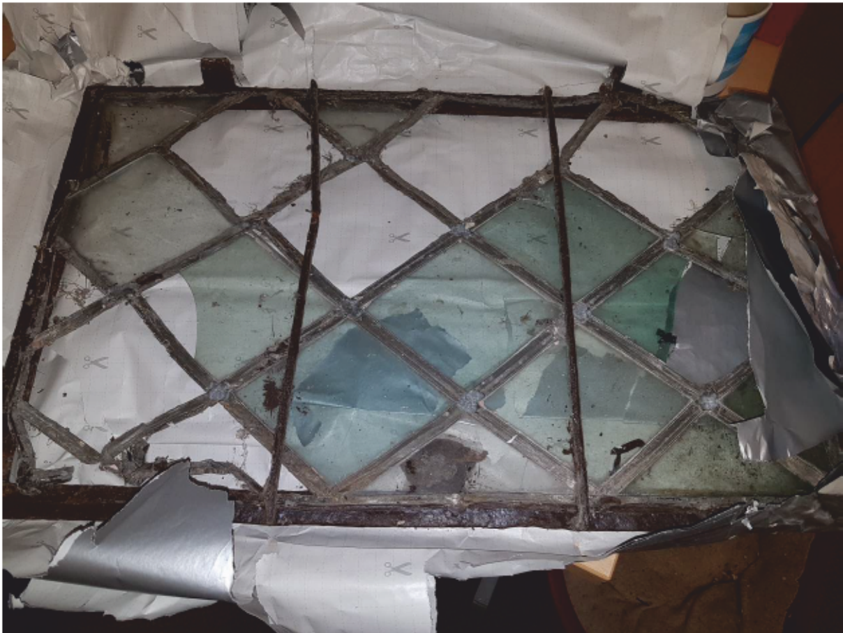
Plate 18: 17 th century window after removal from south wall of Sitting Room for conservation (photograph provided by George Roberts)
