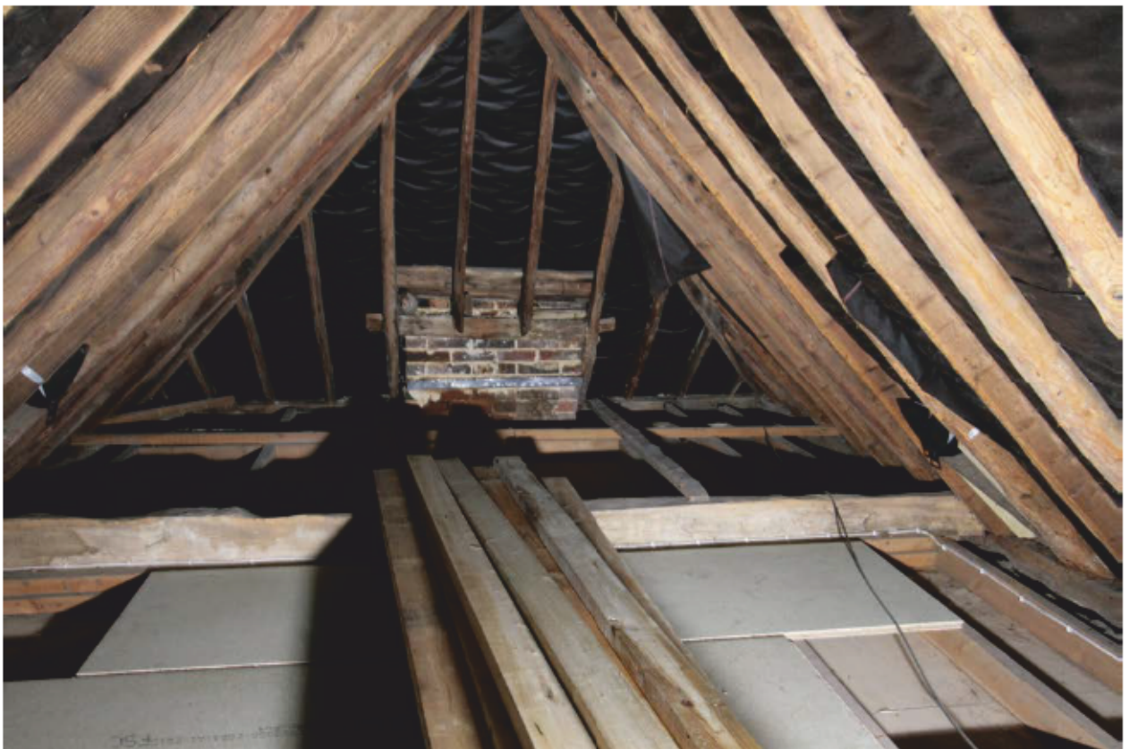
Plate 60: Roof space over Bedroom 1, looking east (D3 024)
