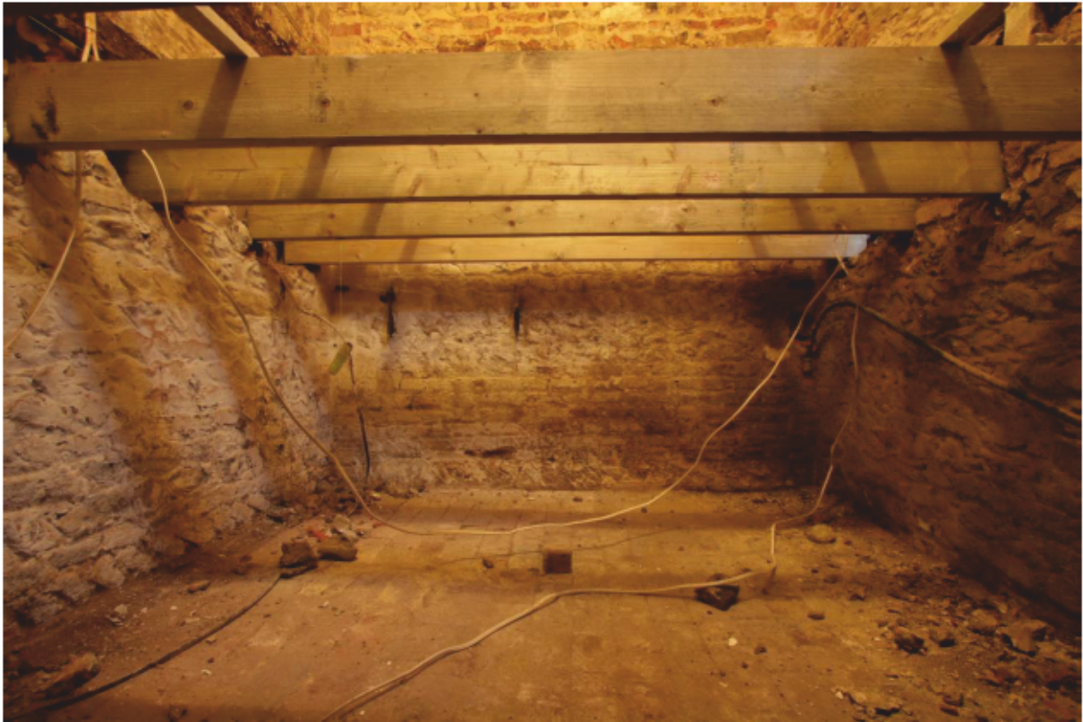
Plate 33: Cellar below Study, looking east (D1 012)
