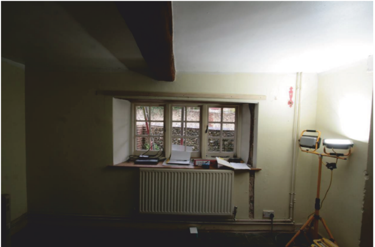
Plate 16: North wall of Sitting Room, looking north (D2 022)
