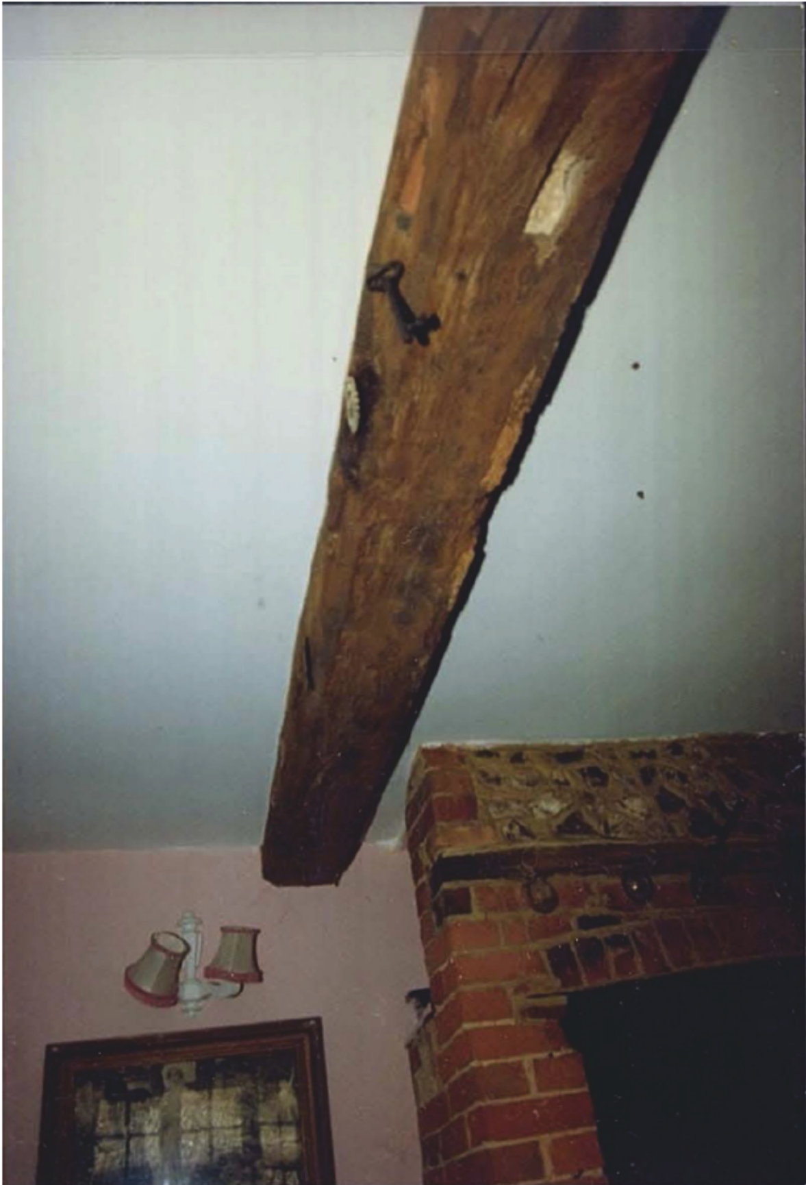
Historic Plate 17 Photograph taken by Sara Squires in September 1991 of the chamfered beam in the Sitting Room of Old Bakery, looking south (© National Trust Wisley)
