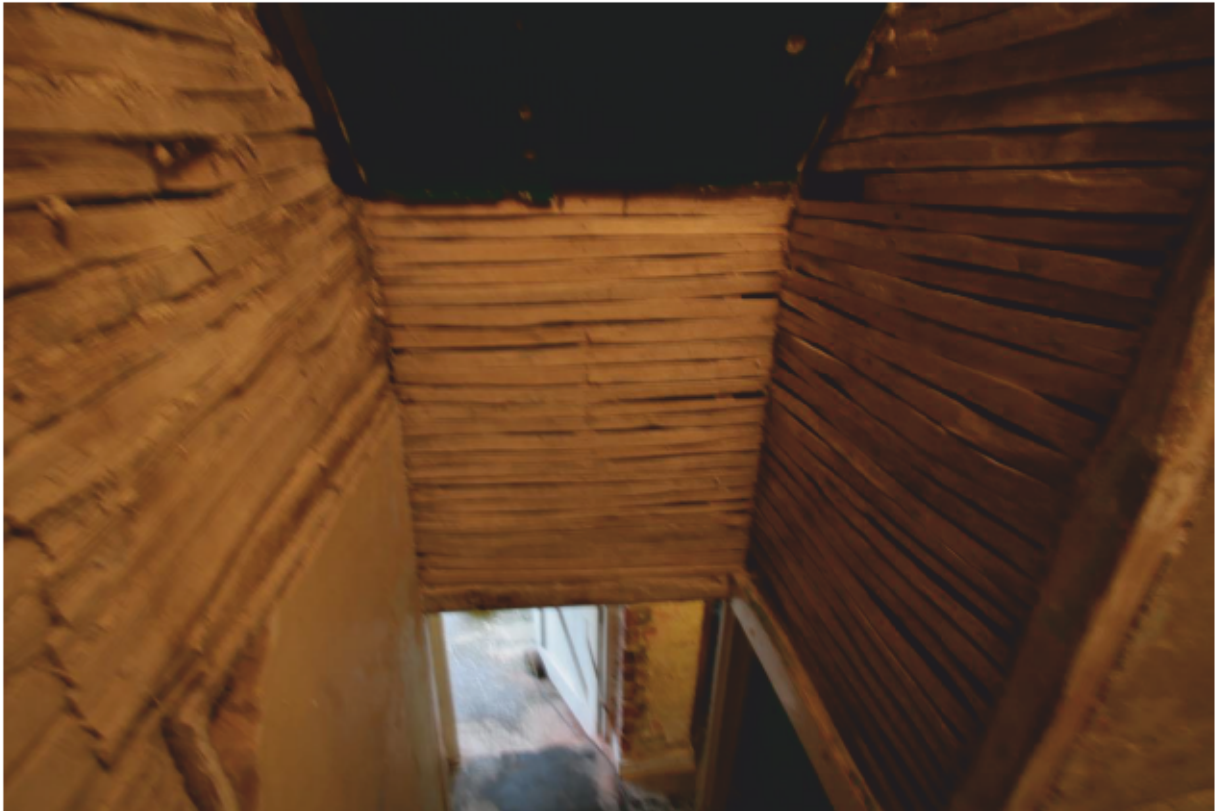
Plate 38: Stairwell, looking south (D1 027)
