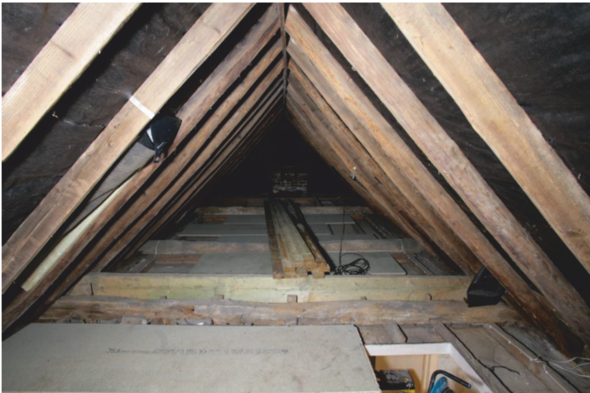
Plate 58: Roof space over Bedrooms 1 and 3, looking east (D3 022)
