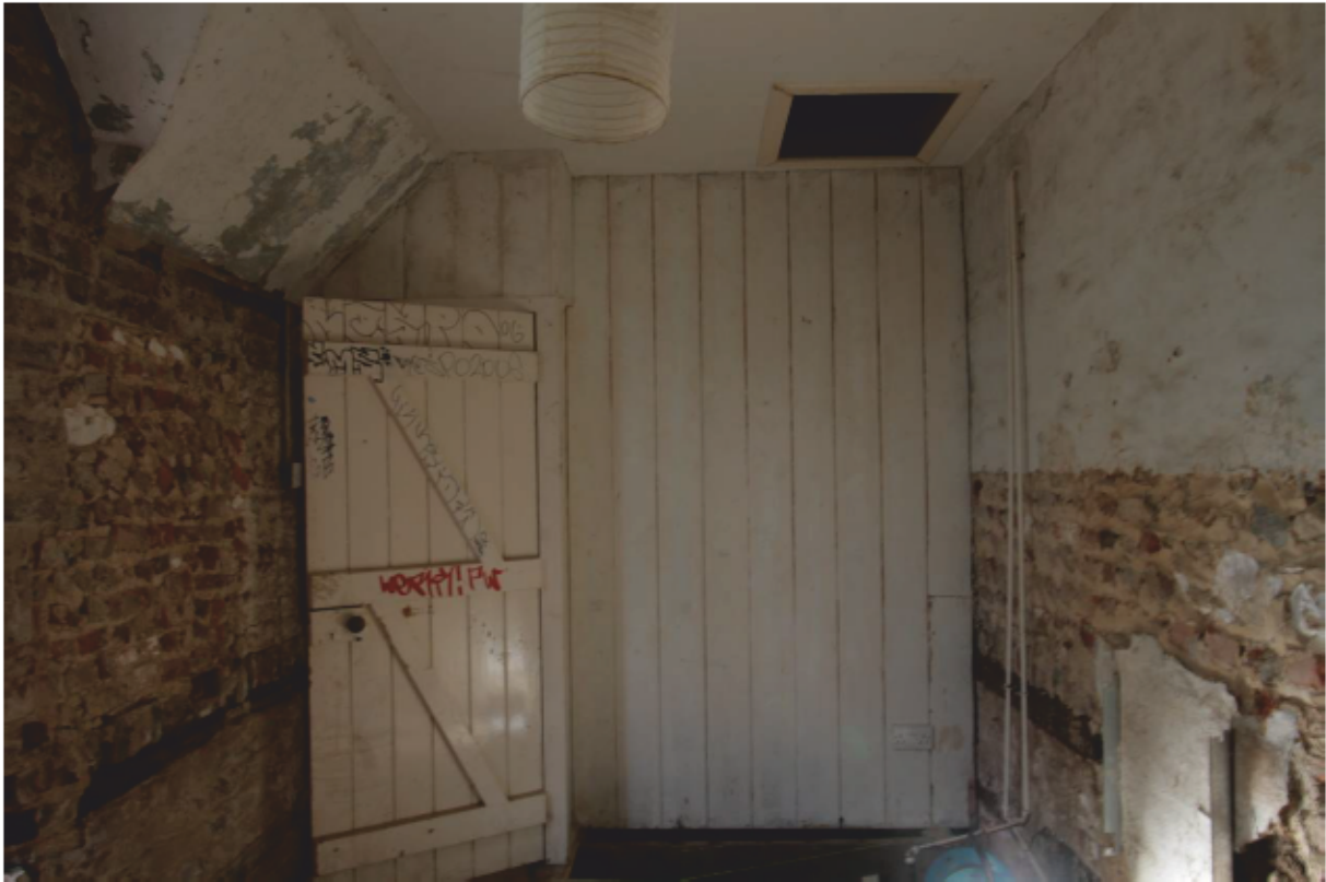
Plate 29: West wall of the Study, looking west (D1 003)
