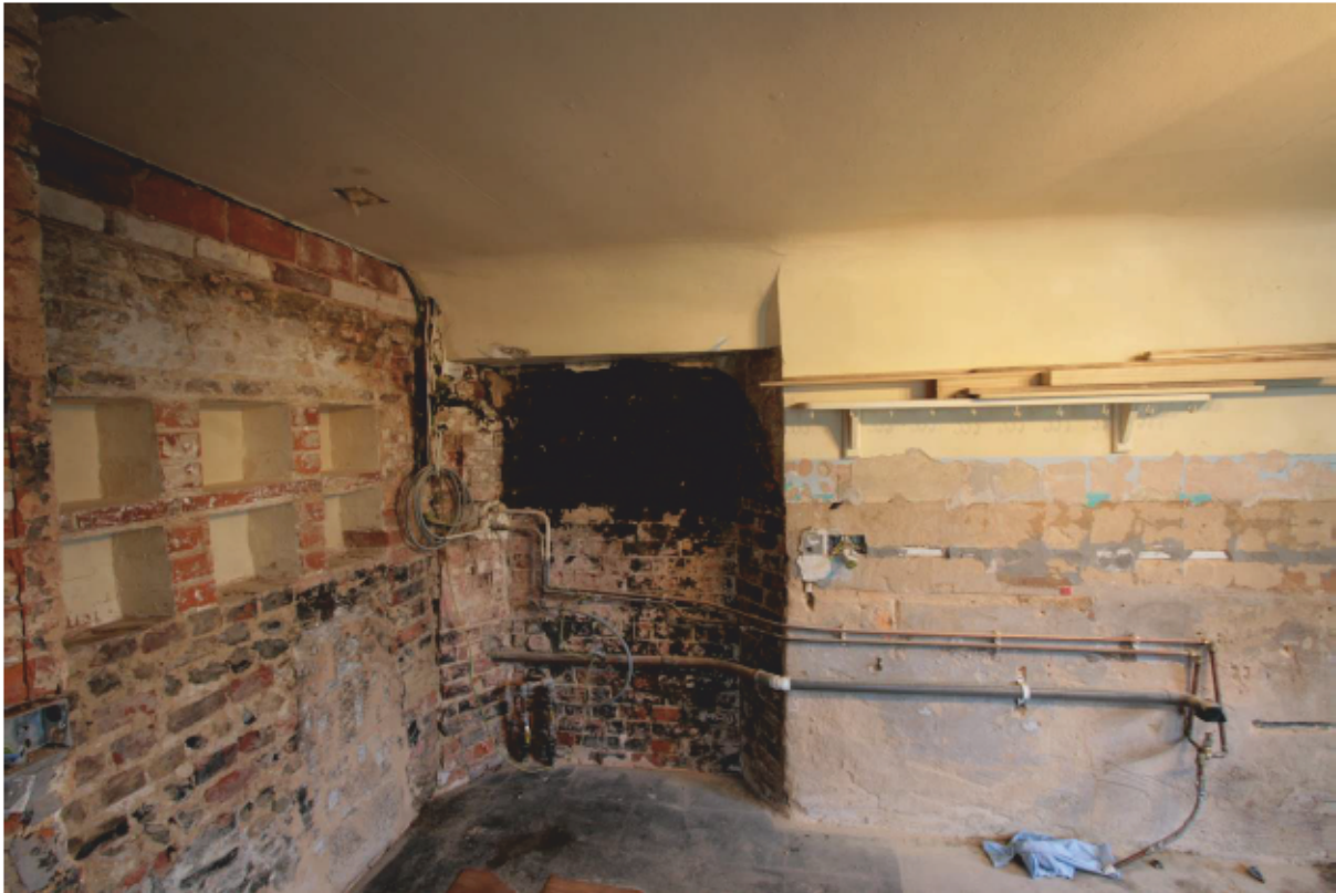
Plate 69: West side of north wall of Kitchen, looking north (D3 012)
