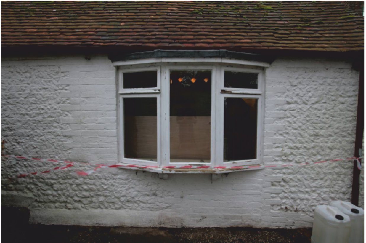
Plate 12: South elevation of the Kitchen, looking north (D3 004)
