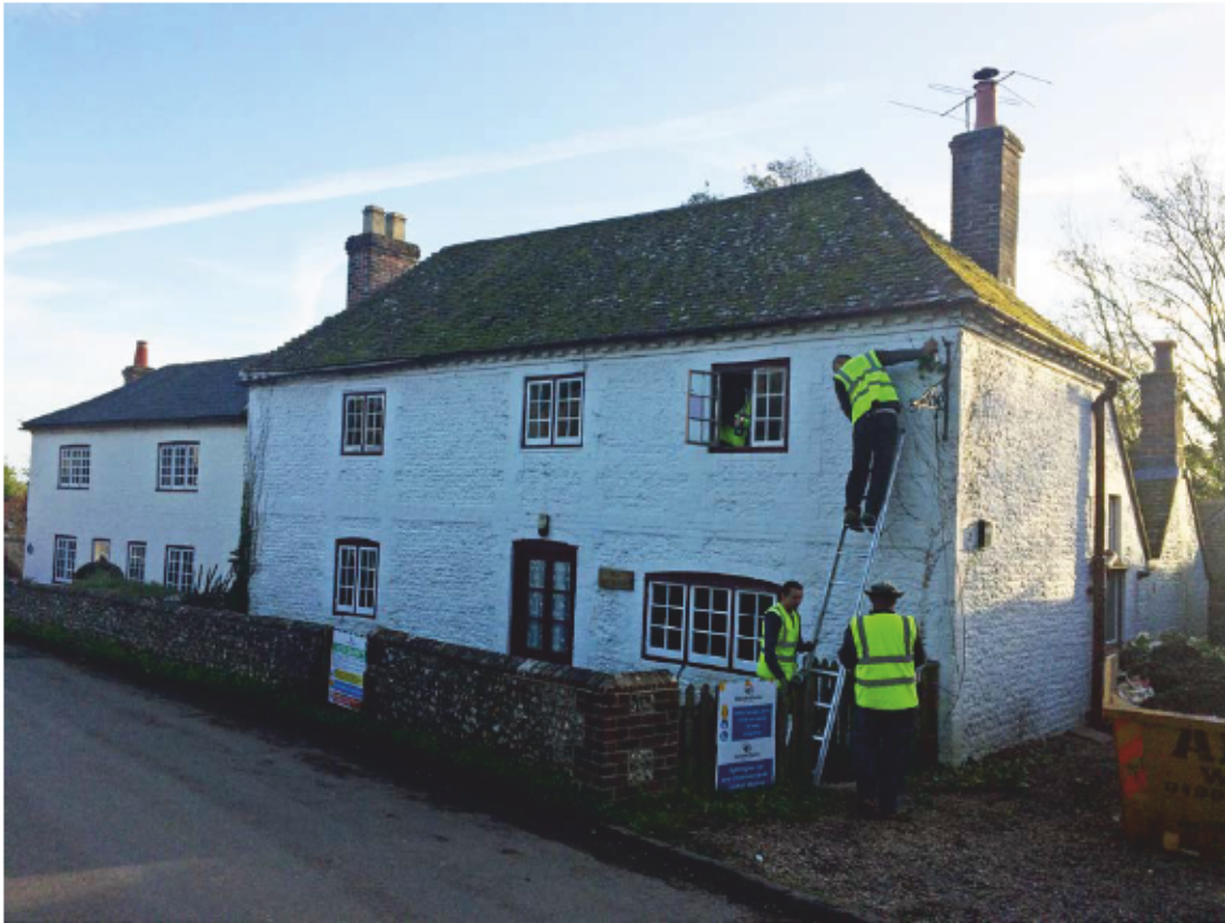
Plate 1: Front (north) and side (west) elevations of the Old Bakery, looking south-east (photograph provided by George Roberts)
