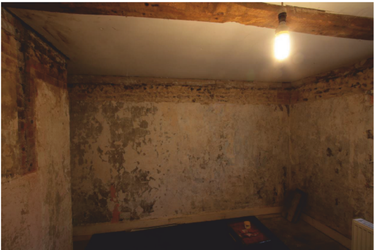
Plate 50: Bedroom 2, looking west (D2 010)
