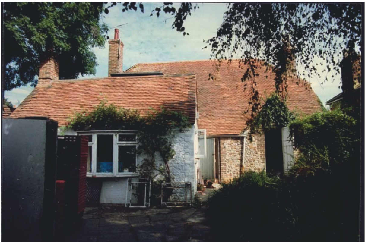
Historic Plate 10 Photograph taken by Sara Squires in September 1991 of the former bakehouse (now Kitchen) extension at the Old Bakery, looking north (© National Trust Wisley)
