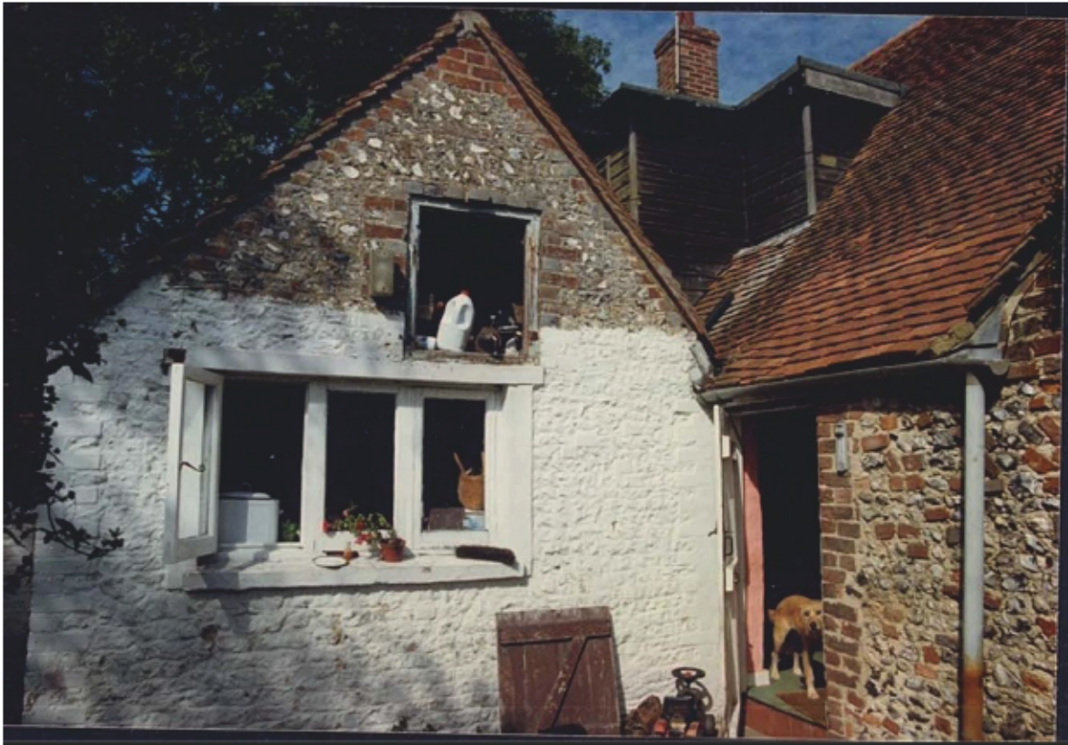
Historic Plate 11 Photograph taken by Sara Squires in September 1991 of the former bakehouse (now Kitchen) extension at the Old Bakery, looking east (© National Trust Wisley)
