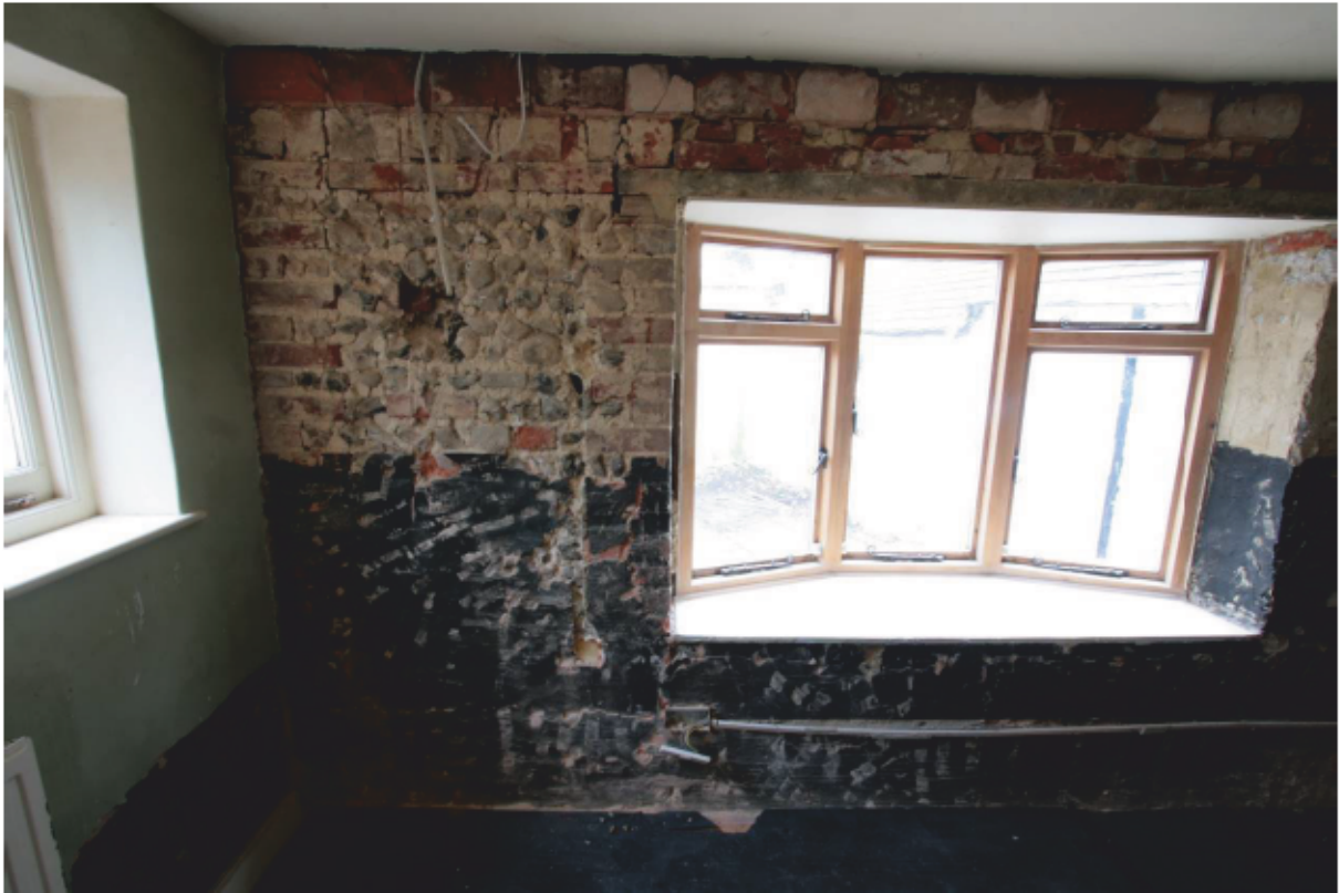
Plate 65: East side of south wall of Kitchen, looking south (D3 018)
