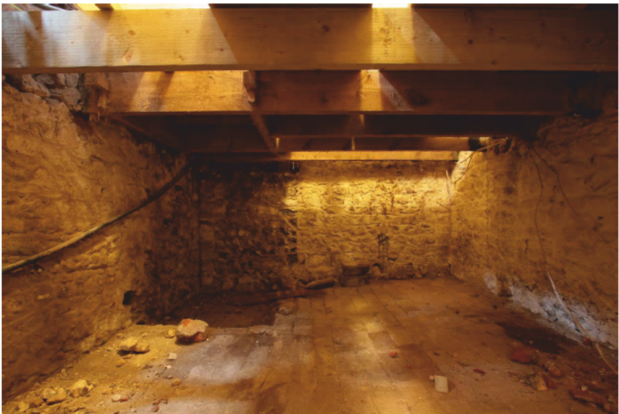
Plate 34: Cellar below Study, looking west (D1 013)
