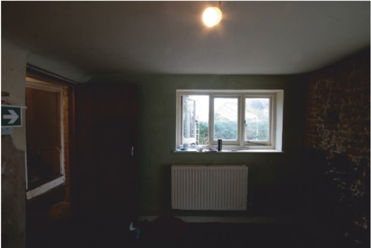
Plate 71: East wall of Kitchen, looking east (D3 014)
