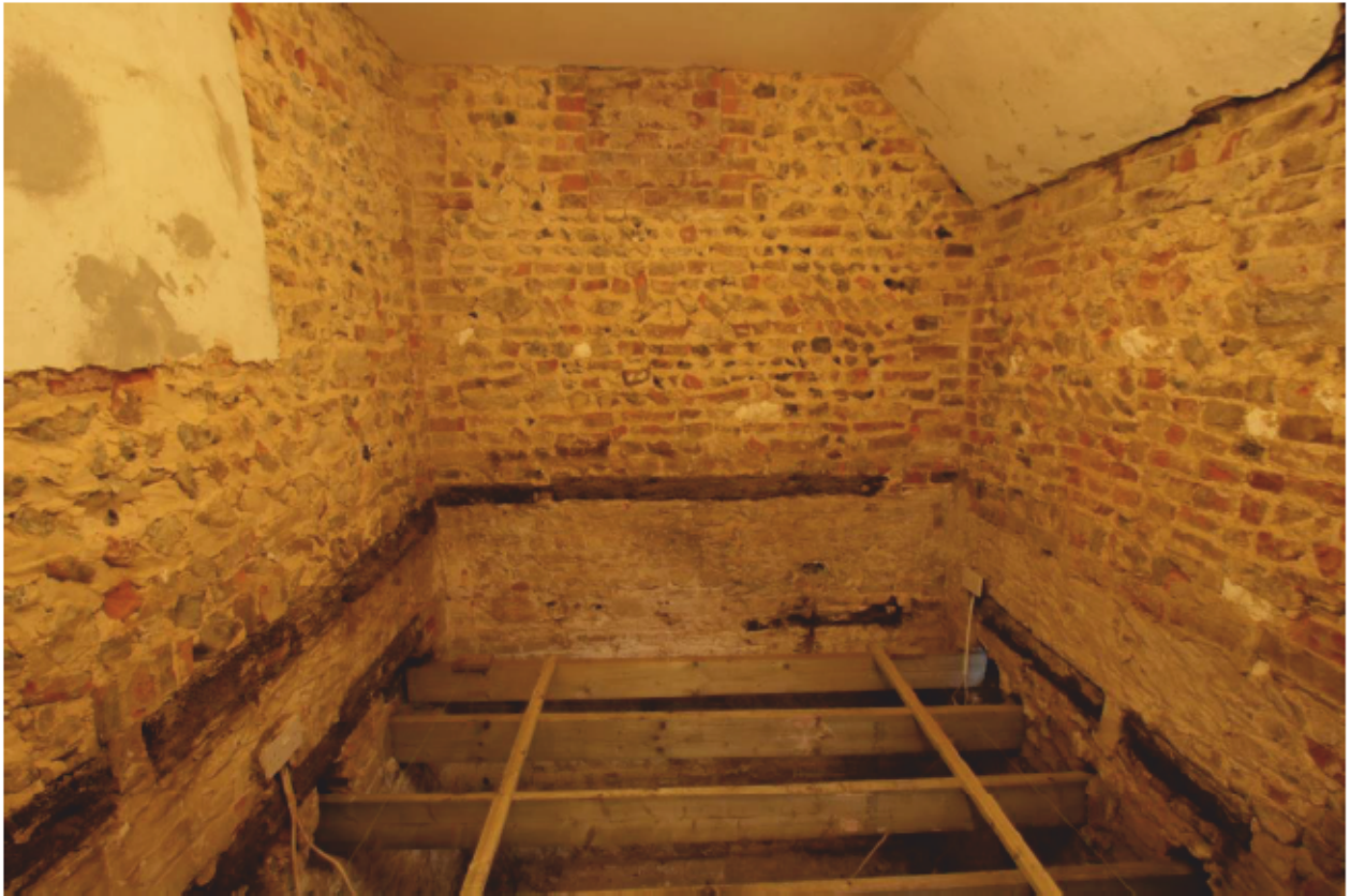
Plate 25: Blocked window in east wall of Study looking east (D1 011)
