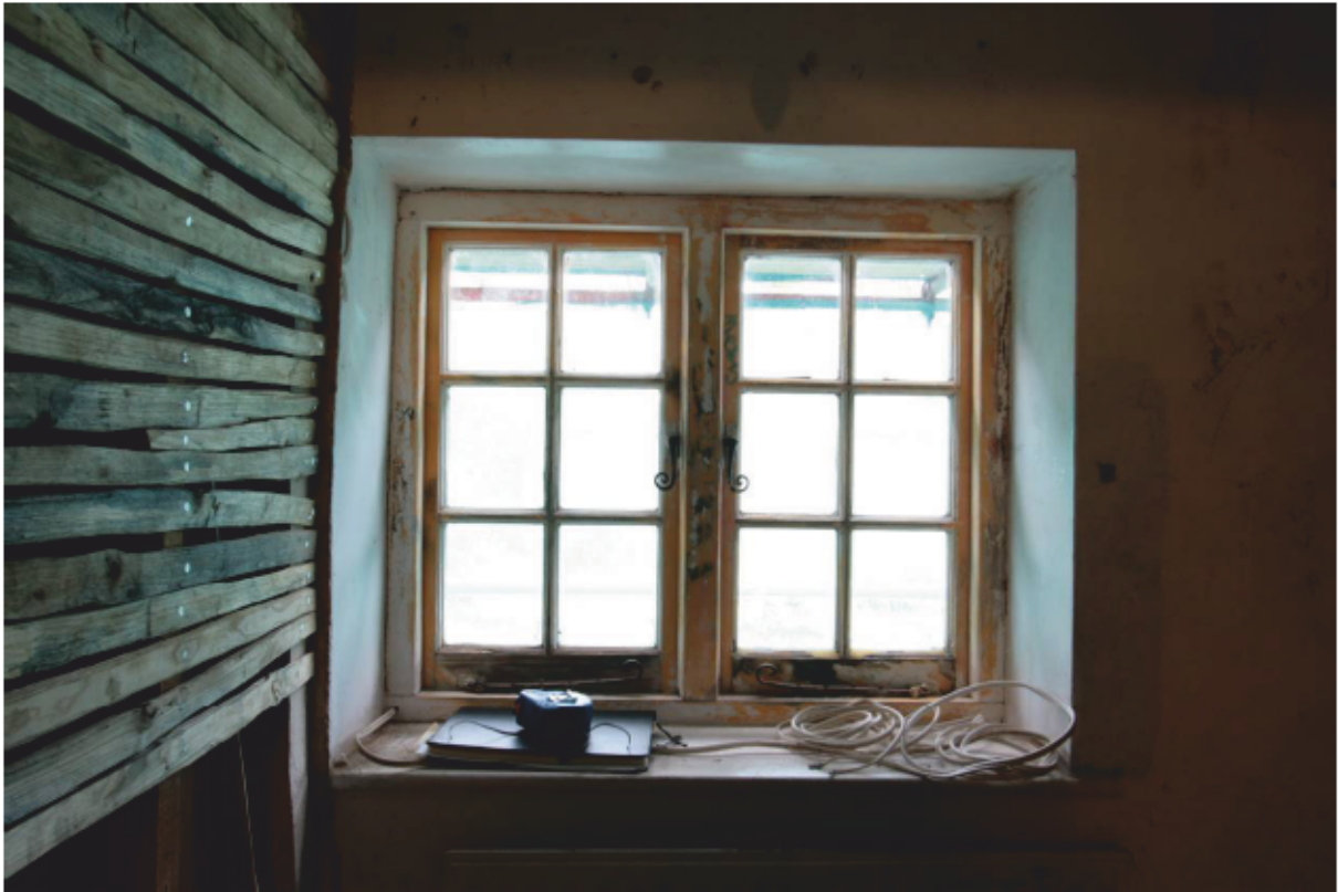
Plate 55: Bedroom 3, looking north (D2 004)
