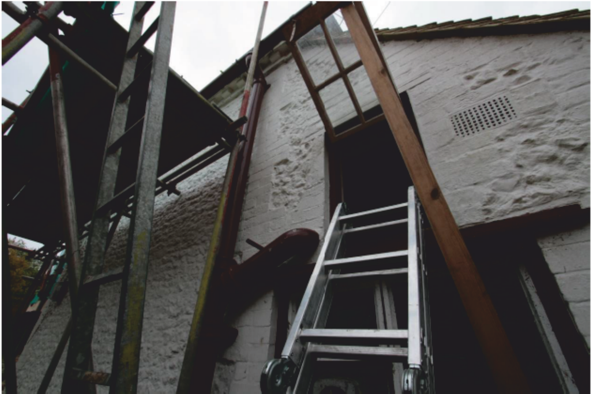
Plate 3: West external elevation displaying Utility Room Attic access (D3 007)
