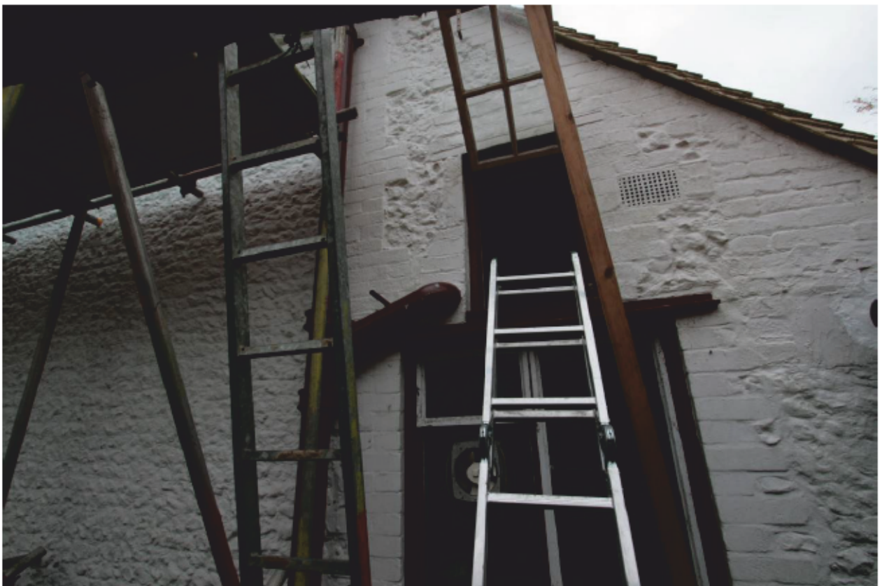
Plate 4: West elevation showing vertical brick strip in short and long work between the main house (left) and the rear pentice (right), looking east (D3 006)
