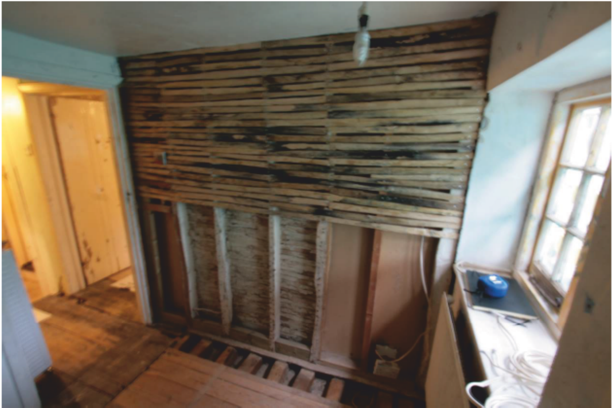
Plate 53: Bedroom 3, looking west (D2 001)
