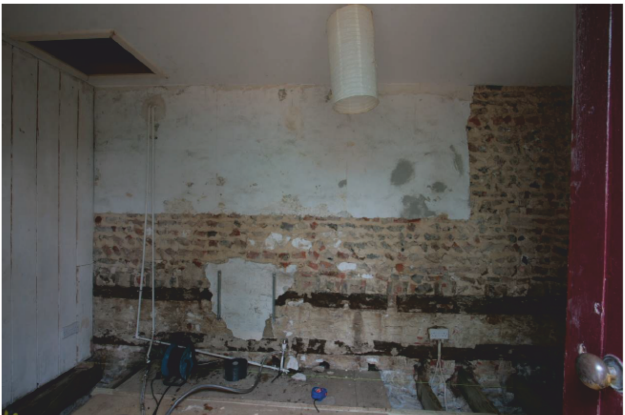
Plate 26: North wall of Study, looking north (D1 007)
