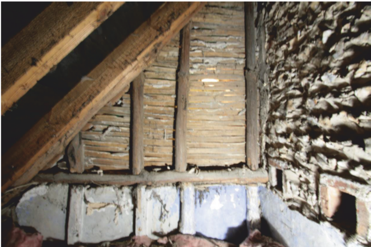
Plate 32: Roof space above Study, looking west (D1 020)
