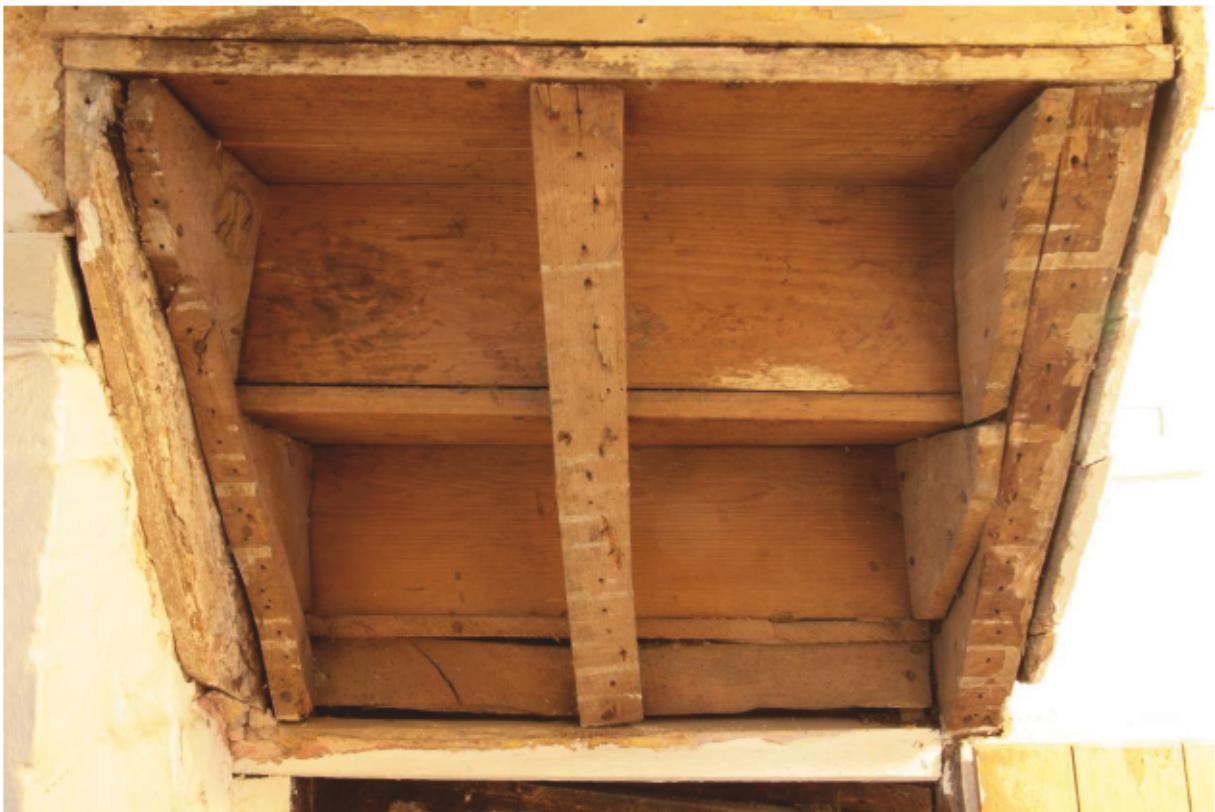
Plate 37b: Underside of staircase, looking east (D2 036)
