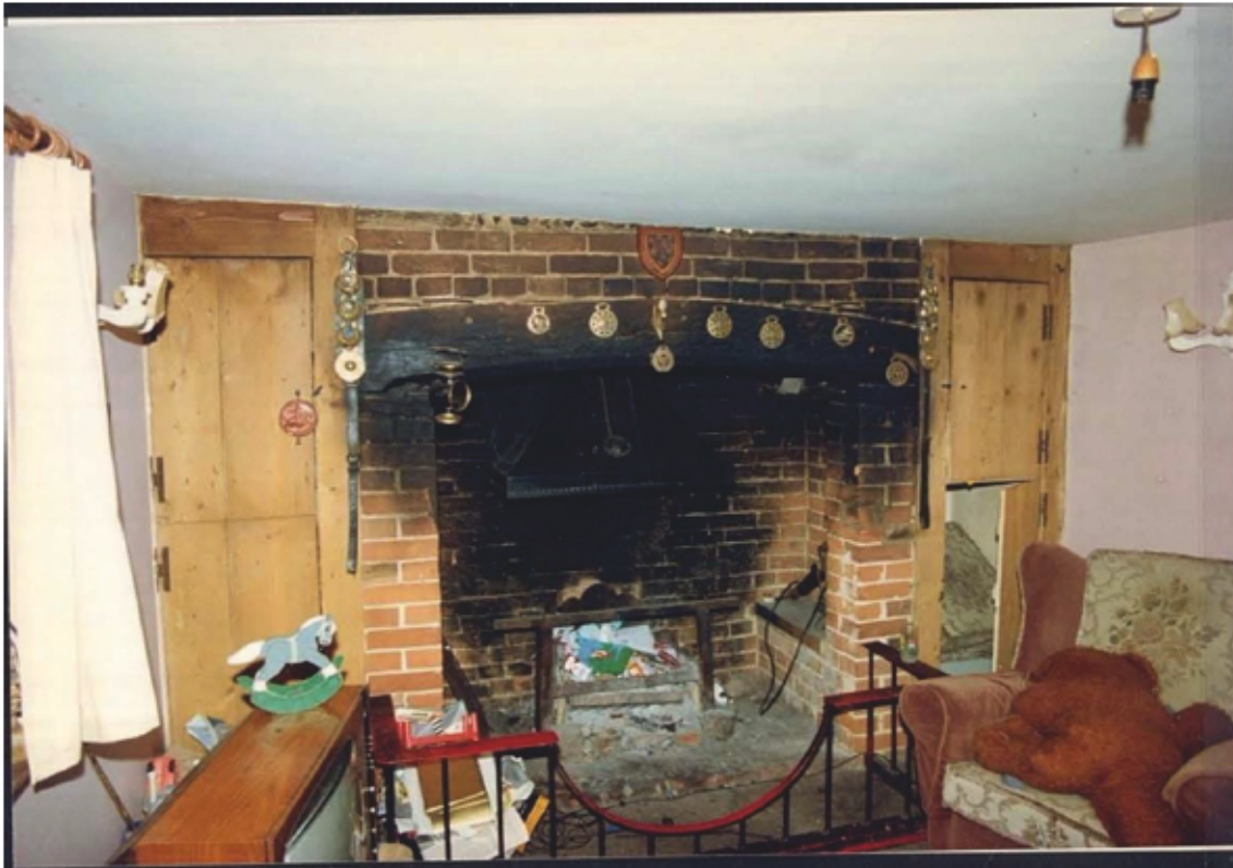
Historic Plate 19 Photograph taken by Sara Squires in September 1991 of the fireplace in the Dining Room of the Old Bakery, looking east (© National Trust Wisley)
