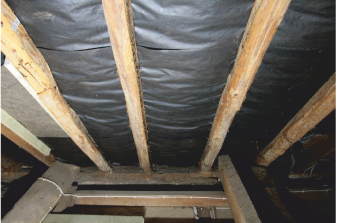
Plate 61: Common rafters in roof space over Bedroom 1, looking south (D3 025)
