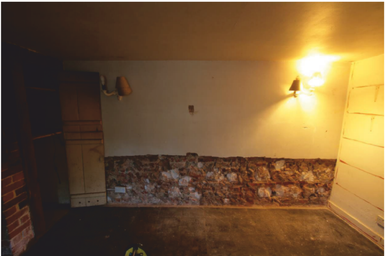
Plate 20: South wall of Dining Room, looking south (D2 027)
