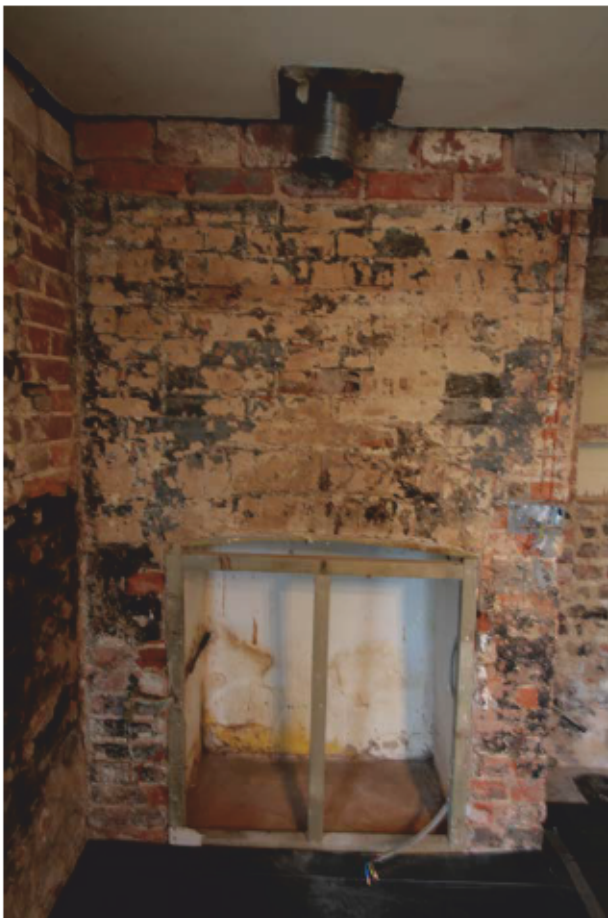
Plate 68: Fireplace in west wall of Kitchen, looking west (D3 029)
