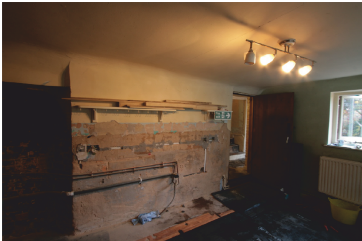
Plate 70: North wall of Kitchen, looking north-east (D3 013)
