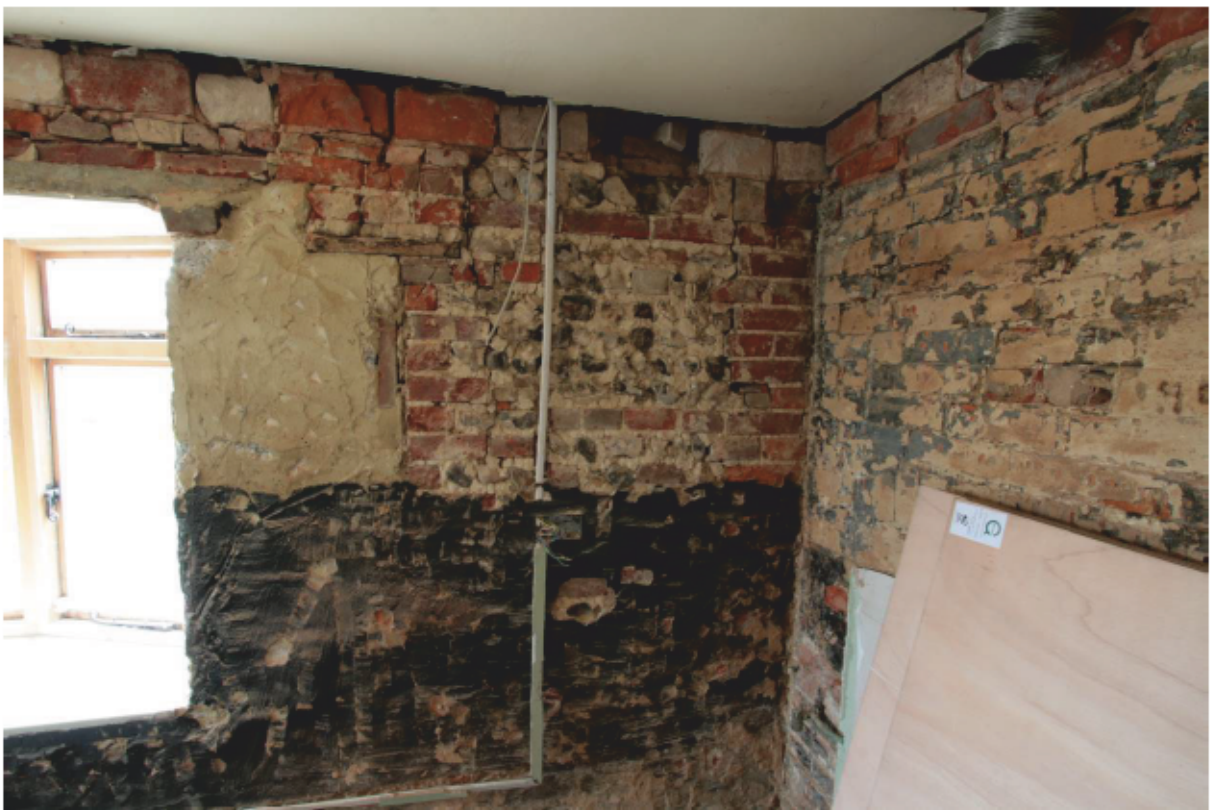
Plate 66: West side of south wall of Kitchen, looking south (D3 017)
