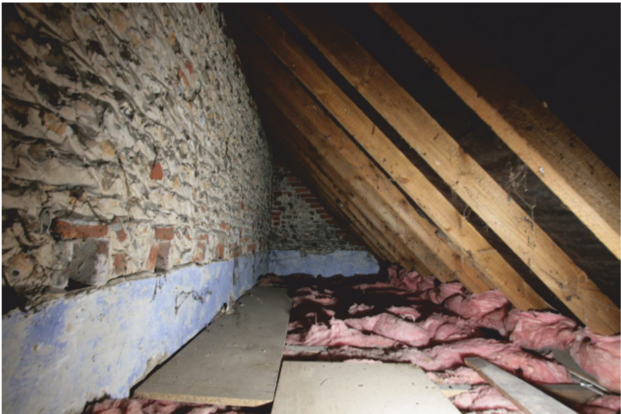
Plate 30: Roof space above Study, looking east (D1 019)
