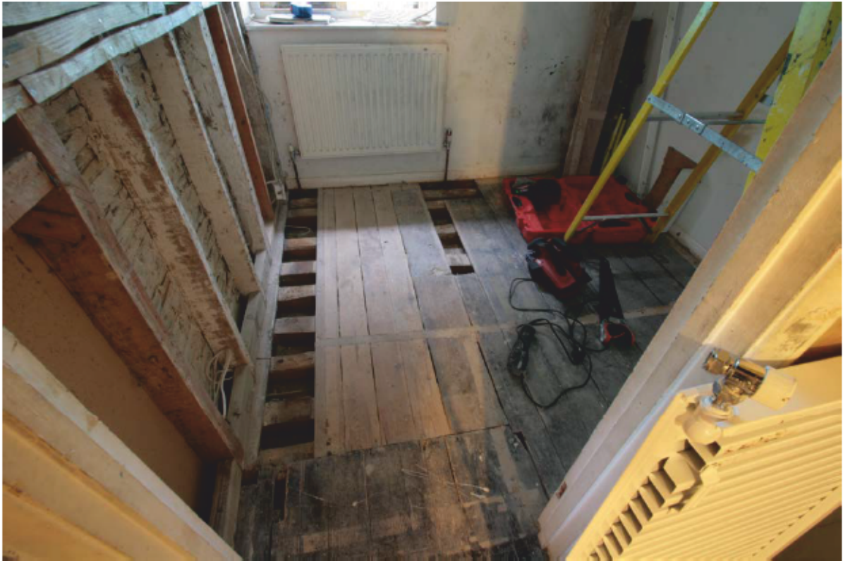
Plate 57: Bedroom 3, looking north (D2 003)
