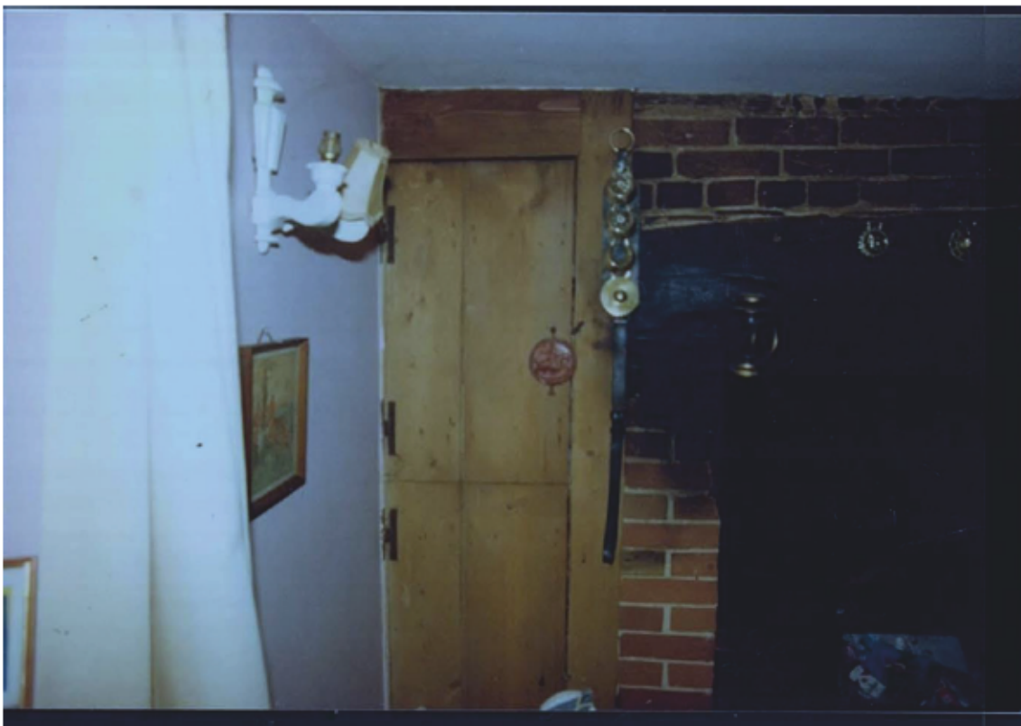
Historic Plate 20 Photograph taken by Sara Squires in September 1991 of the cupboard on the north side of the fireplace in the Dining Room of the Old Bakery, looking east (© National Trust Wisley)
