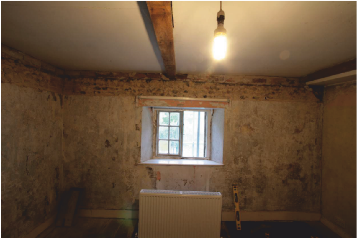
Plate 49: Bedroom 2, looking north (D2 012)
