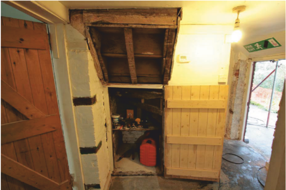
Plate 37a: Underside of staircase, looking east (D1 069)
