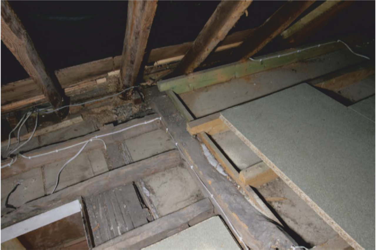
Plate 63: Roof space over Bedrooms 2 (right) and Landing (left), looking south (D3 028)
