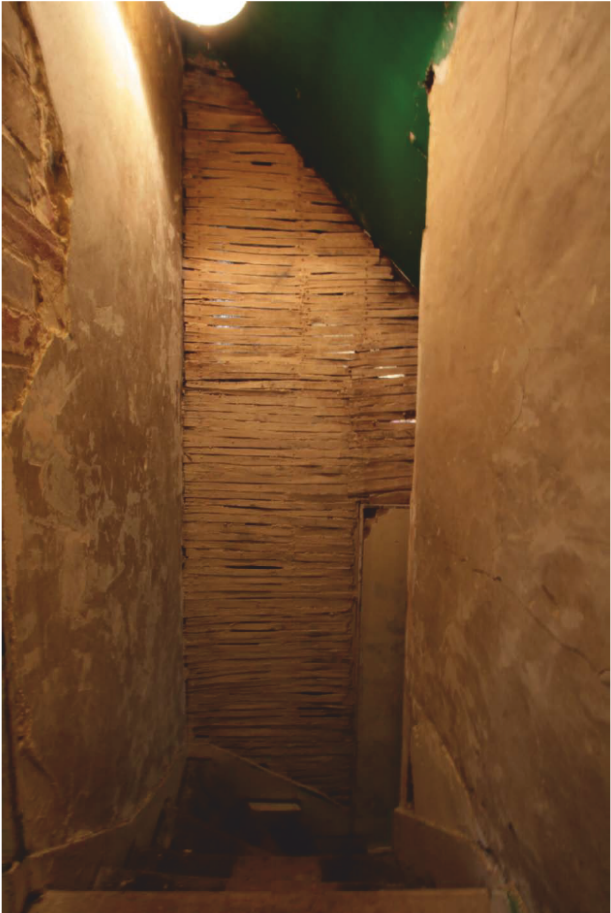
Plate 36: Stairwell looking east and down from first floor facing east (D1 026)
