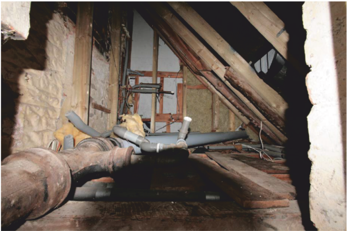
Plate 44: Roof space above Utility, looking east (D3 009)
