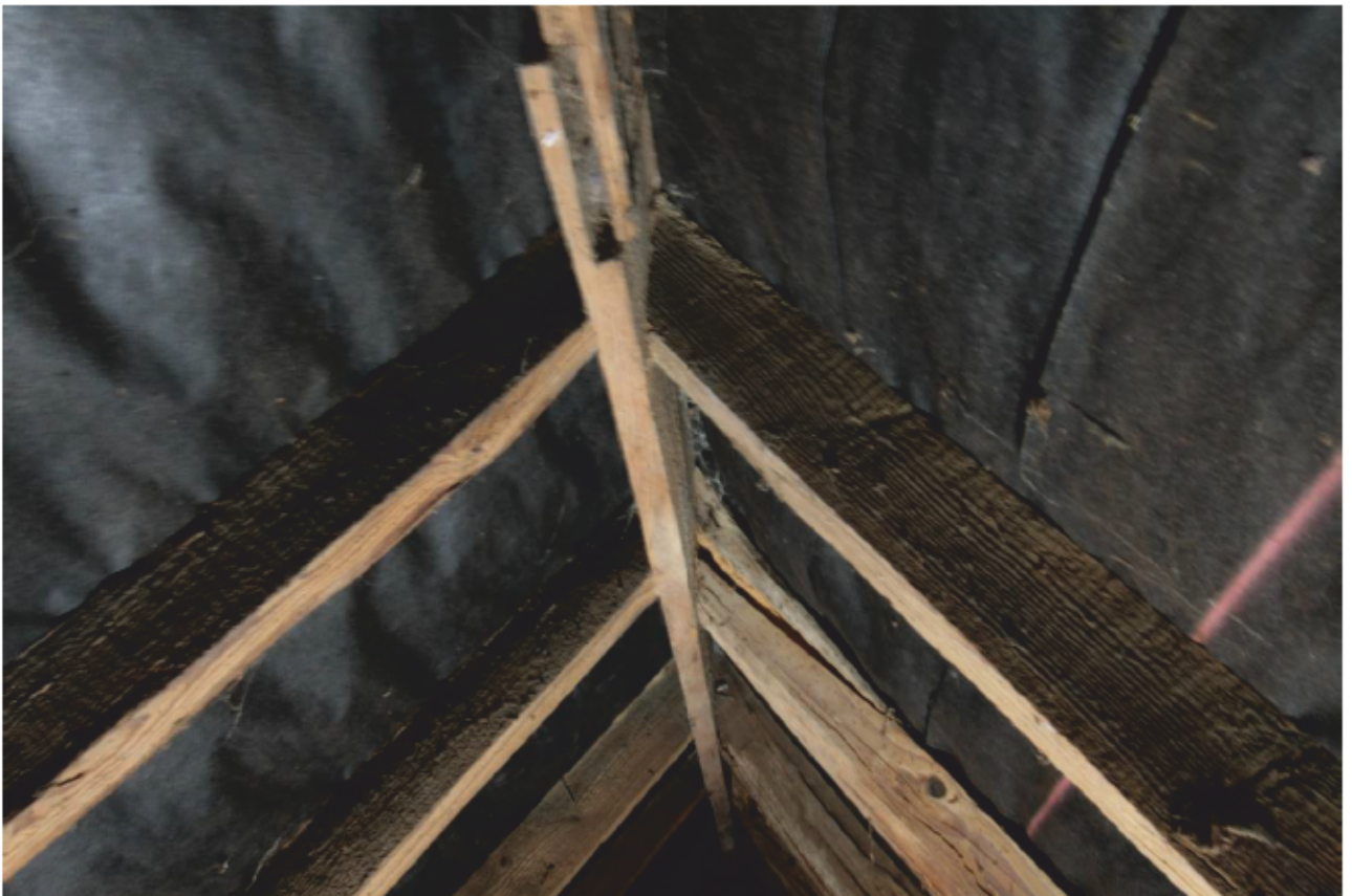
Plate 64: Roof space over Bedrooms 1 to 3, looking east (D3 026)
