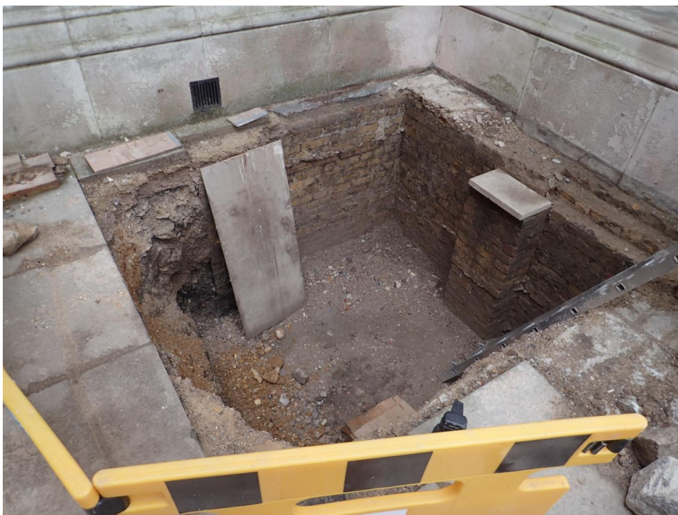
Plate 1: Lift pit, facing southwest
