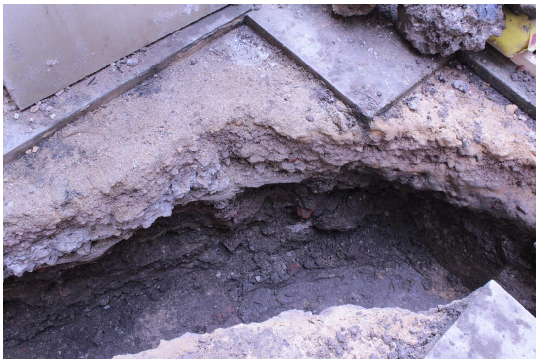
Plate 6: Service trench, Section 5. Facing north-west
