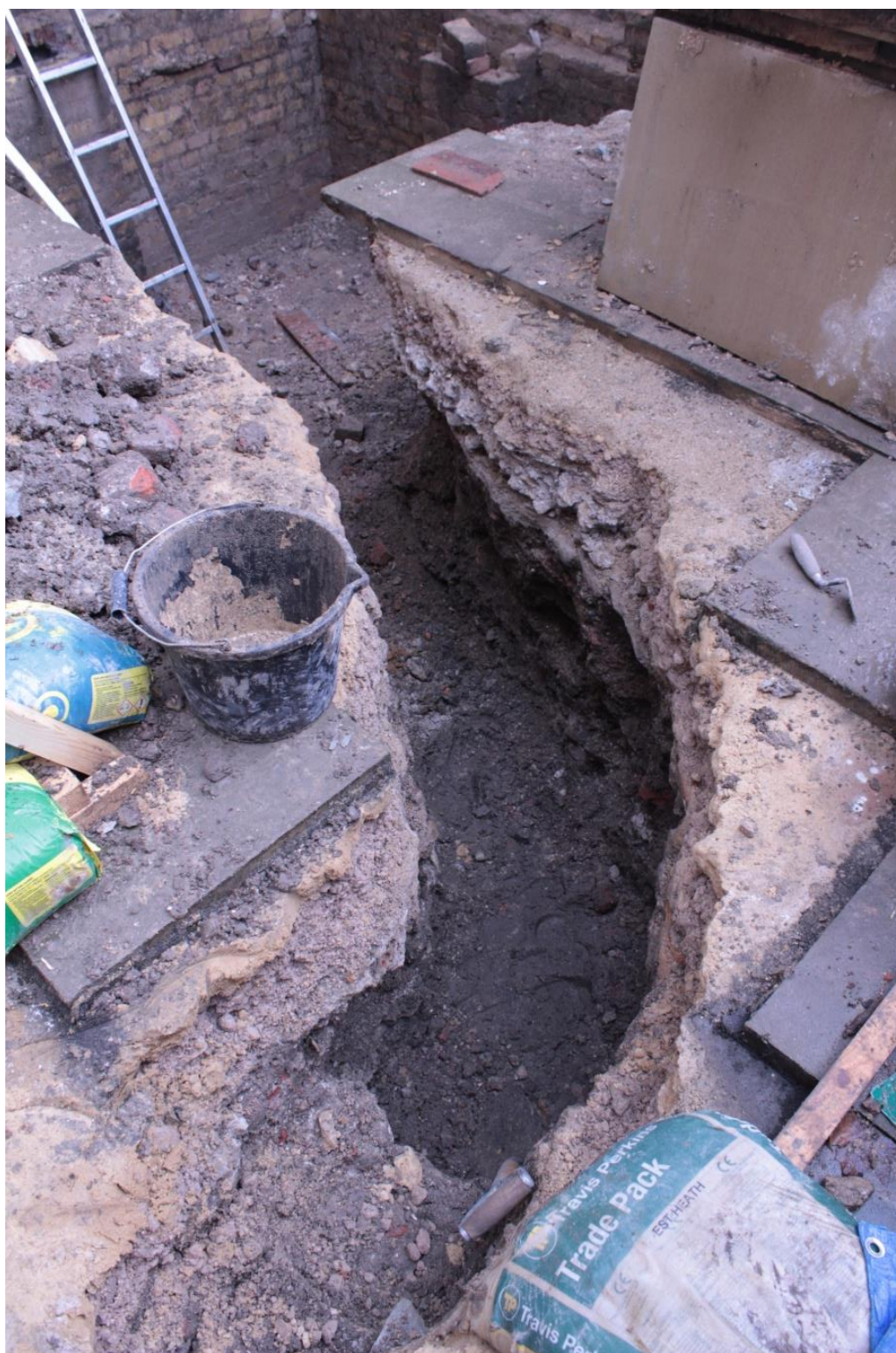
Plate 5: Overview of service trench, facing south-west
