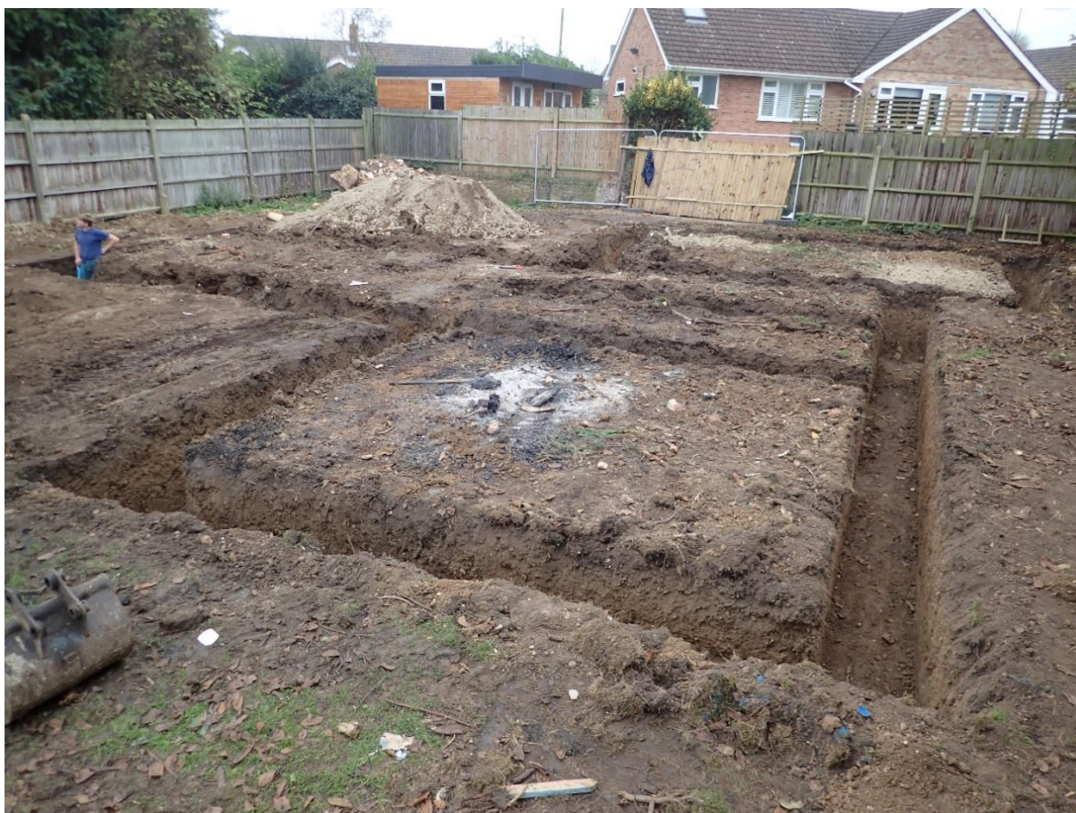
Plate 1: Foundation trench, looking south-east.
