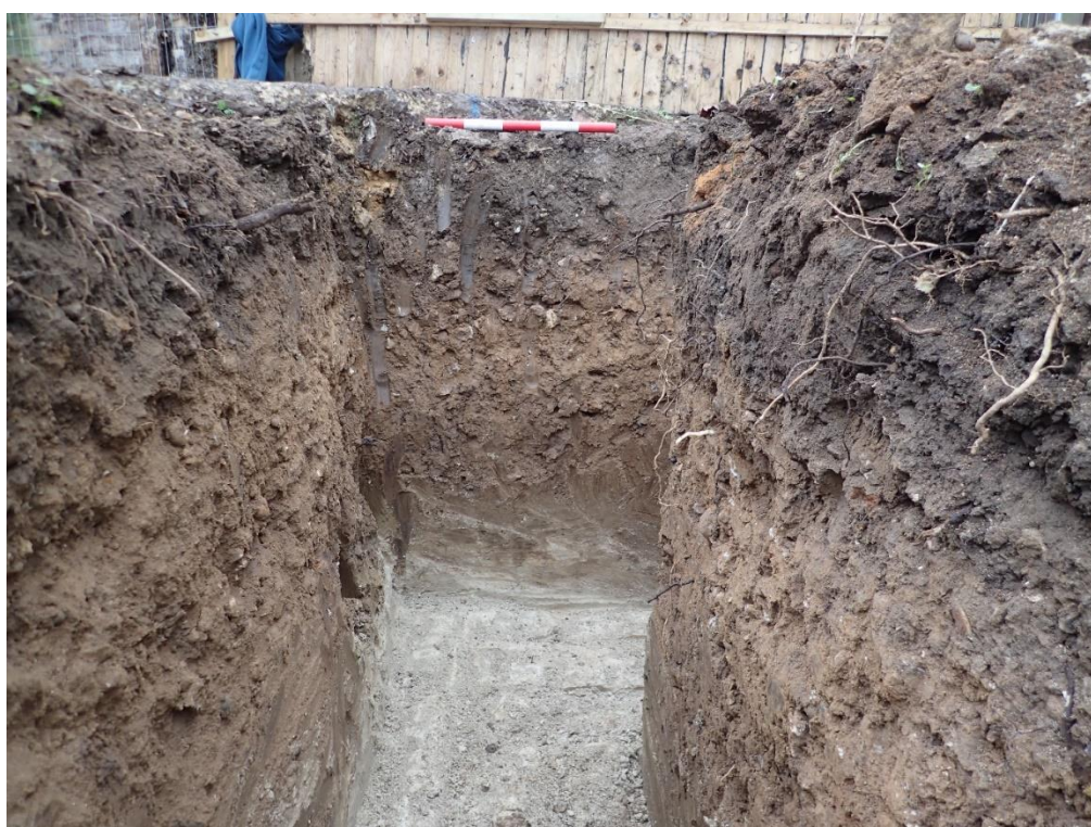
Plate 3: Foundation trench, Section 9. Looking south.
