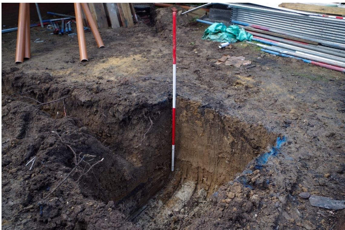
Plate 6: Soakway Pit 2. Looking south-east.
