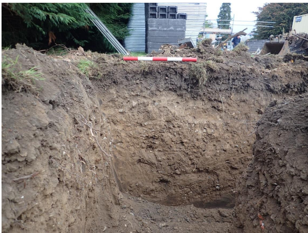
Plate 2: Foundation trench, Section 7. Looking north.
