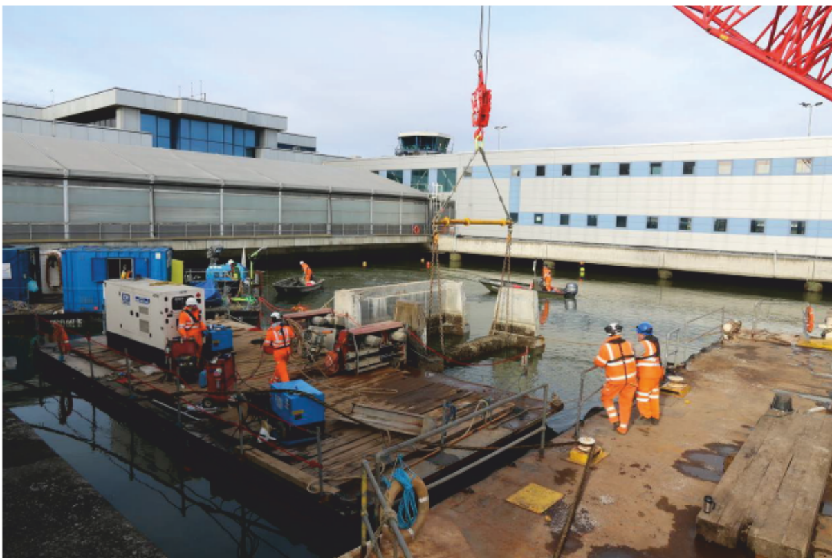
Plate 44: Cradled brace cut from Dolphin 7 using waterborne diamond wire saw, looking north-west
