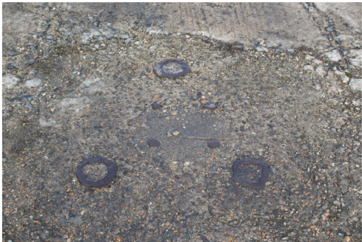
Plate 4: Historic crane mooring at east end of south side of King George V Dock, looking north (CIY17 D1 5)
