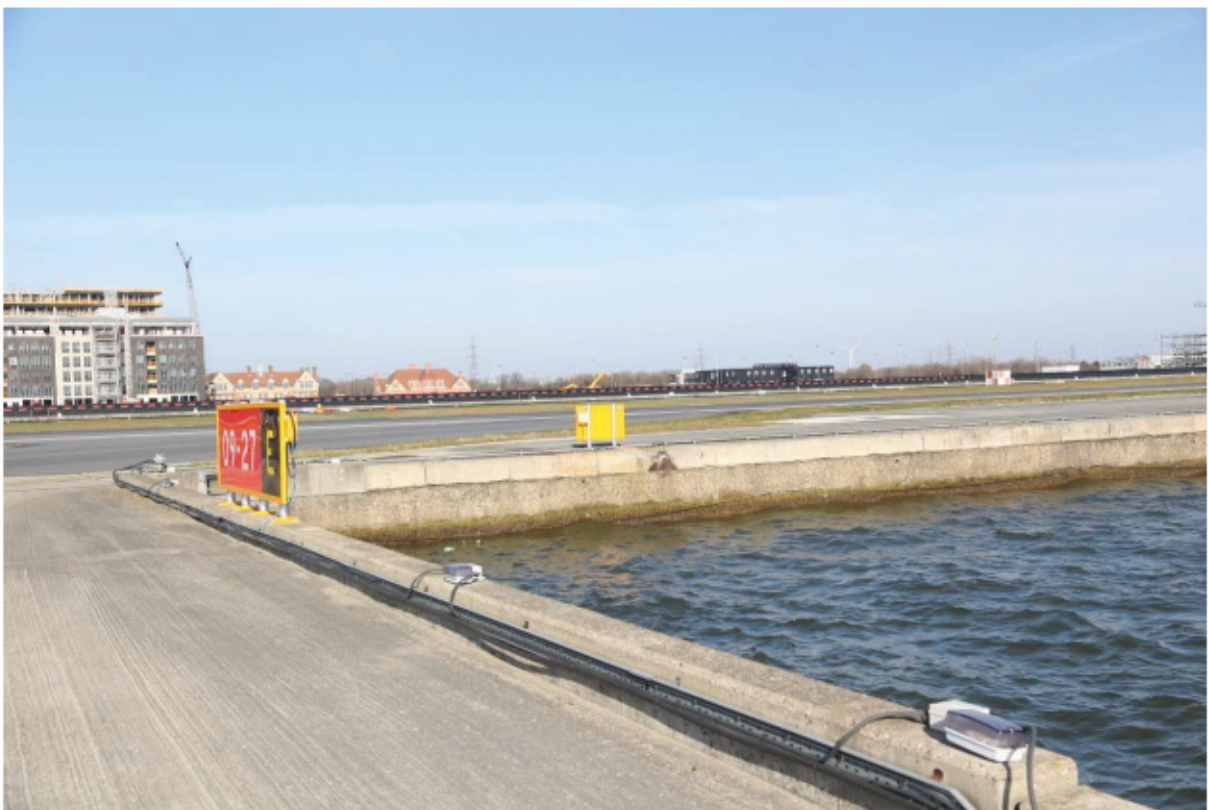
Plate 68: Coping stones on north quayside of King George V Dock, looking north
