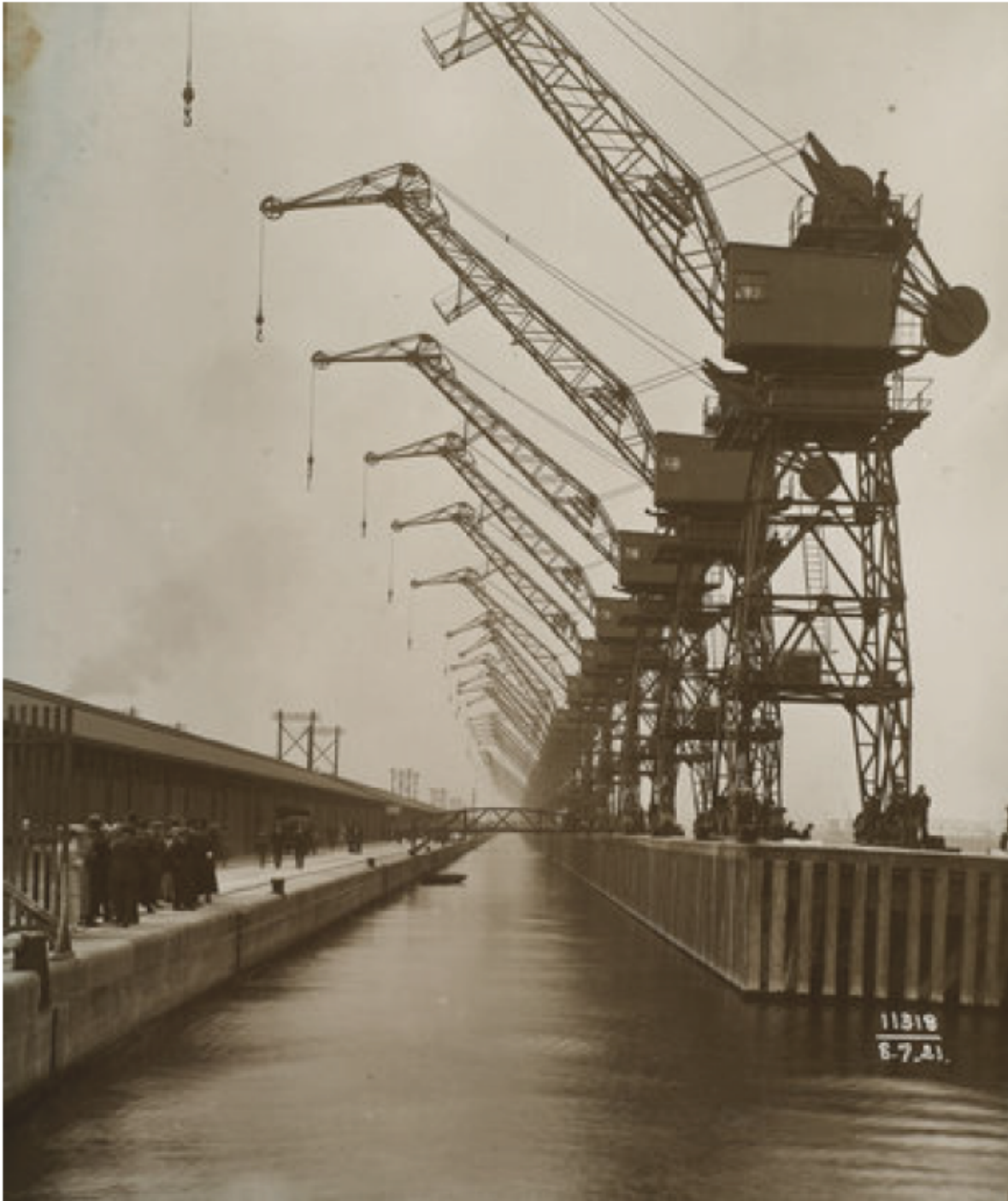
Historic Plate 5: Forty-two new Babcock & Wilcox electric quayside cranes on the Dolphins at the south side of King George V Dock on opening day, 8 July 1921, looking west (© PLA collection/Museum of London)
