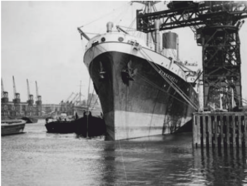
Historic Plate 19: Photograph taken c.1960 of the 'Menestheus' (1958) moored at one of the concrete 'dolphins' or jetties in the King George V Dock, looking east (©National Maritime Museum, London)
