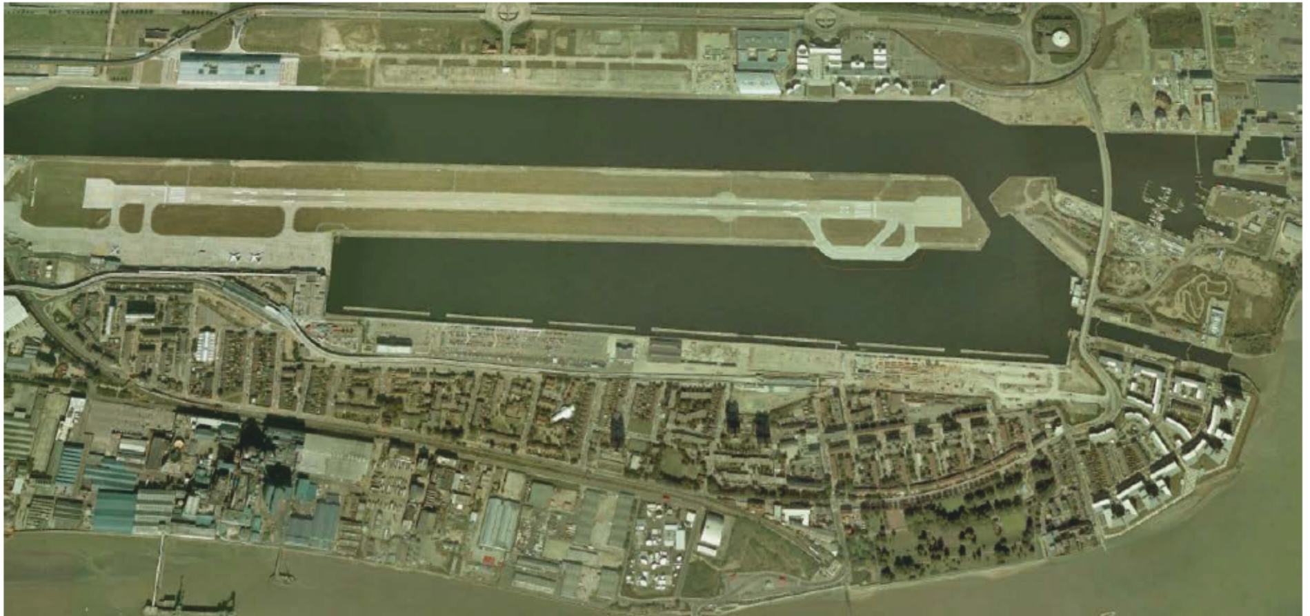
Historic Plate 25: Aerial view of King George V Dock showing DLR c.2005
