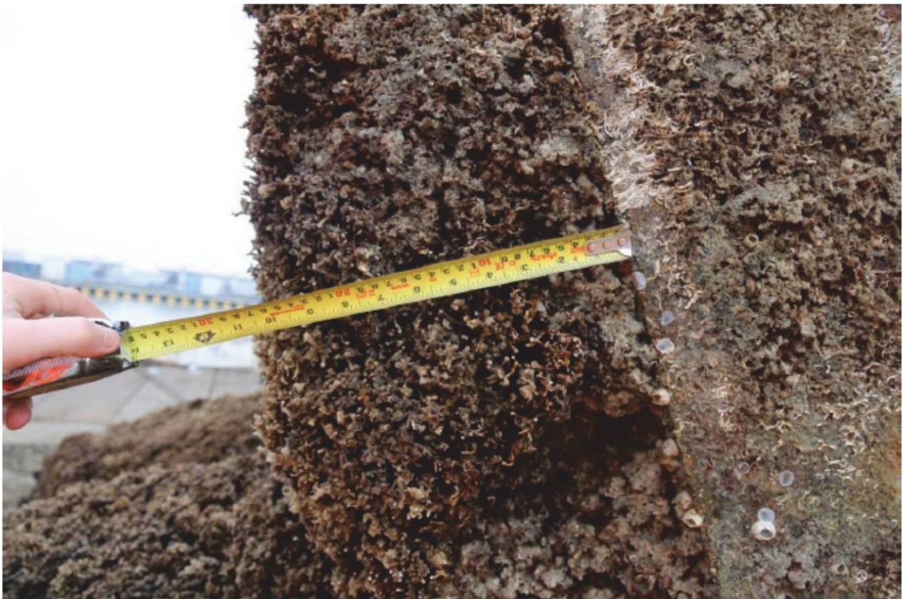
Plate 56: Aquatic growth on the below-water part of Dolphin 7, looking north (CIY17 D3 26)
