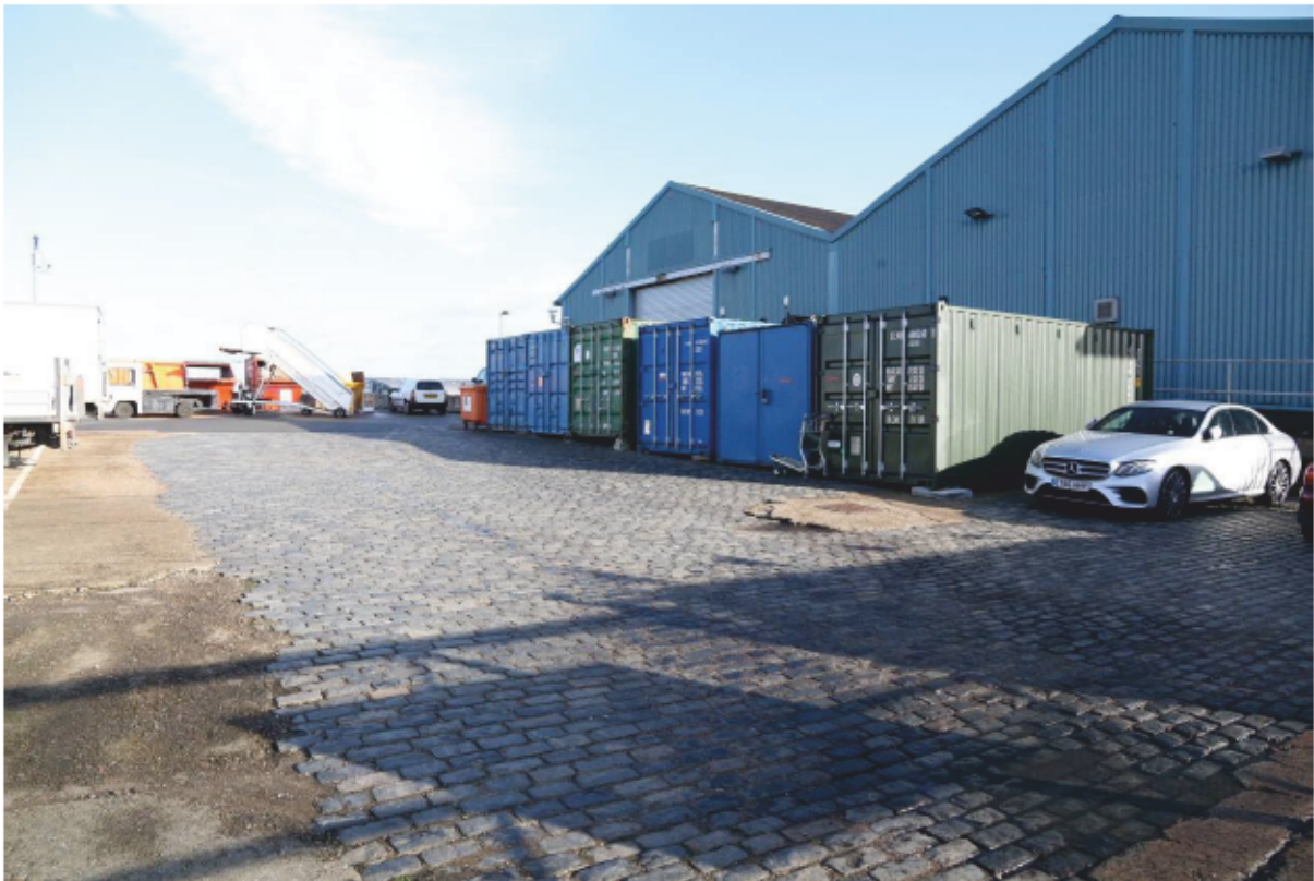
Plate 28: Granite setts in the gap between Transit Sheds 4 and 5 on the south side of King George V Dock, looking north (CIY17 D5 3)
