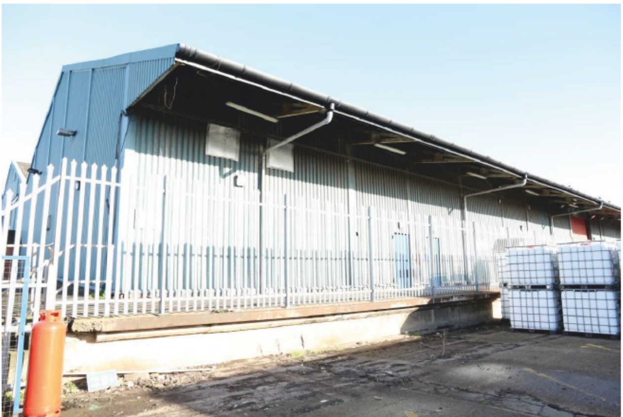
Plate 22: Original steel frame of Transit Shed 4 re-clad on the south side of King George V Dock, looking north-east (CIY17 D5 11)
