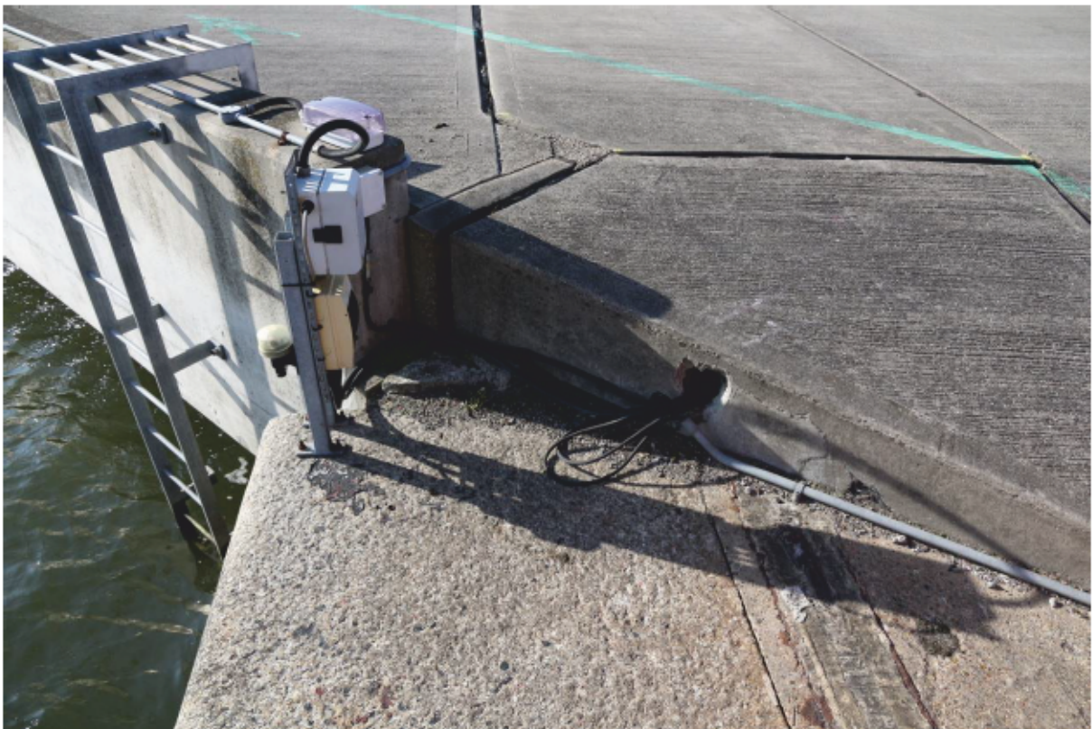
Plate 74: Coping stones continue under runway extension along north quayside of King George V Dock, looking west
