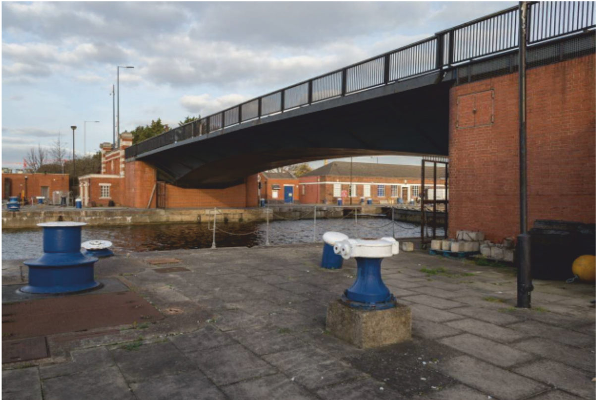
Plate 39: Steel Bascule Bridge that replaced the former Bascule Bridge at the mouth of King George V Dock, looking north-east (CIY17 D100 042)
