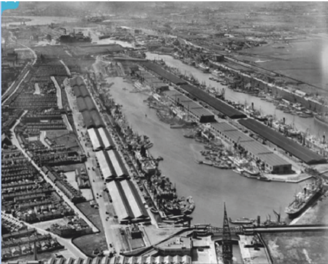
Historic Plate 7: King George V Dock, 1928, looking west (©Britain from Above)
