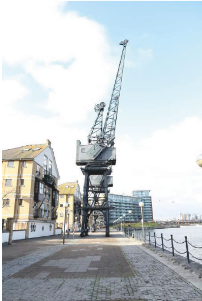
Plate 5: Historic crane remaining on the Royal Victoria Dock, looking west (CIY17 D6 15)
