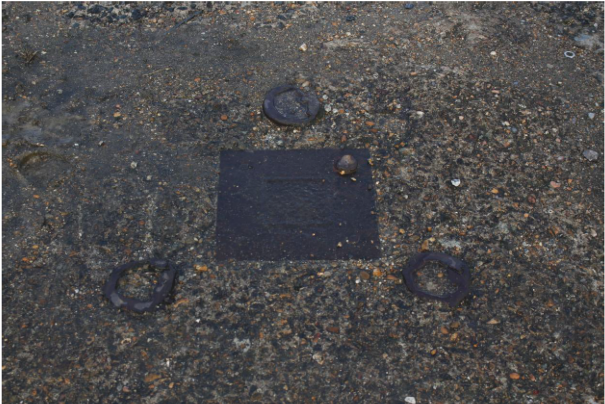
Plate 3: Historic crane mooring at east end of south side of King George V Dock, looking north (CIY17 D1 4)
