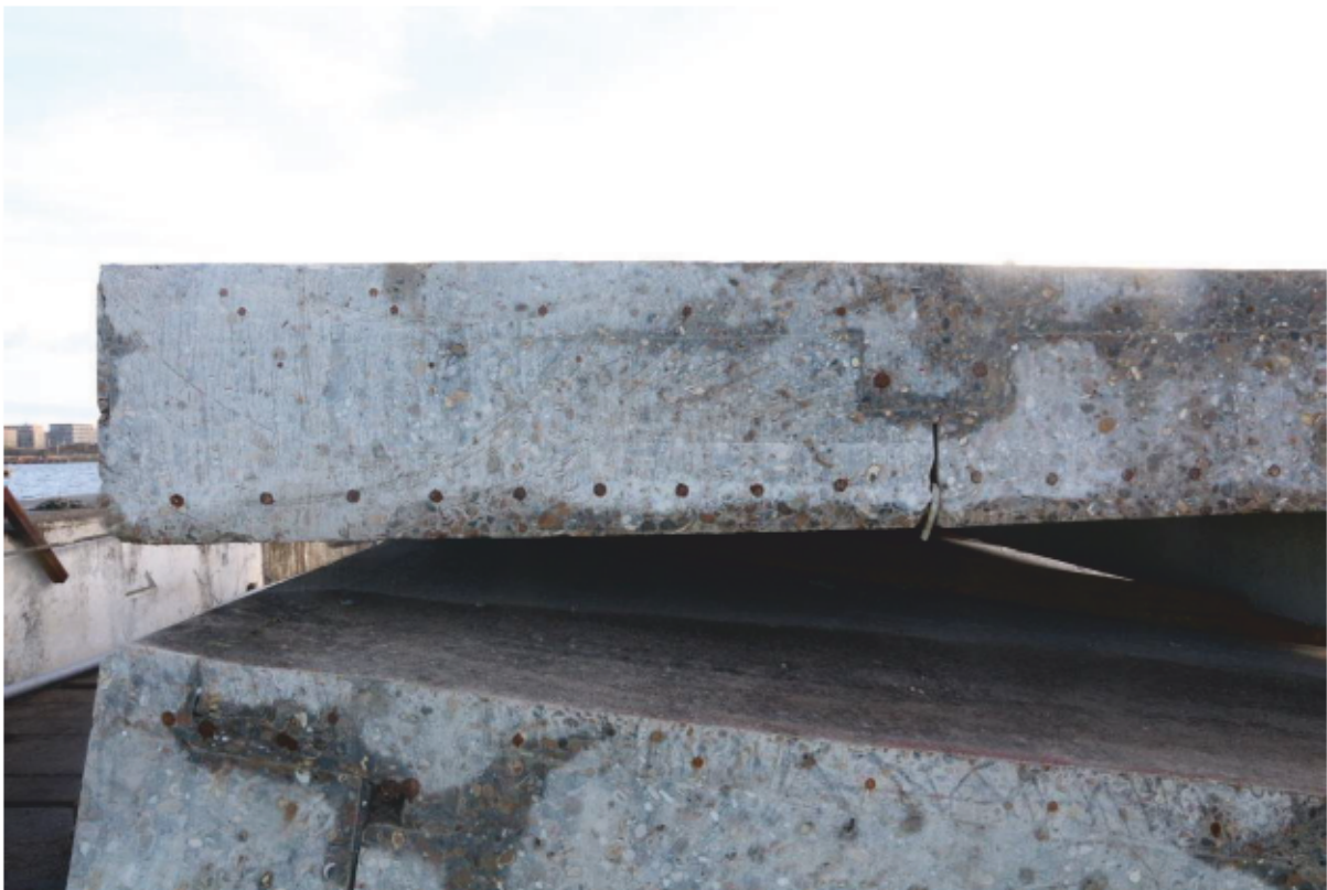
Plate 50: Detail of Dolphin 7's cap, looking east (CIY17 D2 5)
