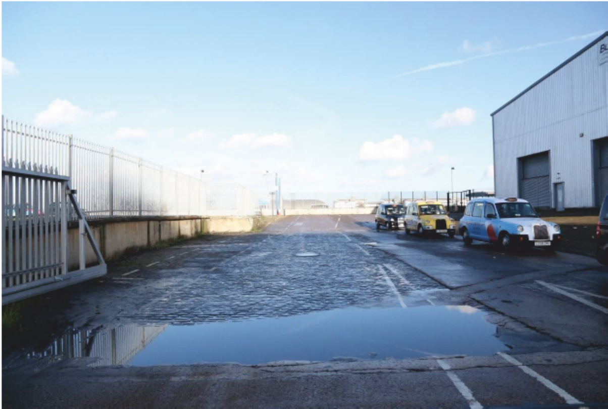
Plate 29: Granite setts in the gap between former Transit Sheds 3 and 4 on the south side of King George V Dock, looking north (CIY17 D5 26)
