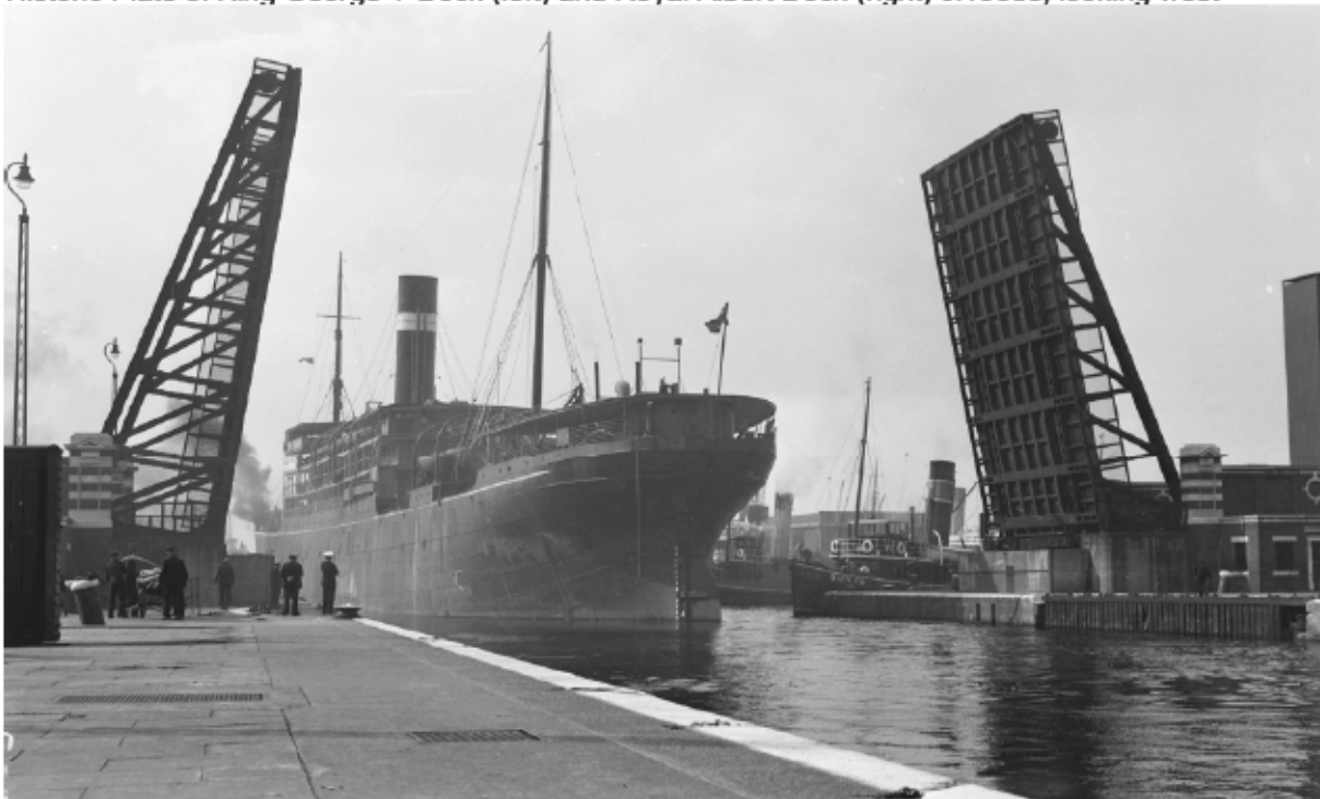
Historic Plate 9: Manor Way bascule bridge closing behind the SS 'Morvada' as she enters King George V Dock on 13th September 1931, looking north-west (© Museum of London)
