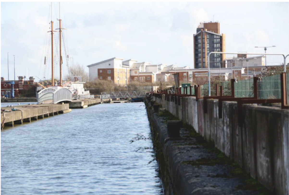
Plate 14: Mooring posts along the east end of the south side of King George V Dock with the Dolphins 1 and 2 to the left, looking east (CIY17 D5 39)
