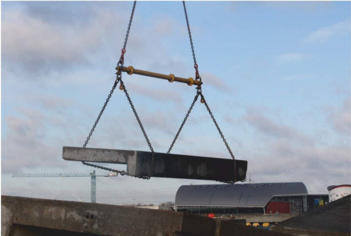
Plate 47: Detail of Dolphin 7's cap lifting operations, looking north (CIY17 D2 17)
