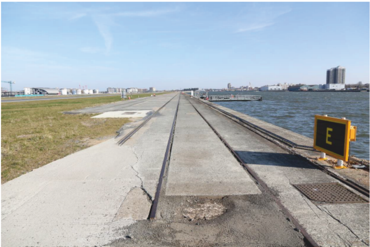
Plate 80: Railway tracks along north quayside of King George V Dock, looking east
