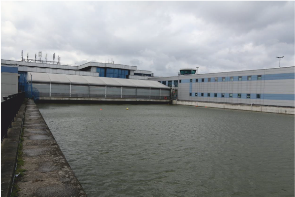
Plate 67: West end of King George V Dock after removal of the upper part of Dolphin 7, looking north-west
