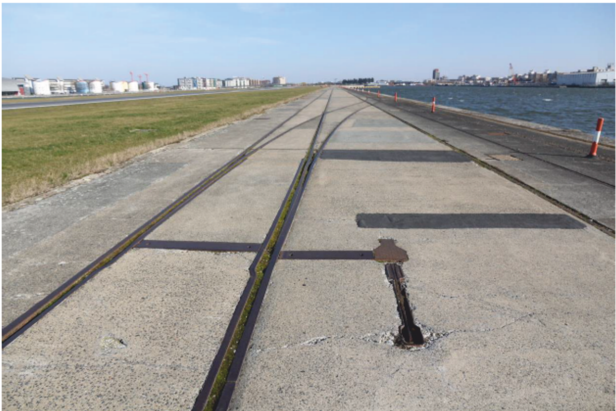
Plate 84: Manual railway track switch along north quayside of King George V Dock, looking east
