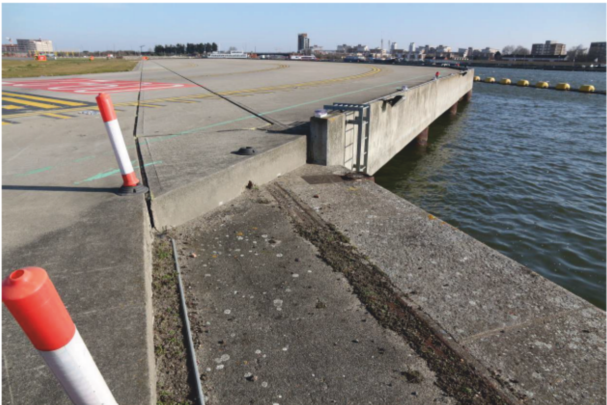
Plate 72: Railway tracks and coping stones continue under runway extension along north quayside of King George V Dock, looking east
