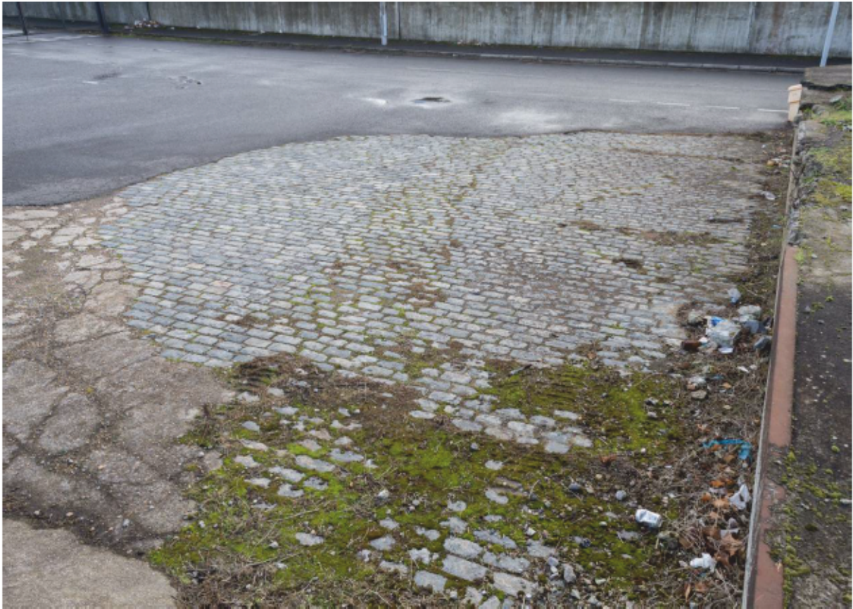
Plate 27: Granite setts in the gap between former Transit Sheds 2 and 3 on the south side of King George V Dock, looking south (CIY17 D100 052)
