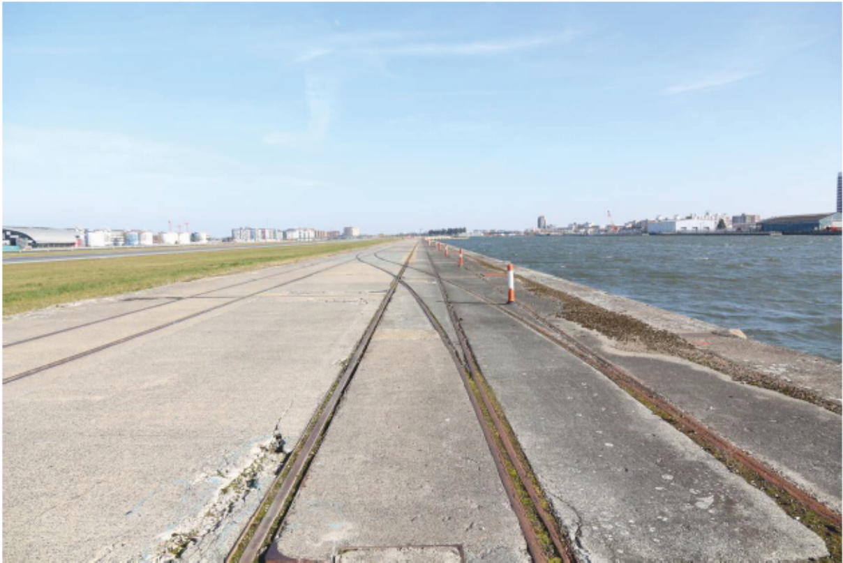
Plate 81: Railway tracks along north quayside of King George V Dock, looking east
