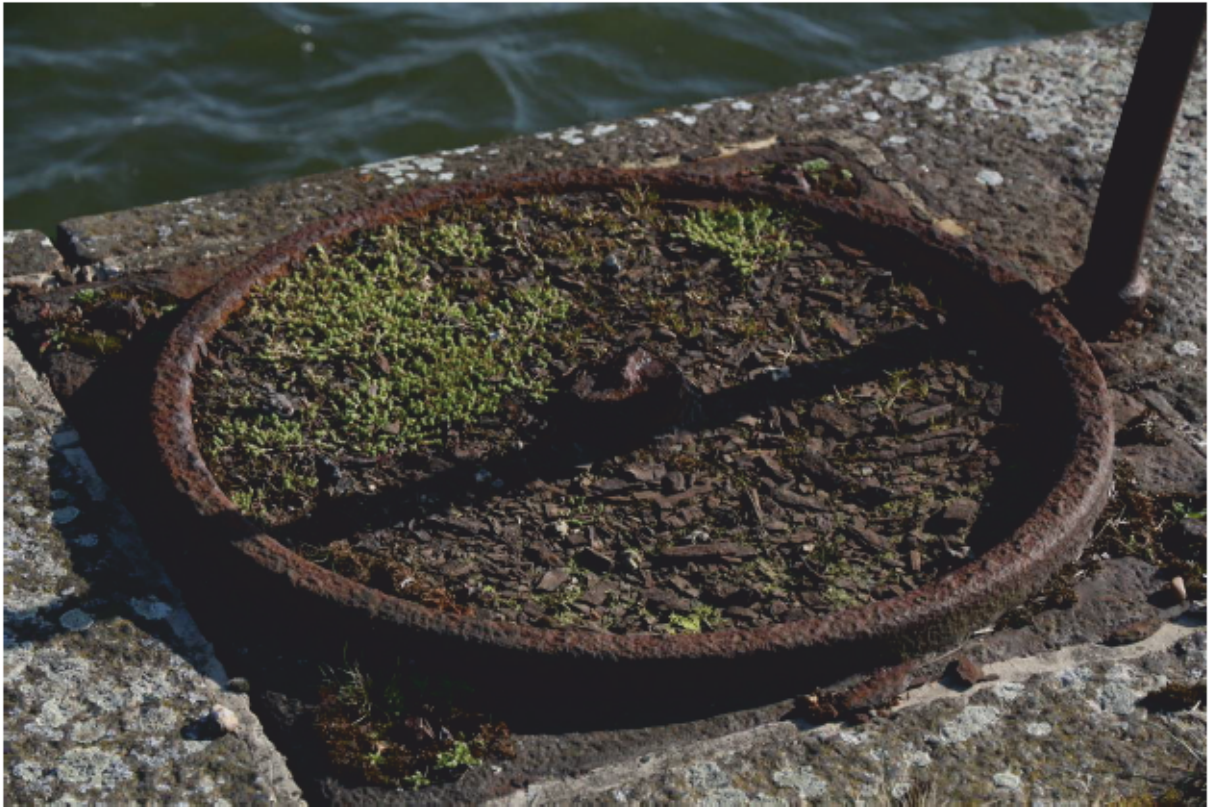
Plate 79: Remains of mooring post on the north quayside of King George V Dock, looking east
