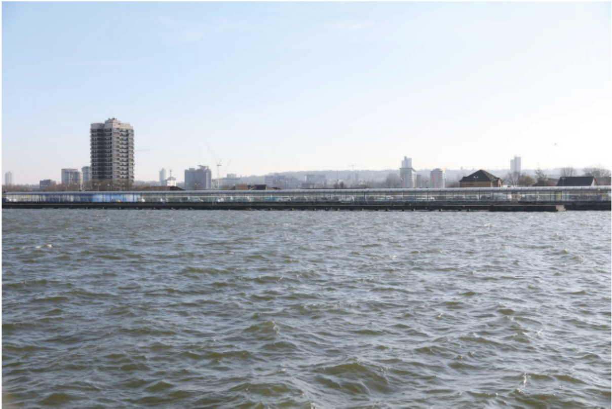
Plate 91: View of Dolphin 6 from north quayside of King George V Dock, looking south
