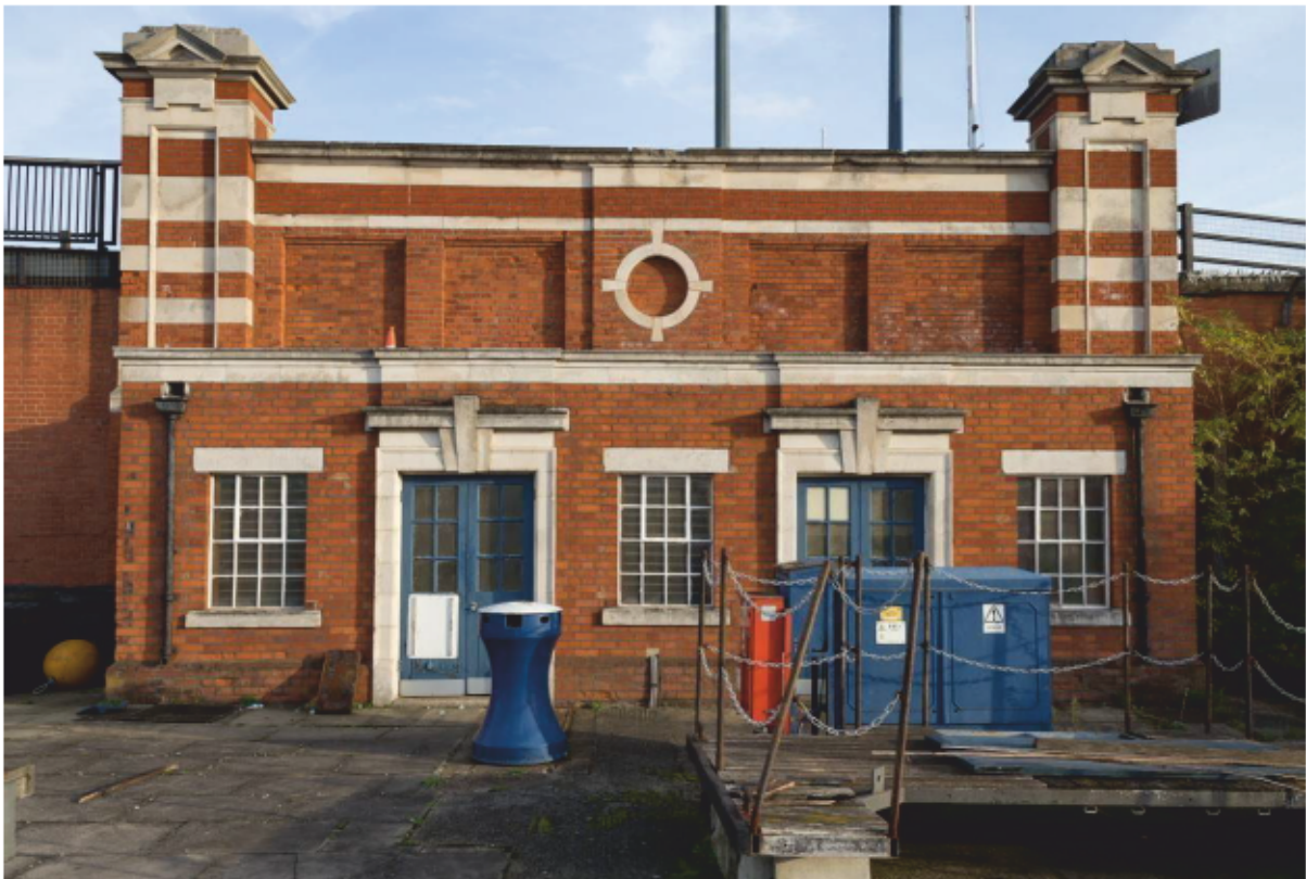
Plate 38: Housing for mechanism of Bascule Bridge at the mouth of King George V Dock, looking east (CIY17 D100 041)
