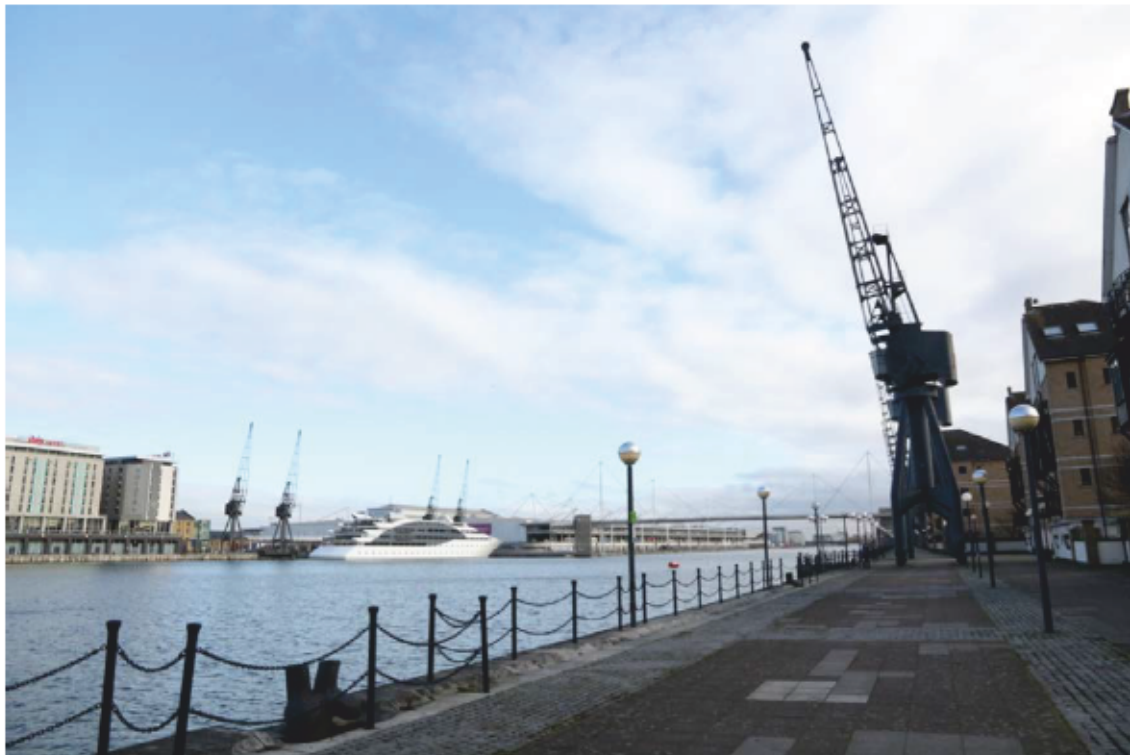
Plate 6: Historic cranes on the Royal Victoria Dock, looking east (CIY17 D6 18)
