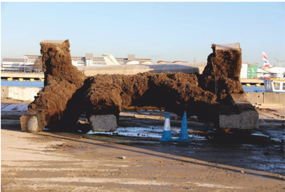
Plate 64: Below water part of Dolphin 7, looking north (CIY17 D4 29)
