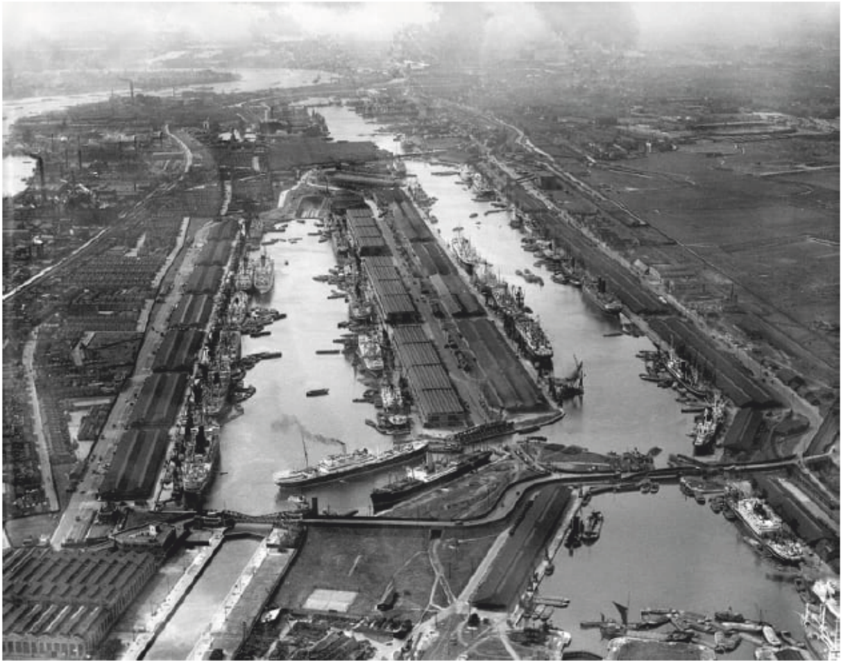
Historic Plate 10: King George V Dock and the Royal Albert Dock, 1934, looking west
