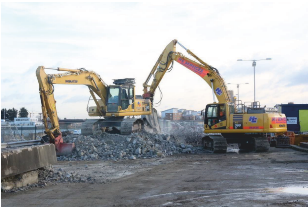
Plate 48: Demolition and separation of Dolphin 7's cap, looking east (CIY17 D2 12)
