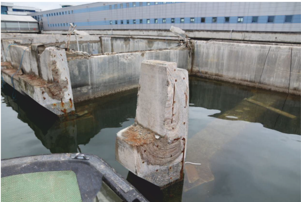
Plate 66: Cross sections of Dolphin 7's step for downturned lip cover in situ , looking north-west (CIY17 D3 108)
