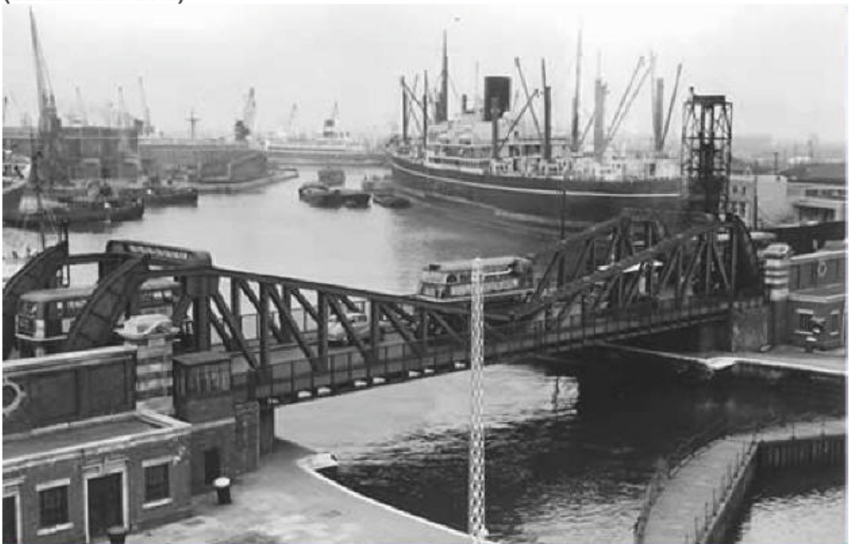
Historic Plate 16: Photograph taken in 1953 of the Bascule Bridge, looking west from King George V Lock
