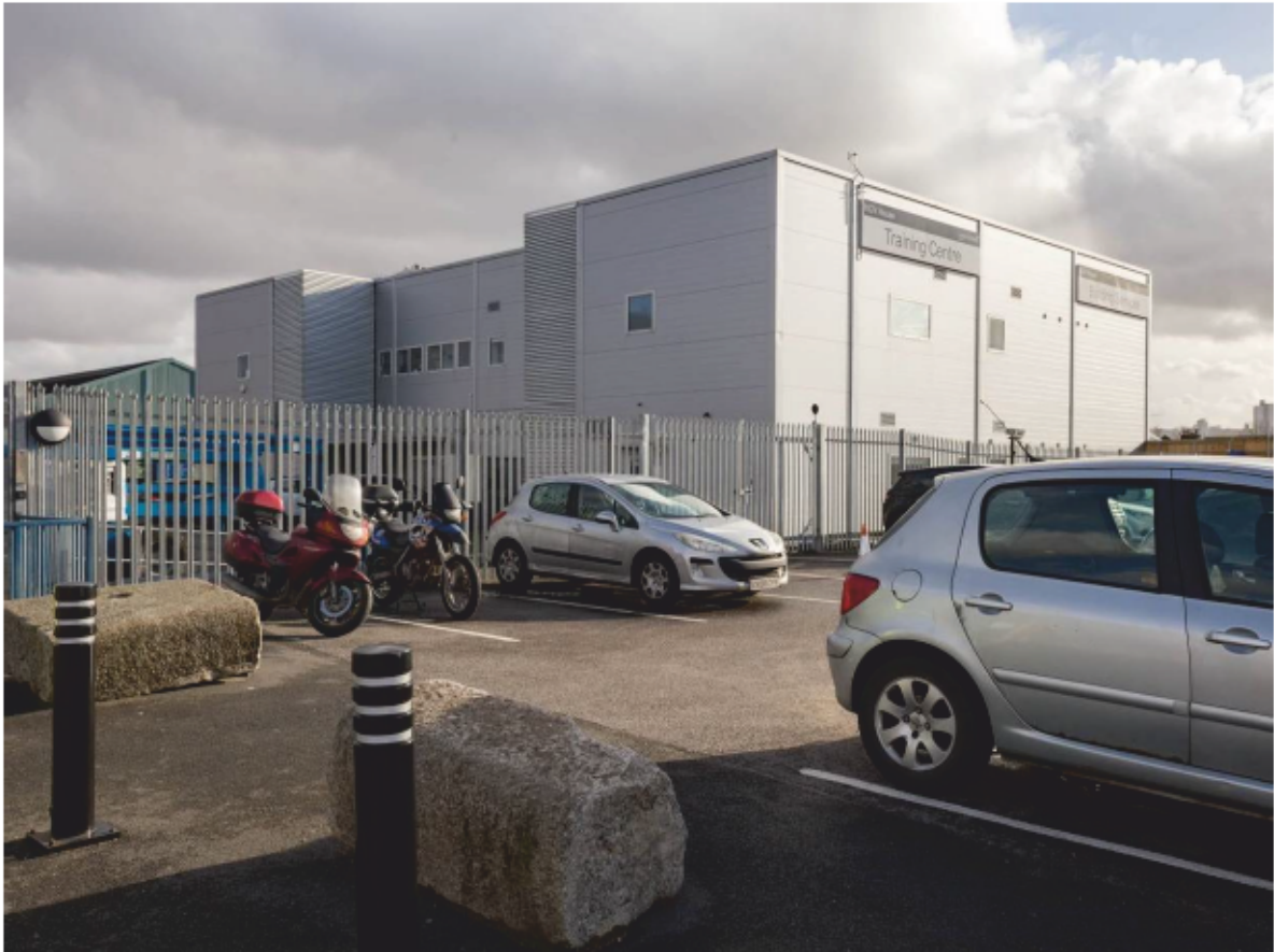
Plate 9: KGV House on the south side of King George V Dock at the east end of former Transit Shed 5, looking south-east (CIY17 D101 061)
