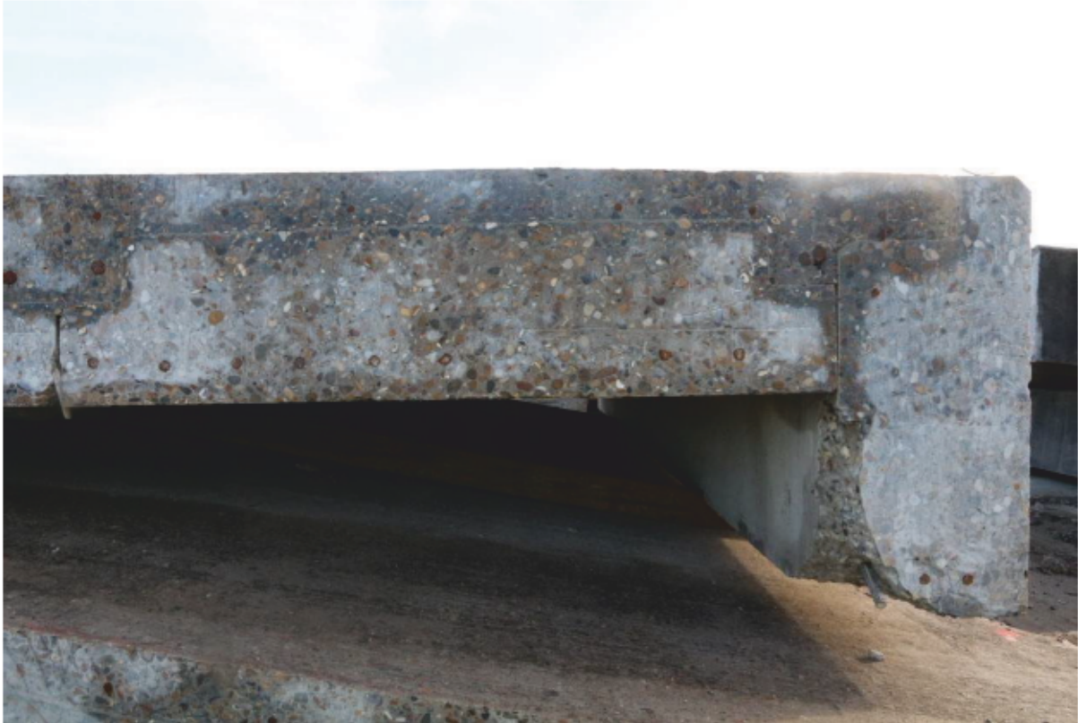
Plate 49: Detail of Dolphin 7's cap, looking east (CIY17 D2 6)
