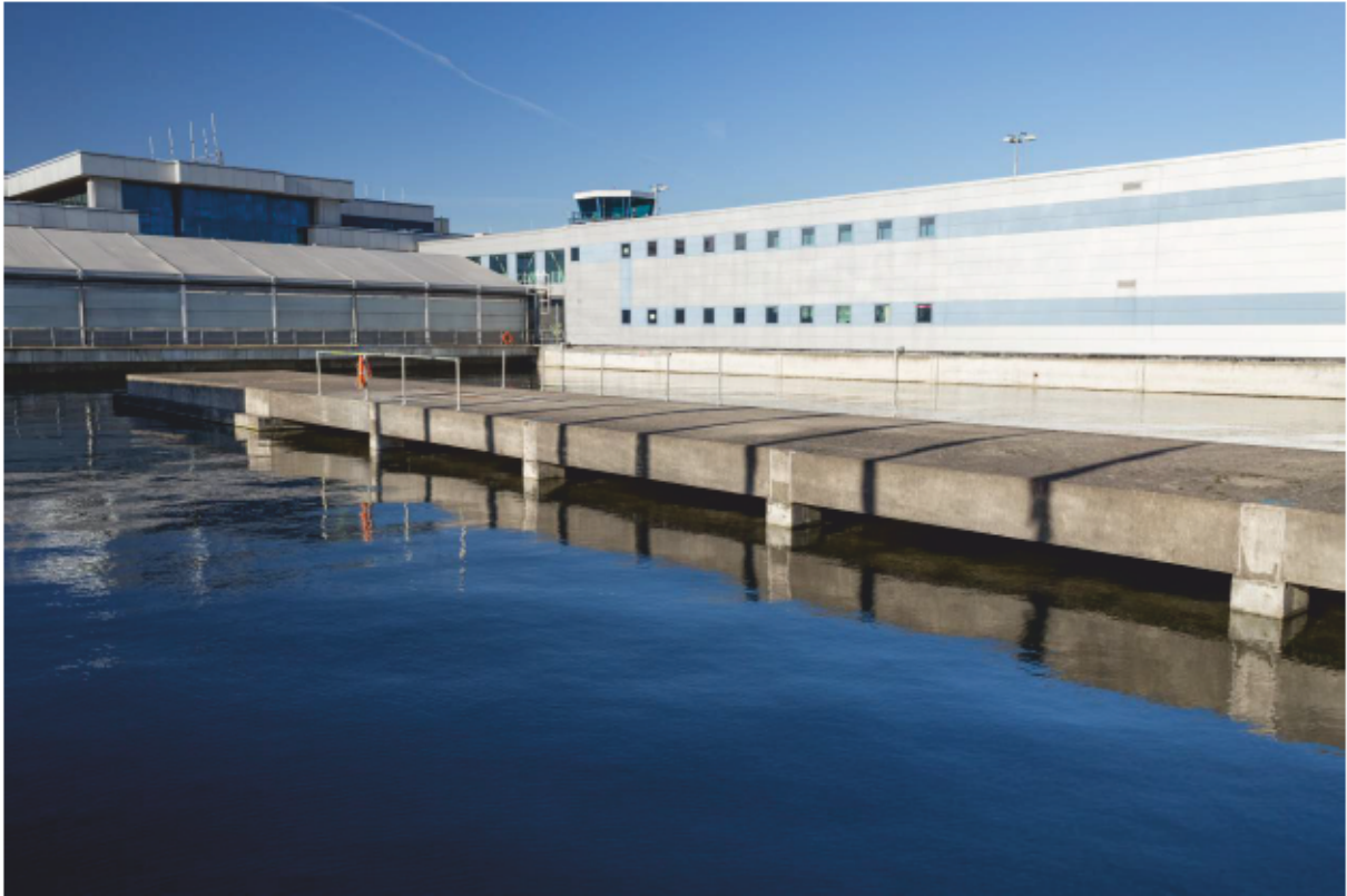
Plate 1: Dolphin 7 before removal of its cap, looking north-west (CIY17 D100 010)
