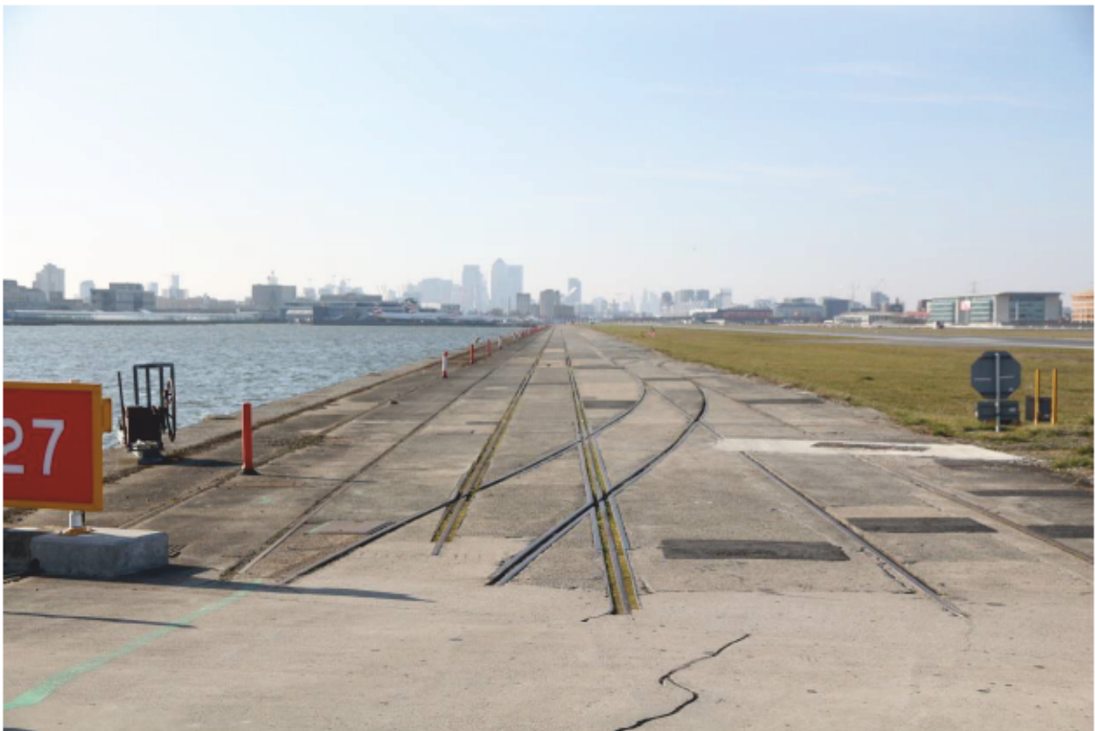
Plate 86: Railway tracks along north quayside of King George V Dock, looking west
