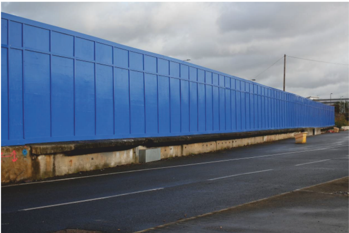
Plate 34: Platform edge on the south side of former Transit Shed 1 at the east end of the south side of King George V Dock, looking north-east (CIY17 D1 3)
