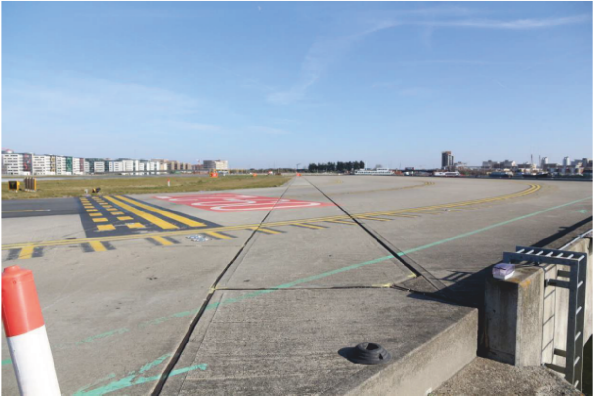
Plate 73: Runway extension into King George V Dock, looking east
