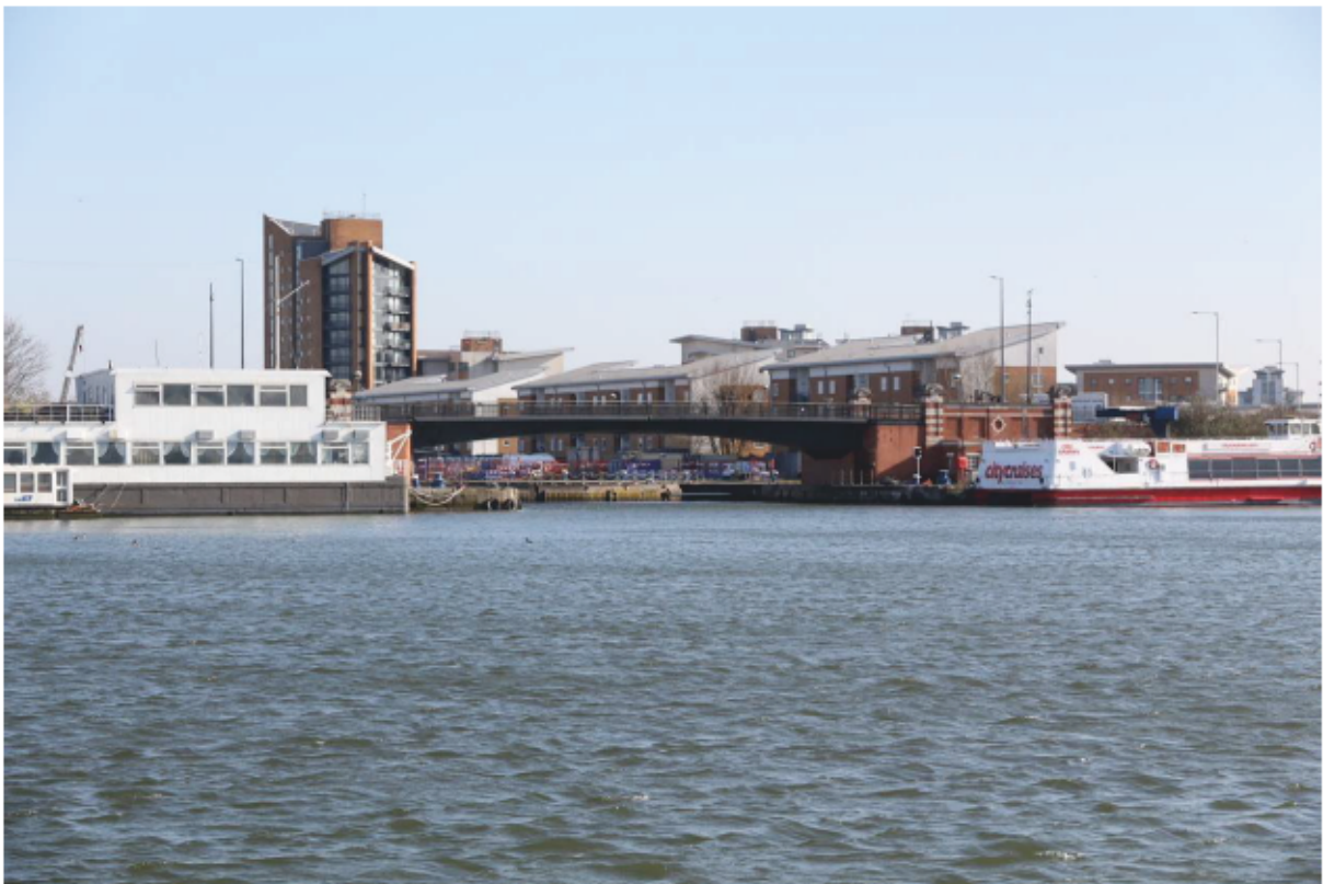
Plate 92: View of the former Bascule Bridge from the north quayside of King George V Dock, looking east
