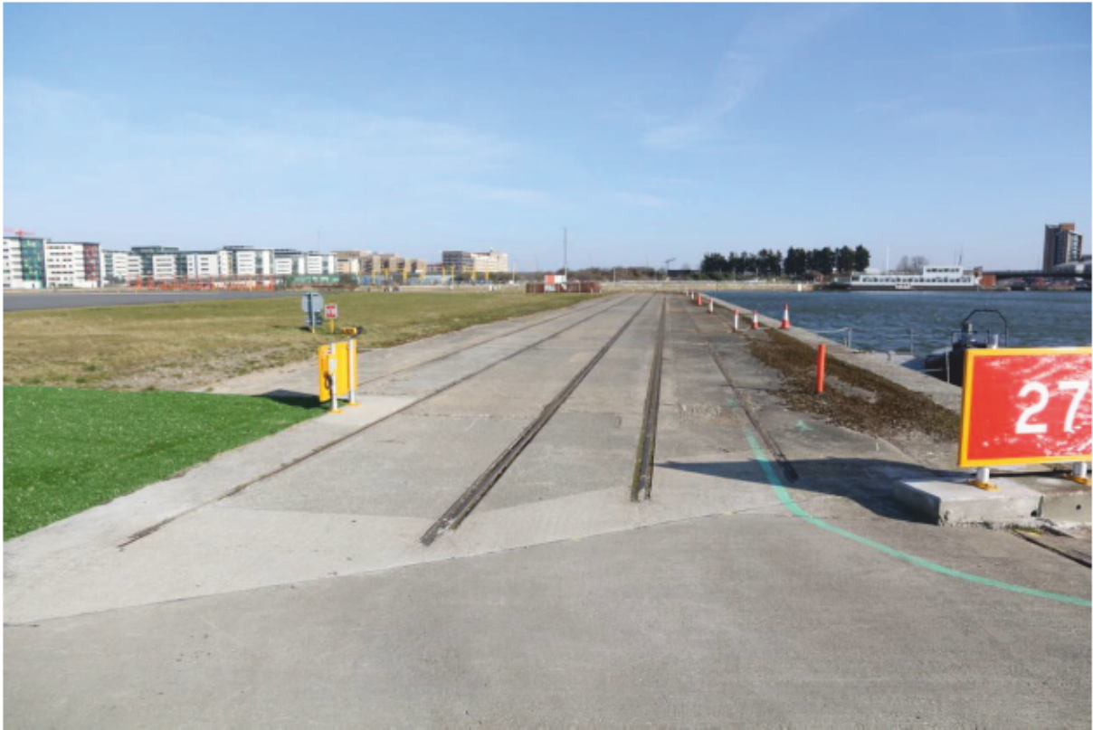
Plate 87: Railway tracks along north quayside of King George V Dock, looking east
