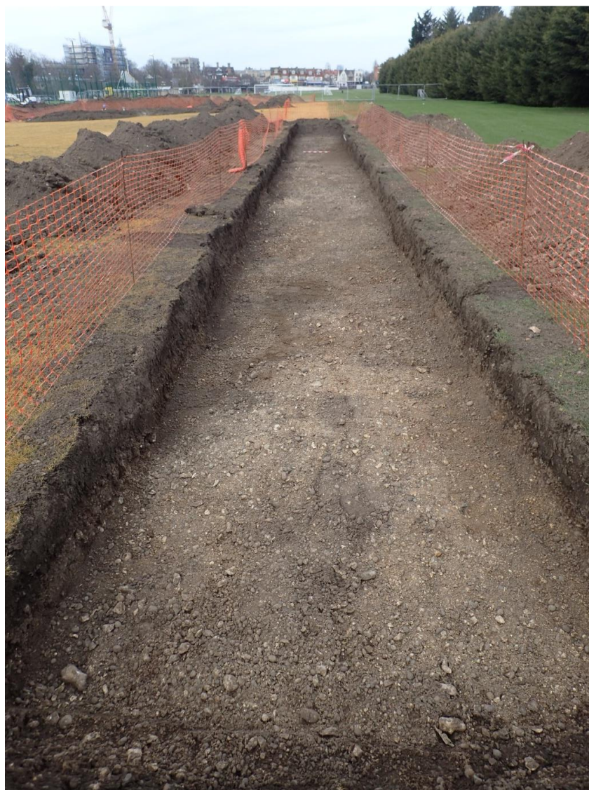
Plate 2. Trench 2, looking north. Natural gravels [4]
