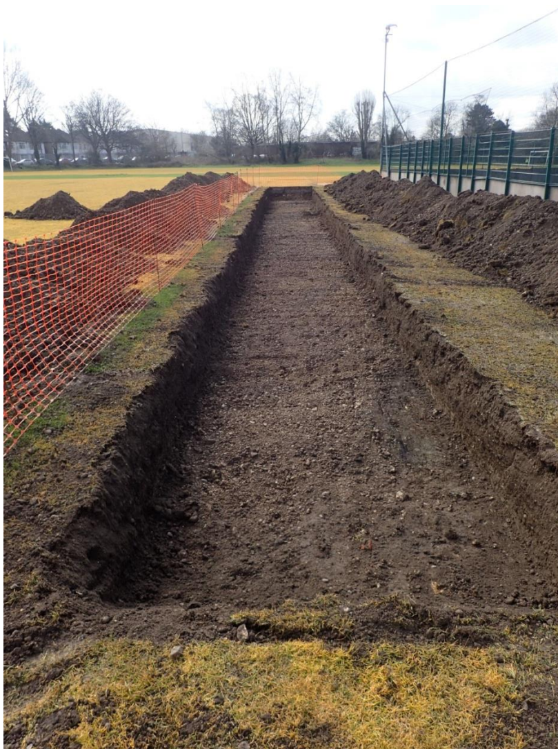
Plate 1. Trench 1, looking south. Natural gravels [2]
