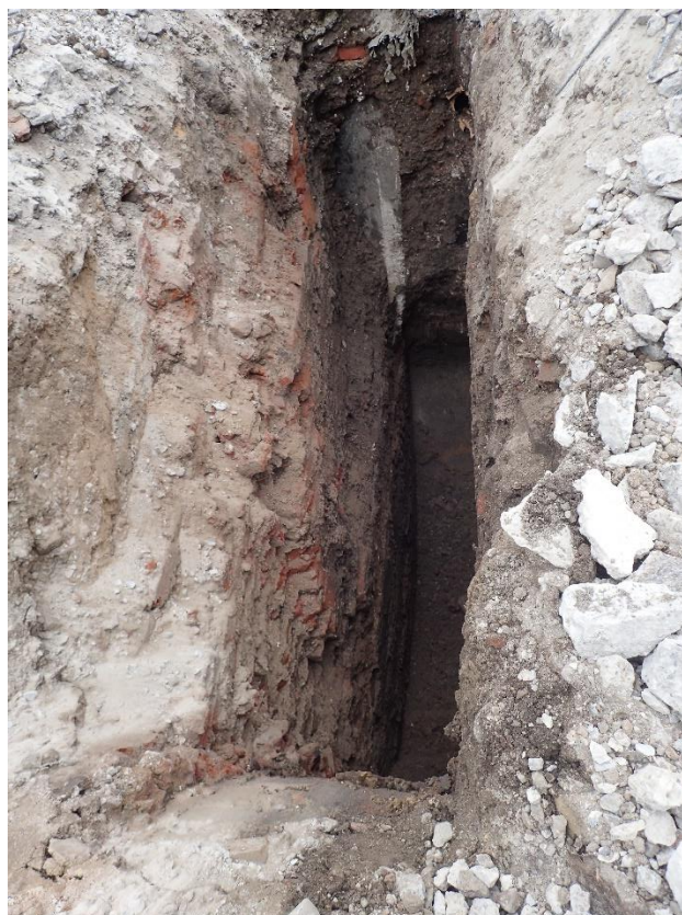
Plate 2: WSTP 2 with wall [100]. Looking north.
