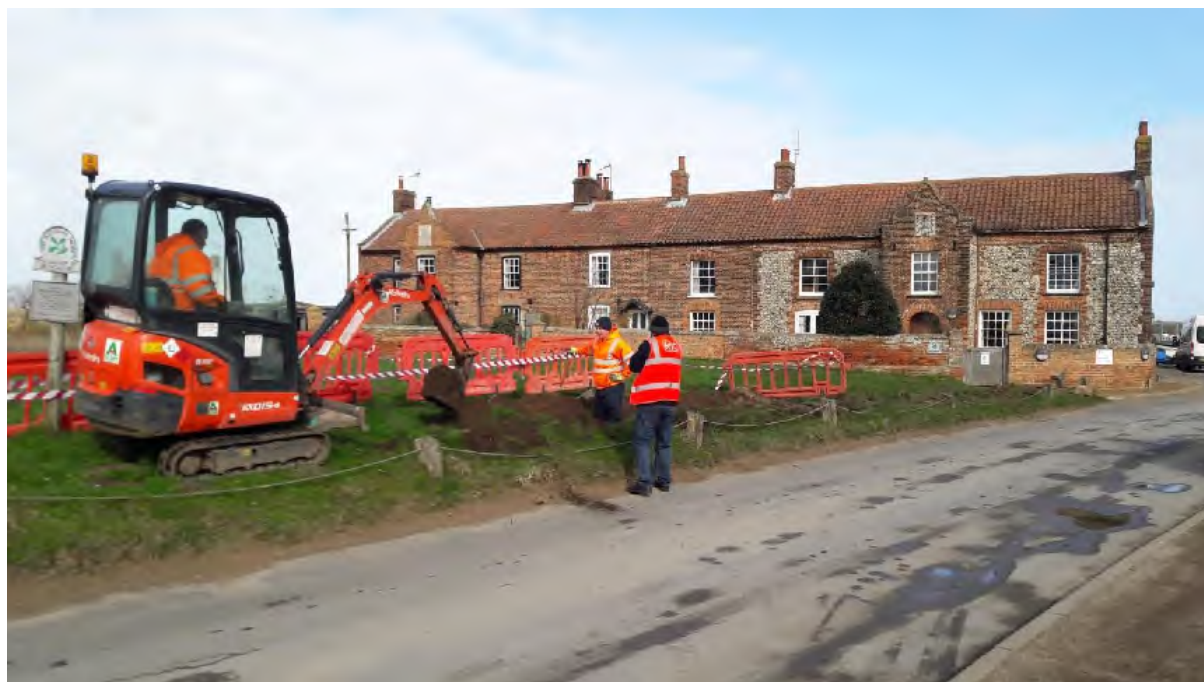
Plate 3 Machining the cable-trench, south of the Activity Centre, looking north-west
