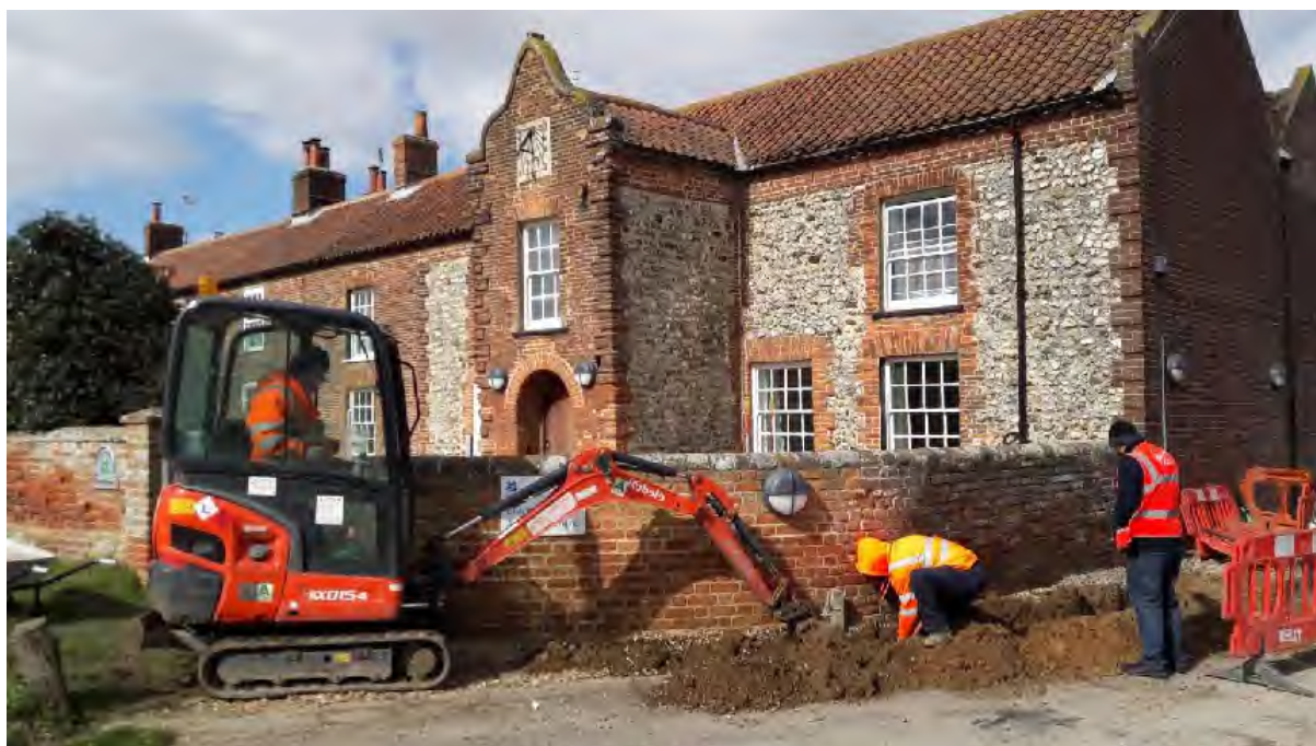
Plate 1 Machining cable-trench adjacent to Activity Centre, looking north-west.
