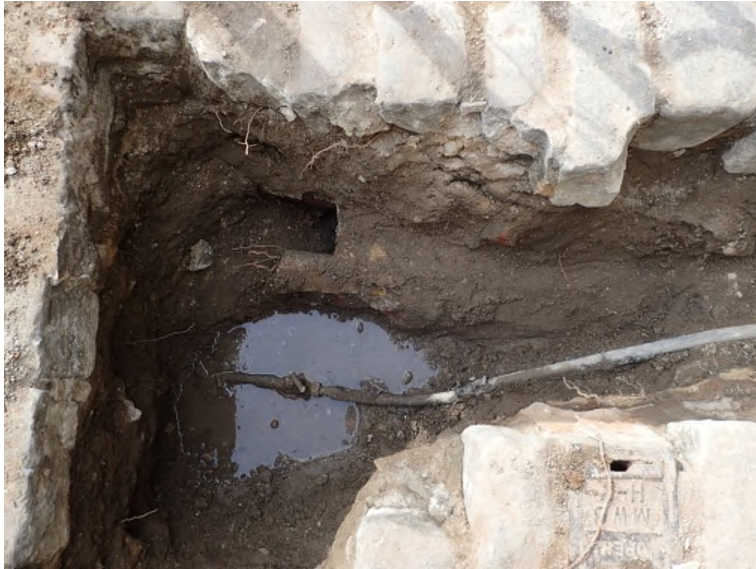
Plate 2: Brick drain [6003]. Looking South.
