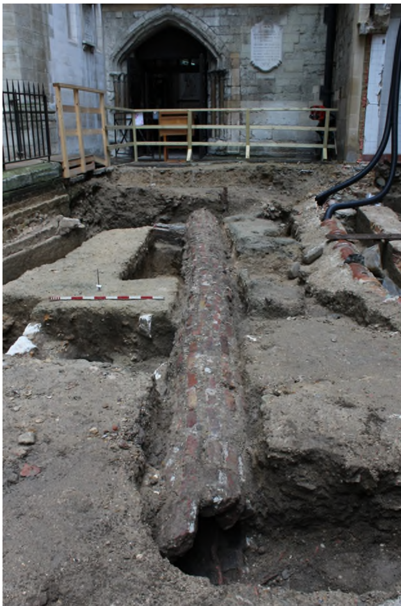
Plate 10: West facing view of culvert [97] (1m scale)
