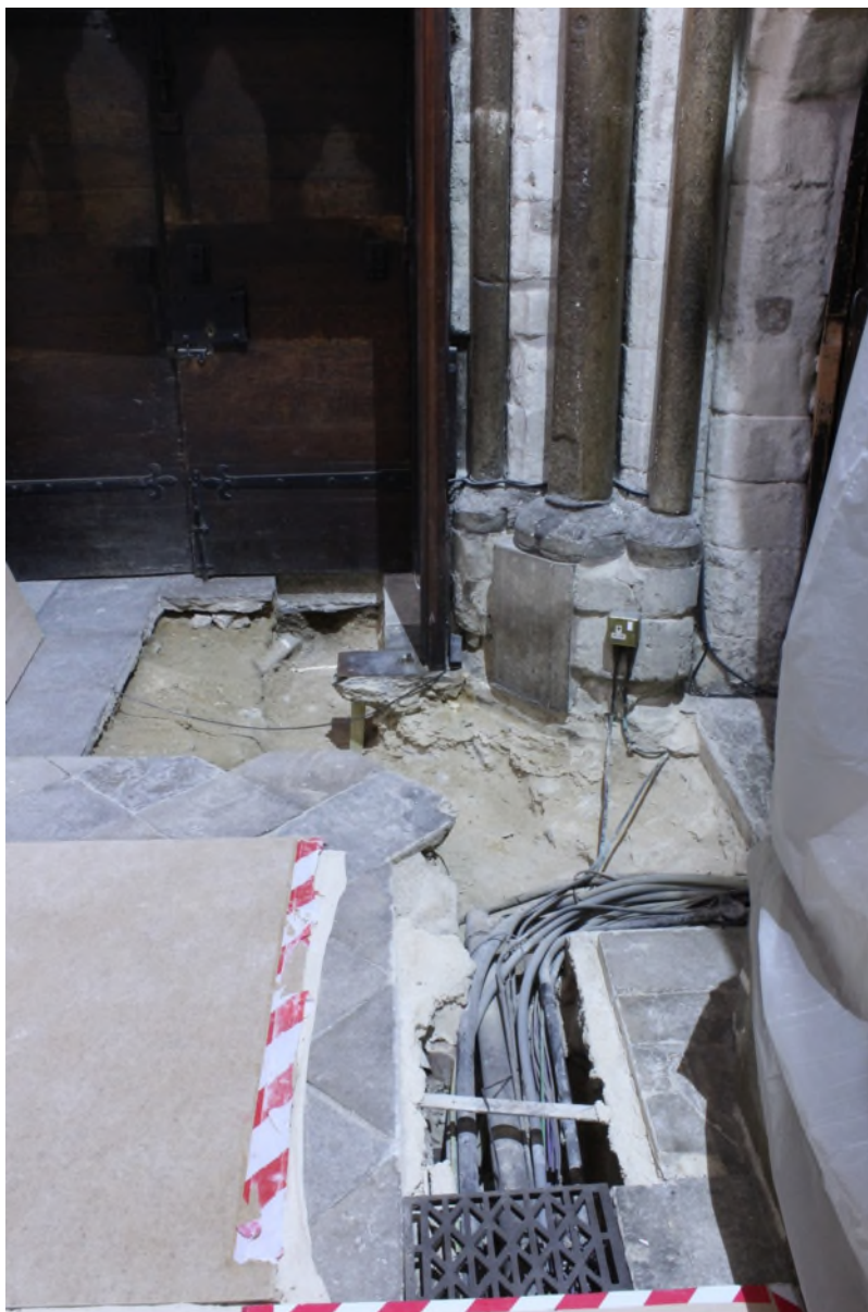
Plate 6: East facing view of South Transept Heating Duct
