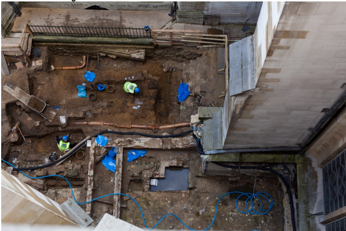
Plate 1: South facing view of Main Excavation Area
