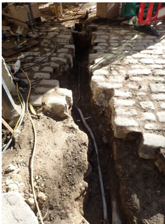
Plate 1: Trench 300 as excavated. Looking East.
