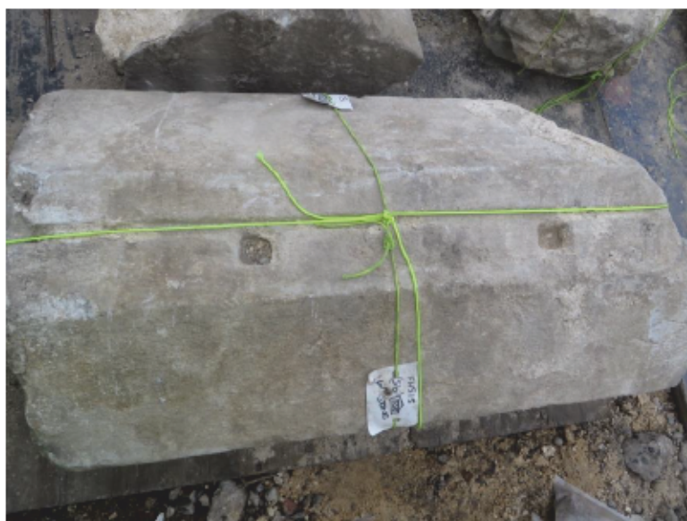
Figure 1: Simple Chamfered Mullion Profile
