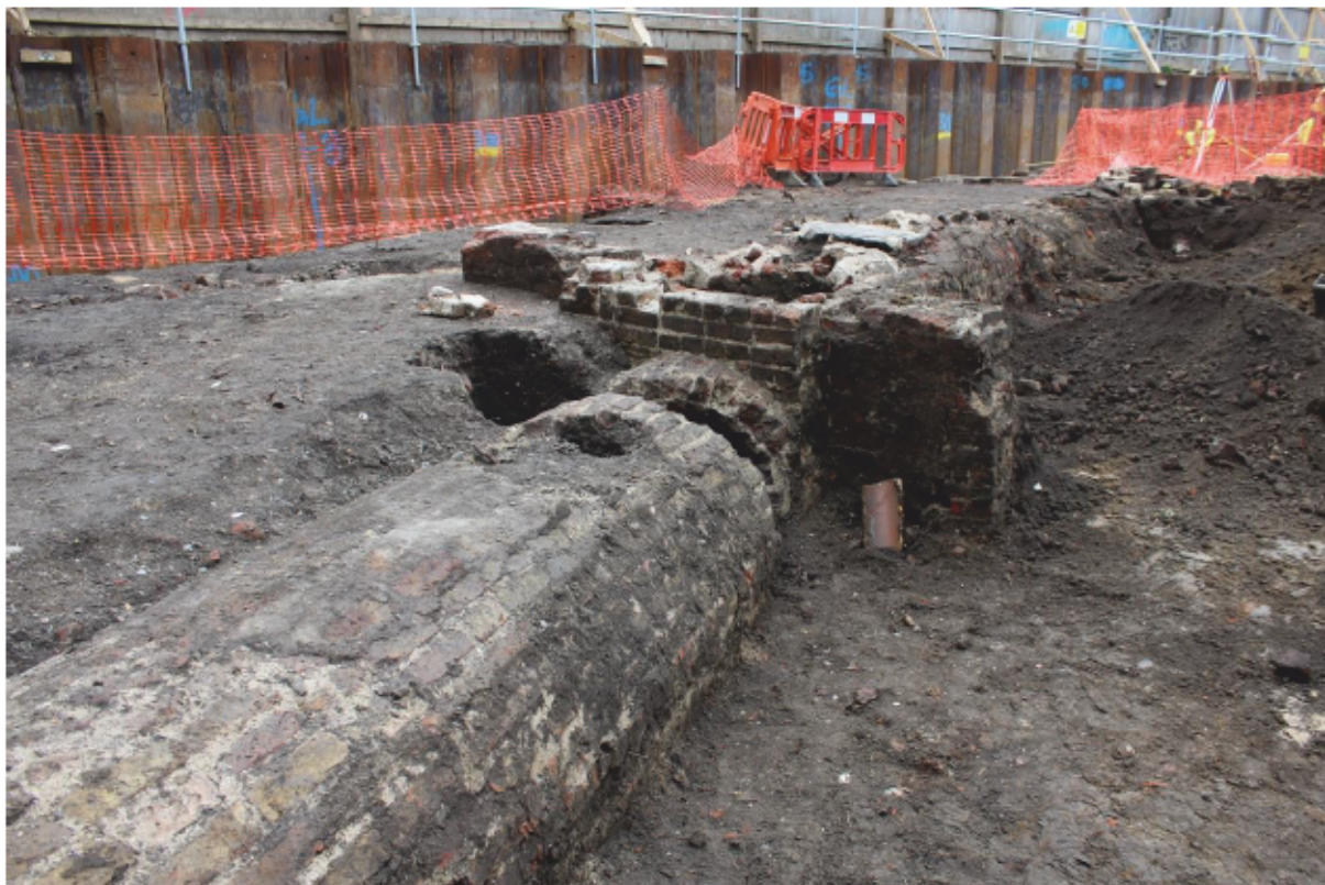
Plate 11: Brick culvert [66], manhole [75] and later connecting sewer [74], looking south-east.
