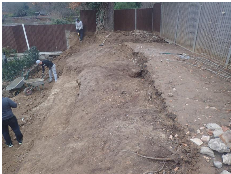
Plate 10: view north of bank during removal of modern dumped material [6]
