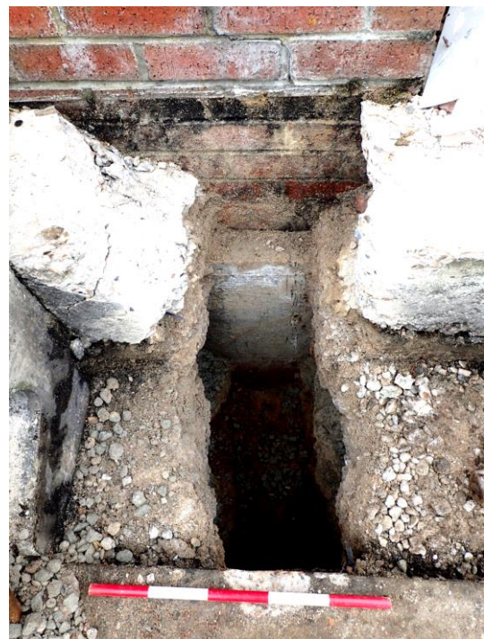
Plate 1a: General view of Test Pit 3 (left) located against the north-west corner of the Canning Flex Warehouse building. View to the south-east. Plate 1b: View of Test Pit 3 (right) to south-east showing concrete foundations. Scale 0.5m.
