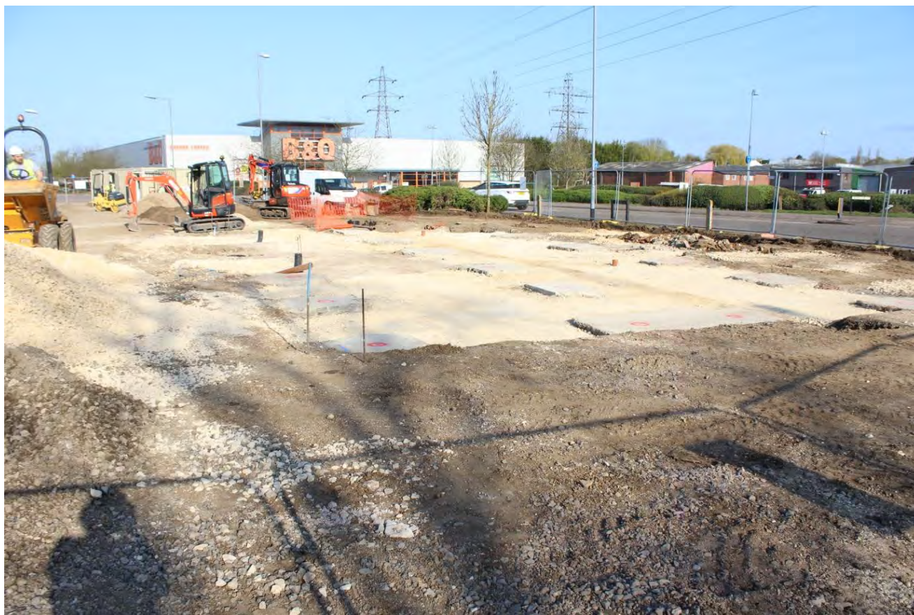
Plate 1: The site, looking north-west
