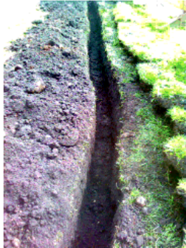
Plate 1: View to west of Cable trench
