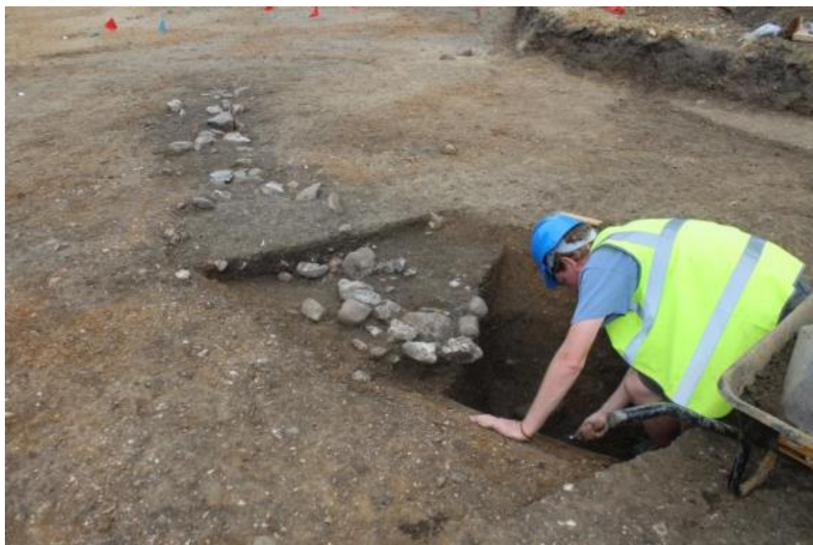
Plate 12: Potential Wall Foundation [1518], mid excavation
