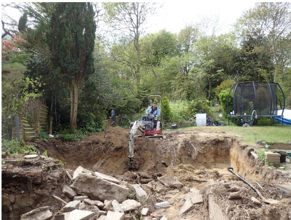
Plate 1: Watching brief area under excavation facing south-west
