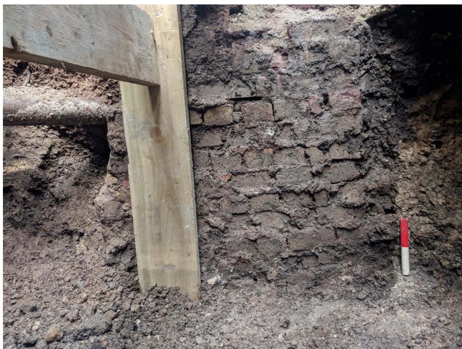
Plate 4: Manhole [25], looking north, 0.20m scale.
