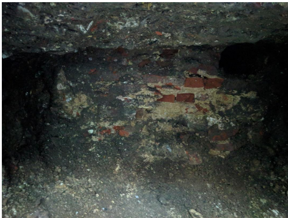
Plate 3: Post-medieval wall [18] below concrete beam, looking east.
