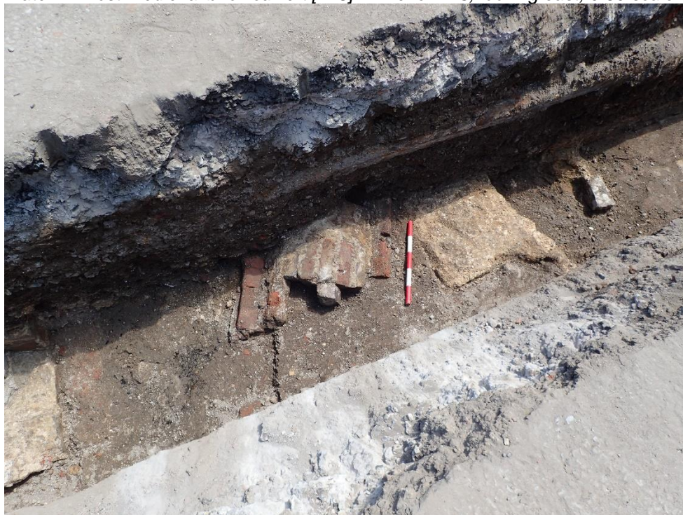
Plate 17: Post-medieval brick culvert [148] in Trench 2-3, looking east, 0.50 scale
