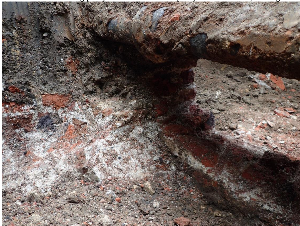
Plate 9: Vaulted ceiling [128] and basement wall [127] in Trench 3-20, looking south-east
