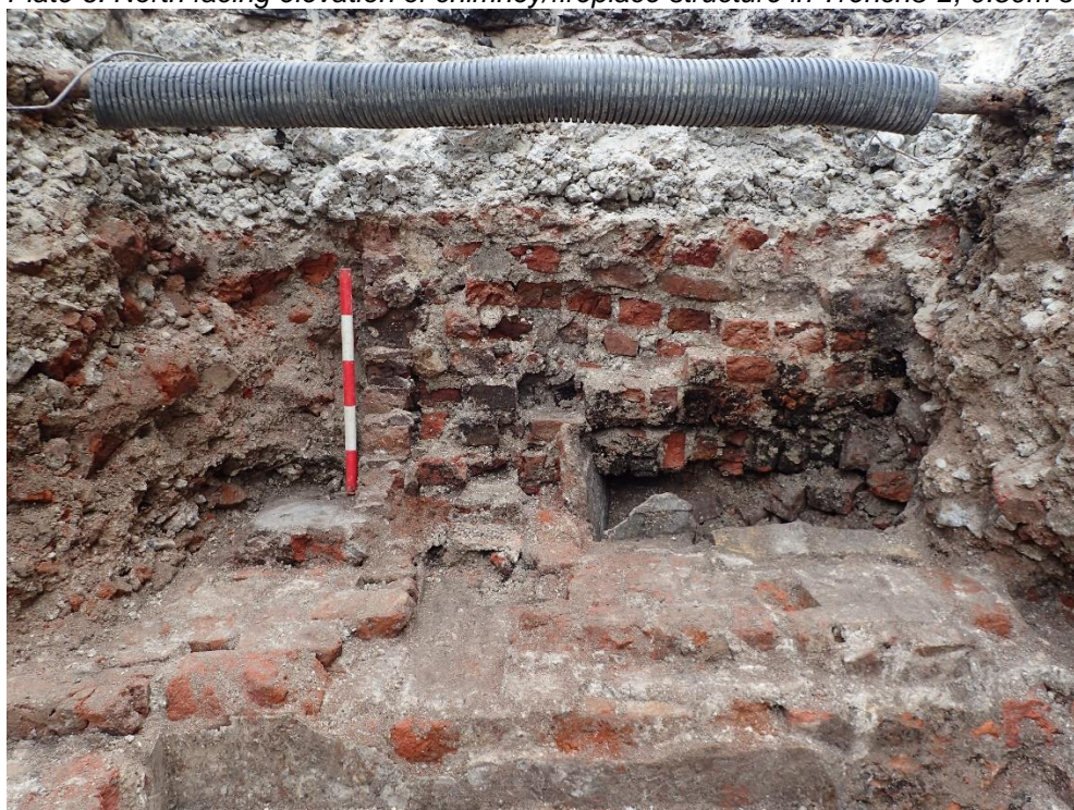
Plate 6: North facing elevation of chimney/fireplace structure in Trench3-2, 0.50m scale
