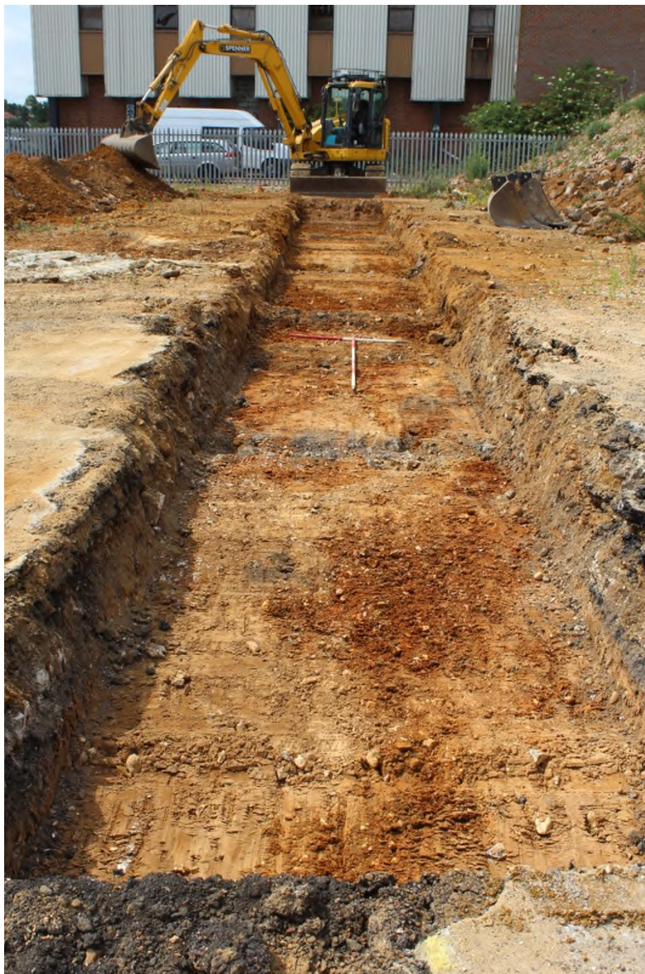
Plate 7: Trench 4, view south-west
