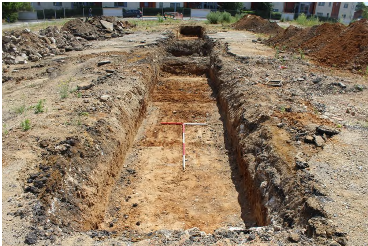
Plate 9: Trench 6, view south-east
