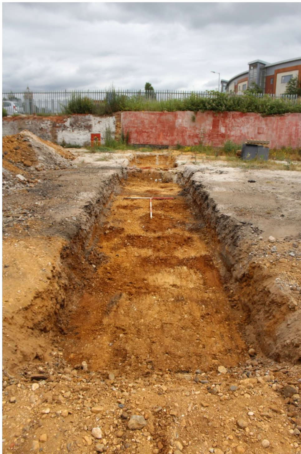
Plate 5: Trench 2, view north with backfilled Wall Foundation [43] in middle ground
