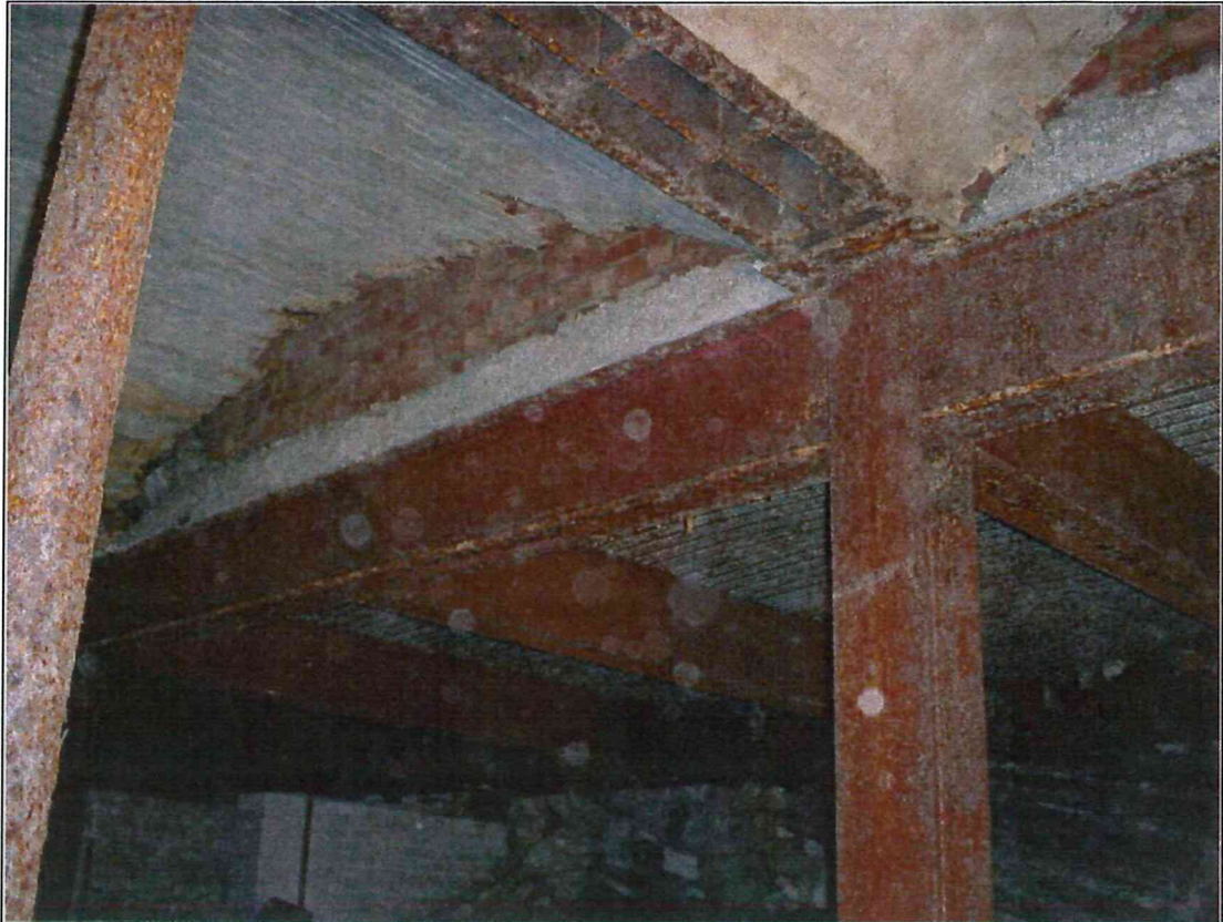
Plate 1 – Stables' Arches and Steel Girder Frame
