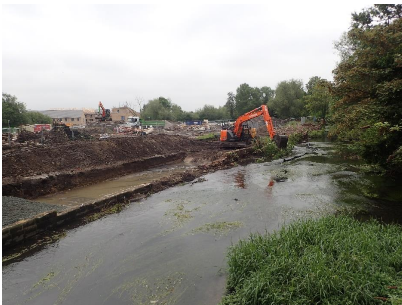
Plate 1: Site Overview, Facing South East
