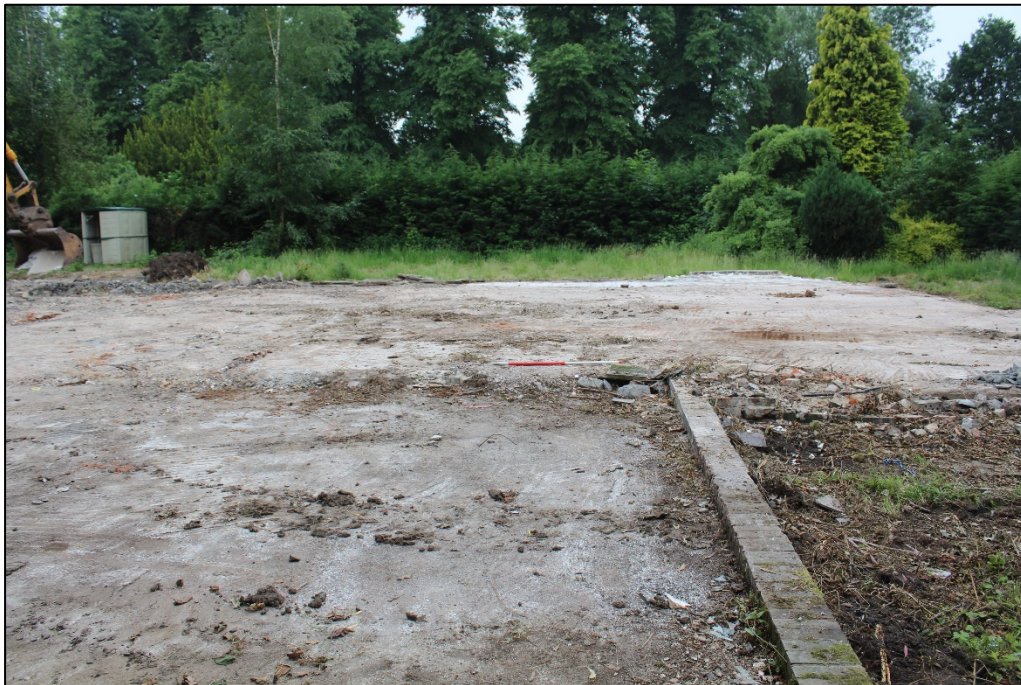
Plate 2: Pre-ex shot showing concrete paving: view west, scale 1m
