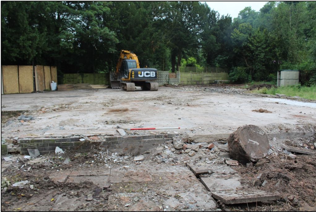
Plate 1: Pre-ex shot showing concrete paving: view south southwest, scale 1m
