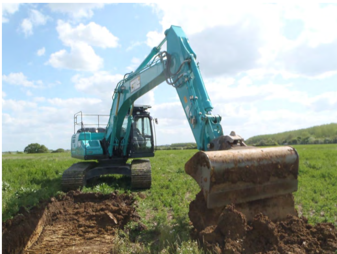
Plate 2: The site, machining, view south.
