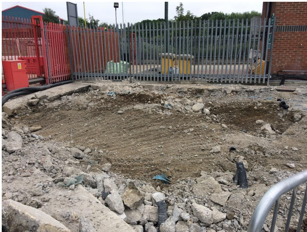
Plate 2: Post-medieval layer, looking west
