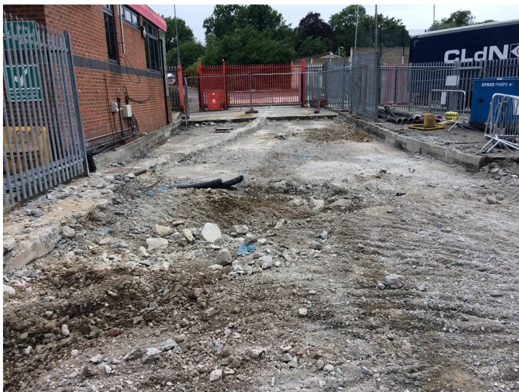
Plate 3: Existing HGV Entrance showing after removal of concrete slab, looking south
