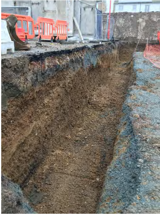
Plate 4: Banding of natural gravels along the western edge of site, looking NW
