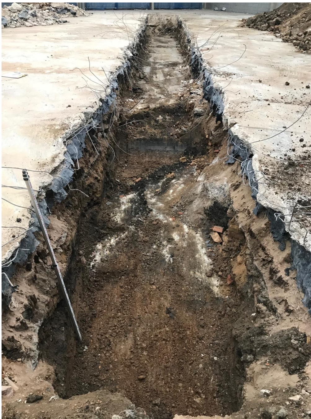
Plate 4: Trench 4 – Looking North-West
