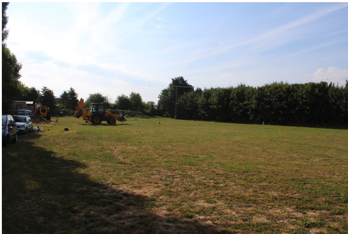
Plate 1: The site, view south-east
