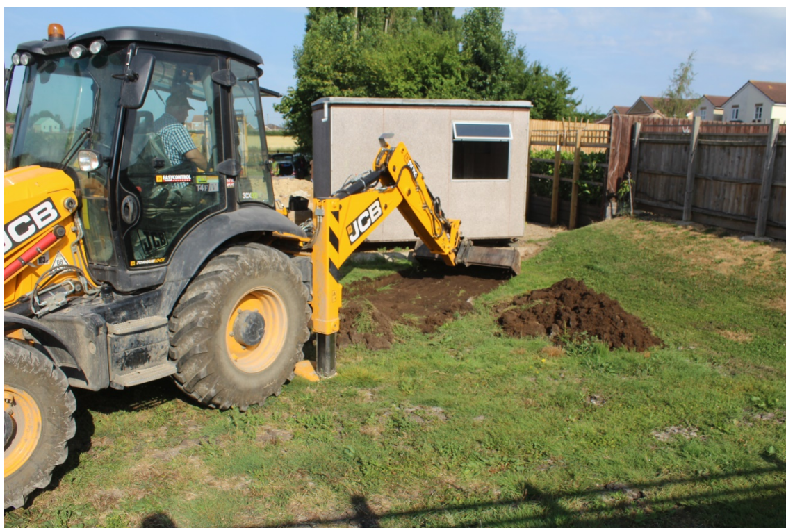
Plate 2: The site, machining, view north-west
