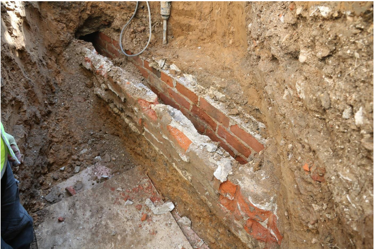
Plate 13: Brick drain [18] and [34], looking north-east
