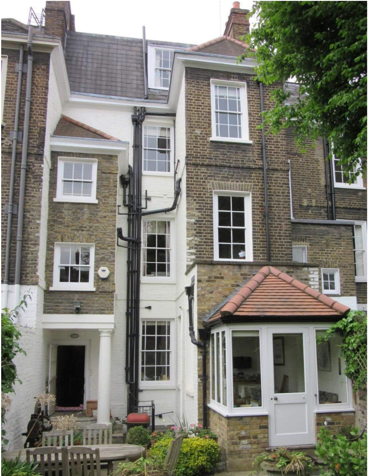
Plate 1: Rear (north-east) elevation of no. 26 Cheyne Row showing 1988 porch extension (left), three storey closet wing (right), late 19th century flat roofed closet wing extension (right) and 1988 garden lobby (right) (©Crone and Cummins, 2017, fig.10)
