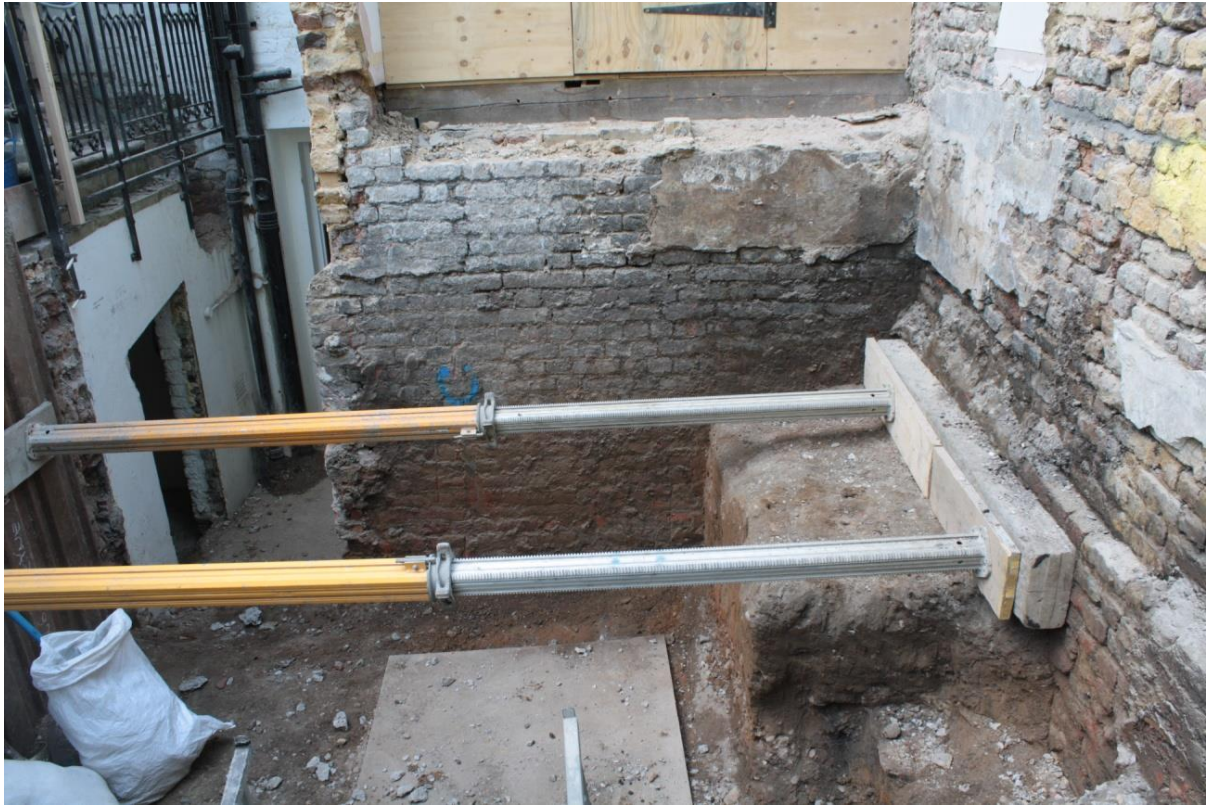
Plate 3: Excavation area showing rear (north-east) wall of closet wing [50], looking south-west
