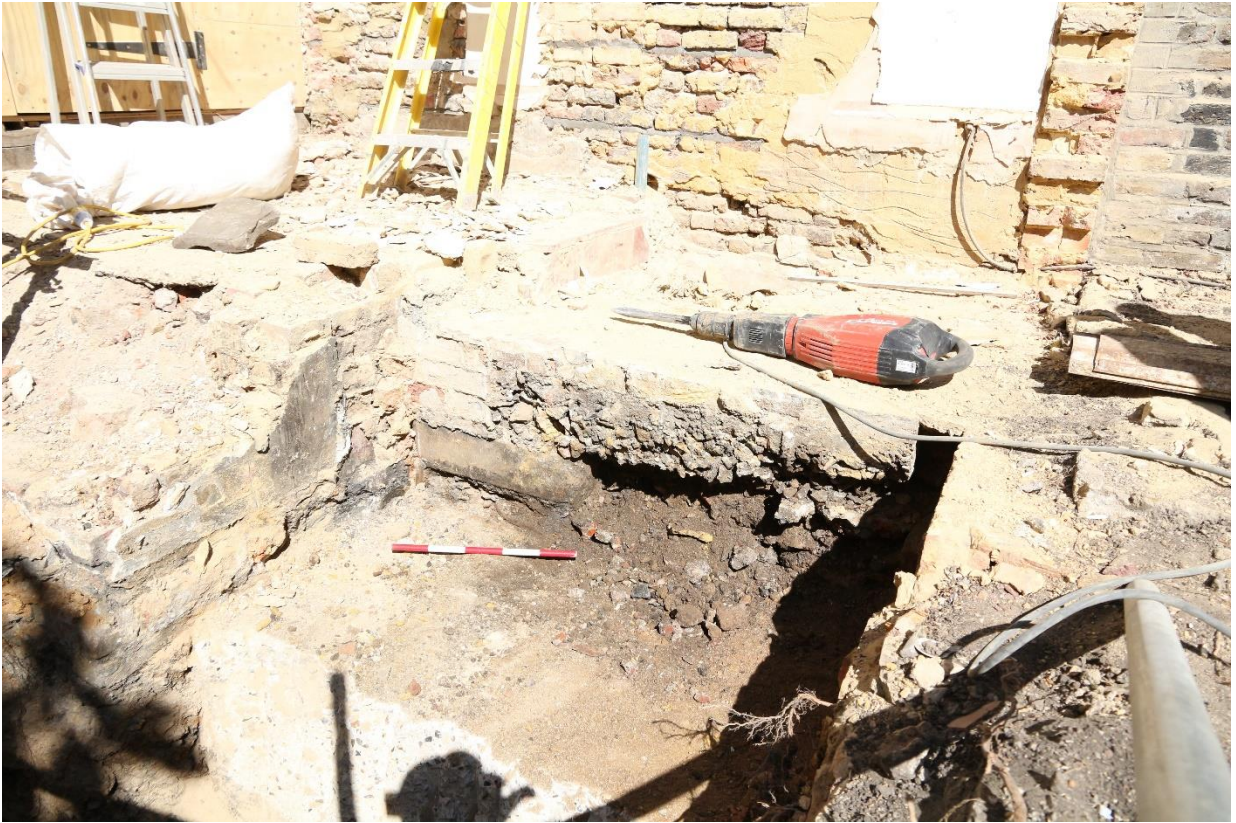
Plate 7: Remains of stone sink (just above scale) in [35], looking west
