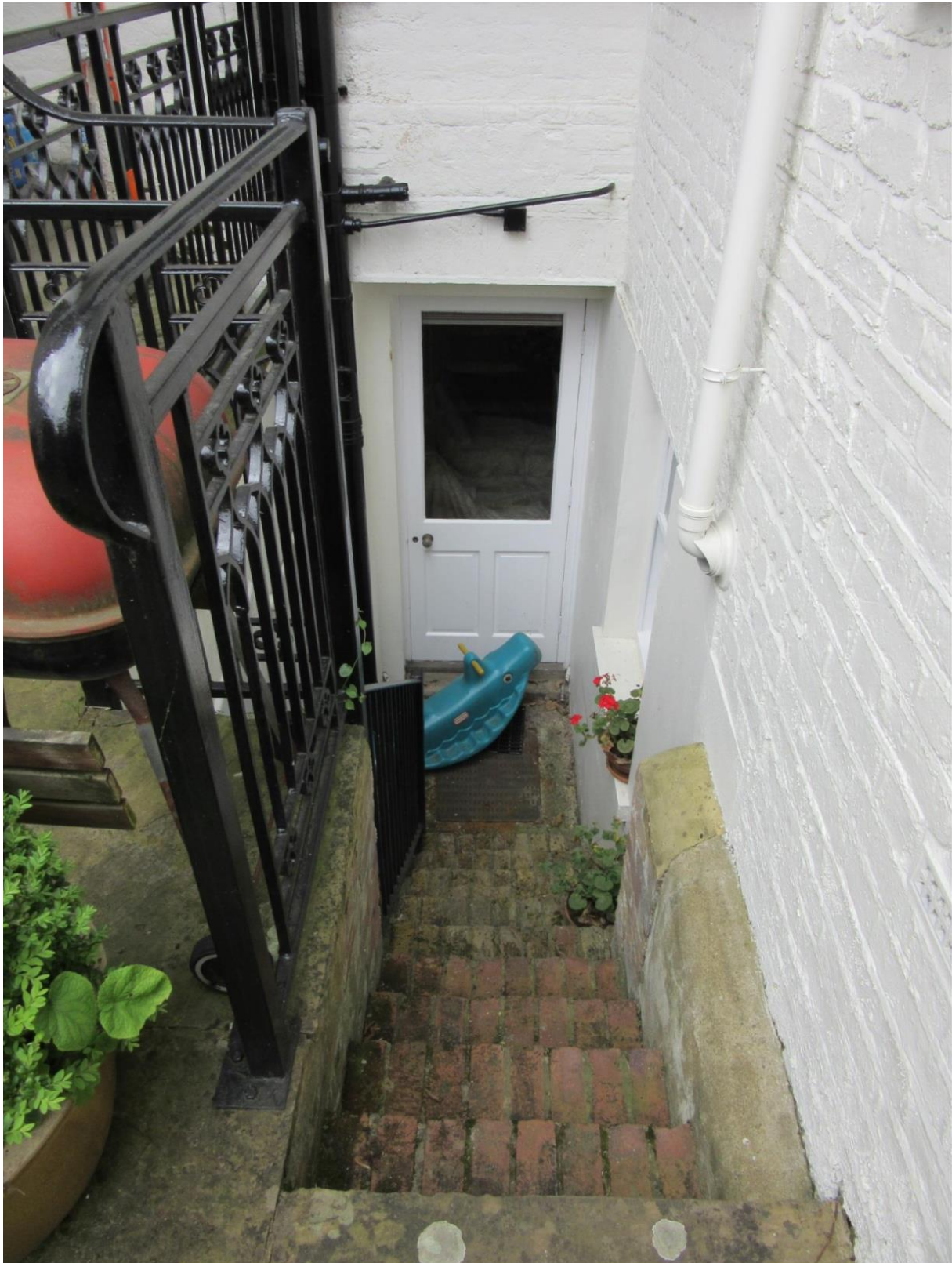
Plate 2: Rear (north-east) elevation of no. 26 Cheyne Row showing steps down to the rear lightwell and doorway into the basement with the storey closet wing and late 19th century flat roofed closet wing extension (©Crone and Cummins, 2017, fig.11)
