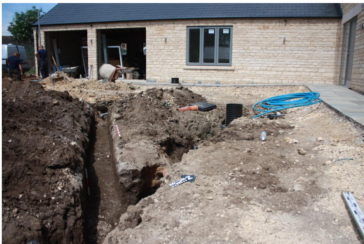
Plate 6: View looking northwest showing an excavated service trench.
