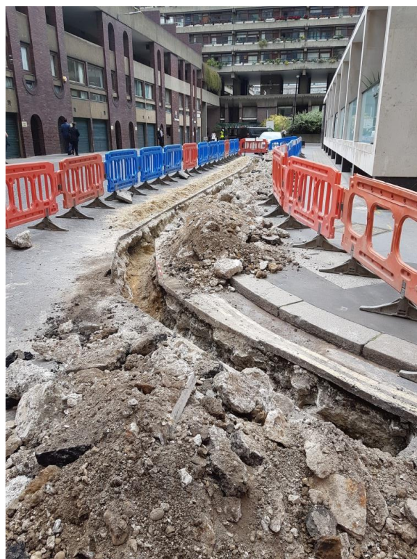
Plates 2: View of Trench
