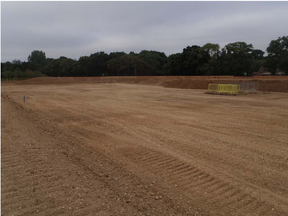
Plate 2 – General view south, topsoil stripped for new car park.
