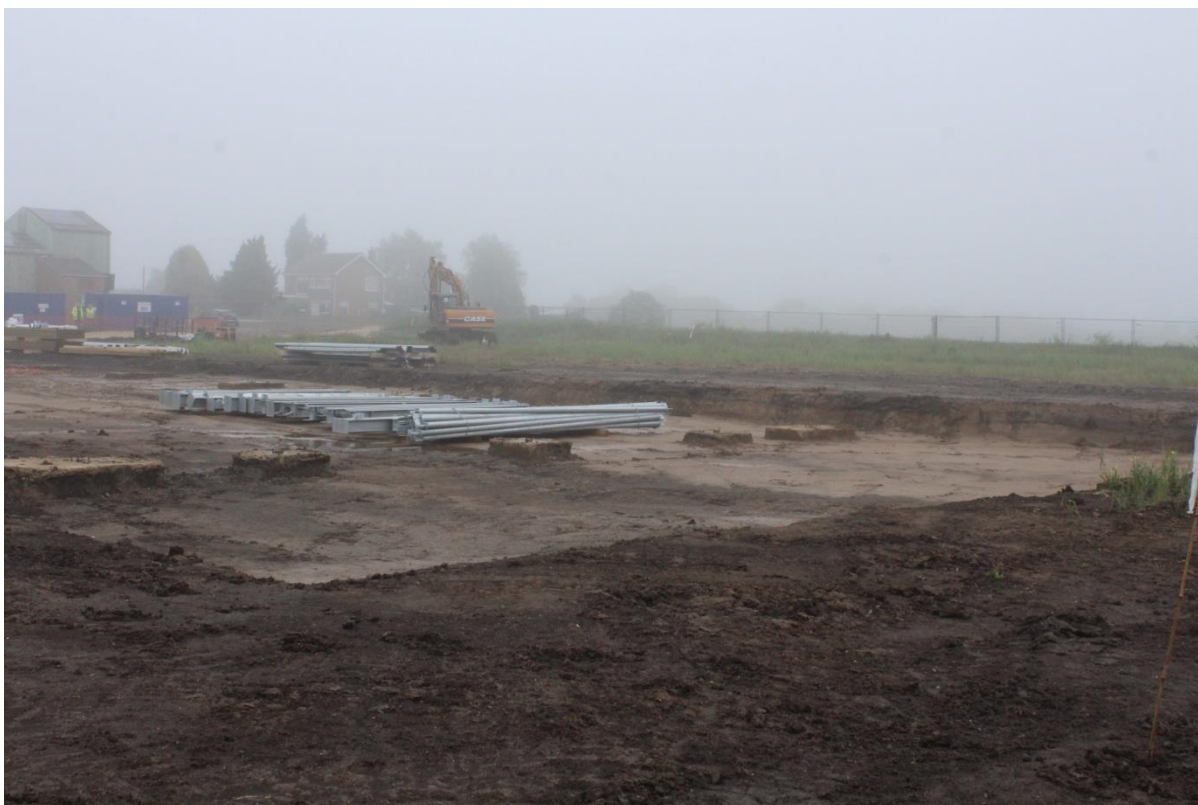
Plate 1: View of the site, looking north.
