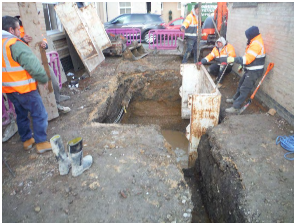
Plate 16: Excavation of the Pumping Station
