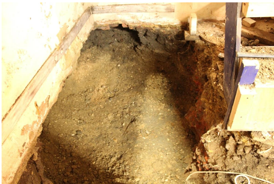
Plate 3: Trench 3, looking NE.
