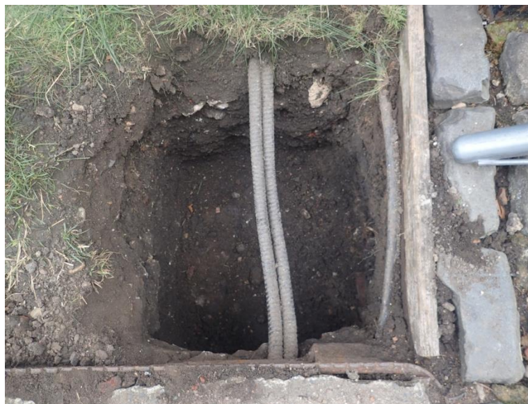
Plate 5: Test Pit 5, Looking west.
