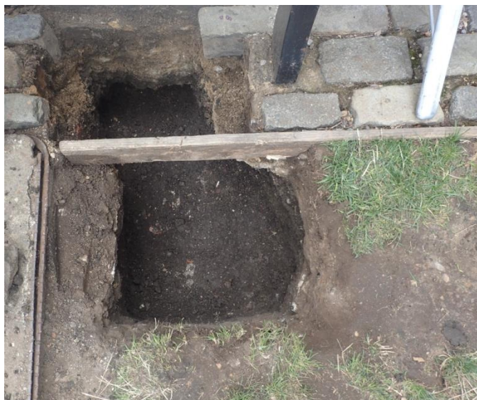
Plate 2: Test Pit 3, looking north.
