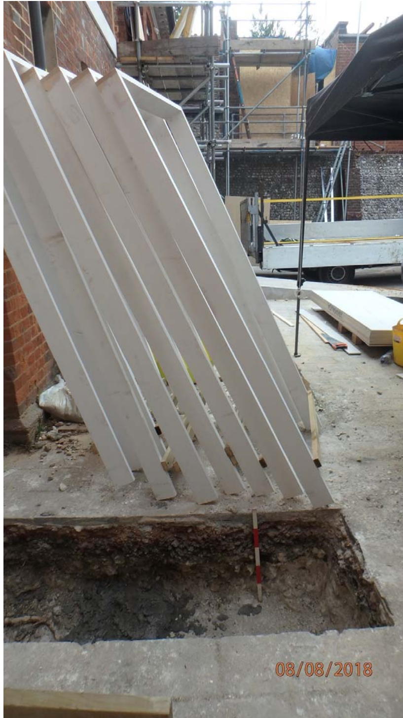
Plate 2: Stairwell pad foundation pit, view to east. Scale: 0.5m.
