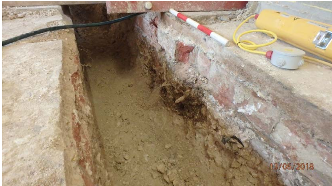
Plate 1: Service trench, inside 45 Romsey Road. Scale: 0.5m.
