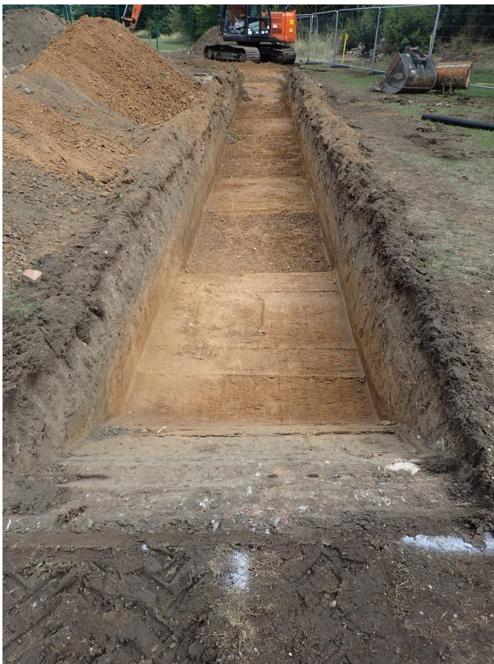
Plate 4: North facing view of Trench 5.
